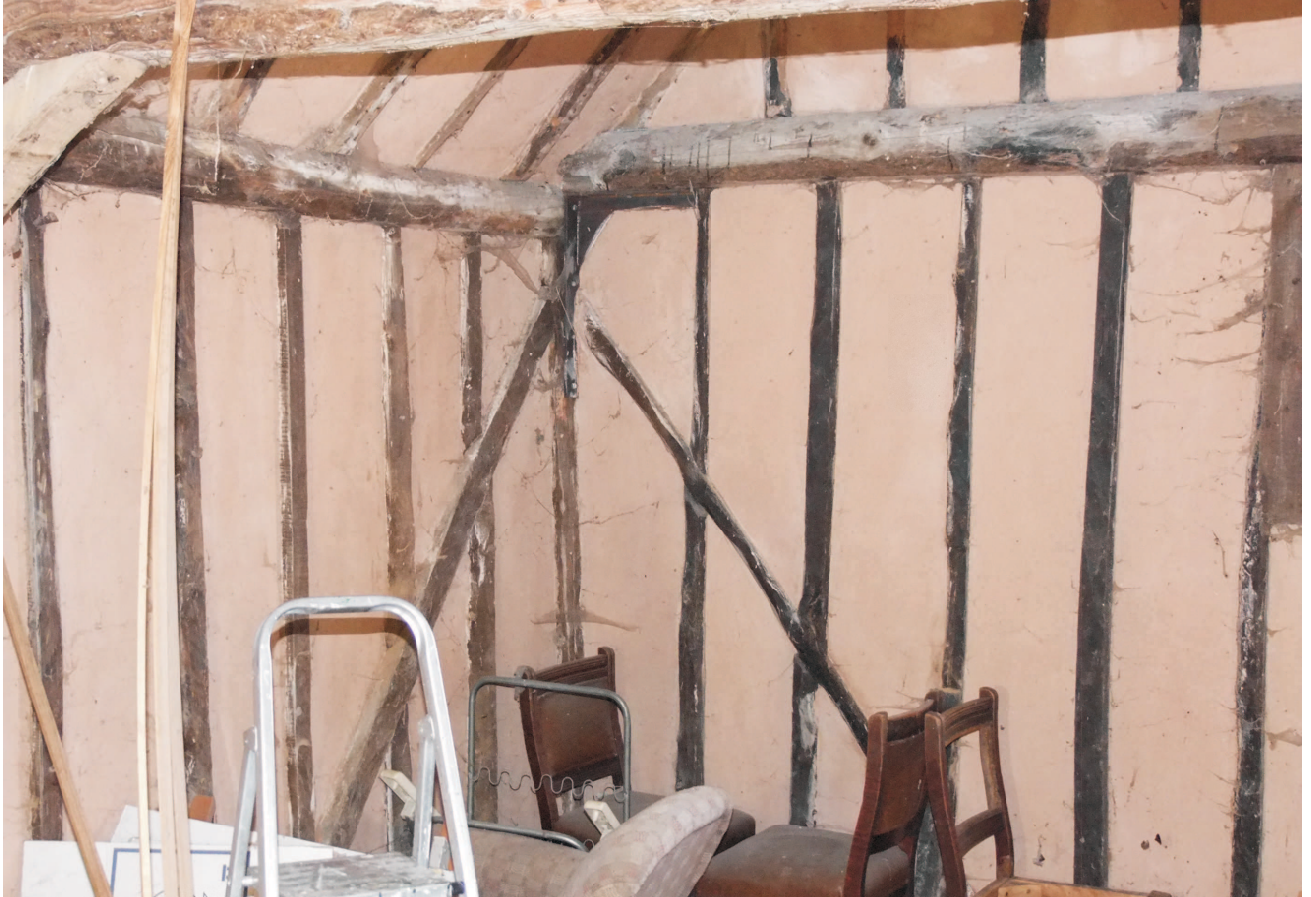
Granary view to south west corner showing wallplate and tiebeam joint with iron bracket. Primary bracing to walls
