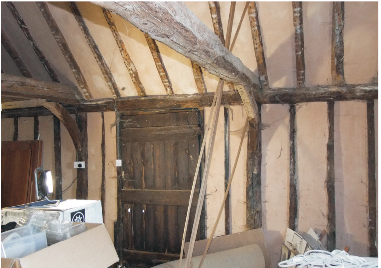
Granary view to south entrance wall. Board door in central bay. Oak arch braces between tiebeam and post.
