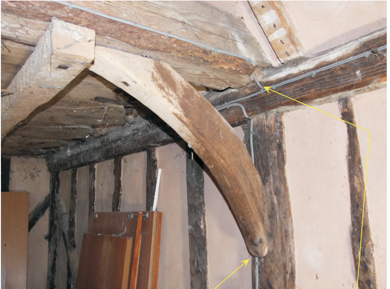
Granary south east wall showing post, plate, tiebeam & brace joint with joist for inserted floor under tiebeam.
