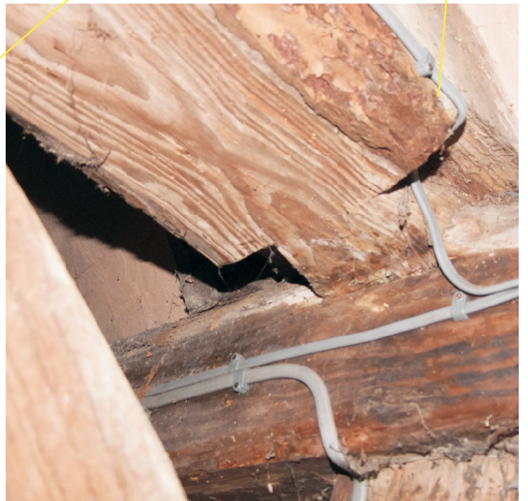
Detail of dovetail to tiebeam - wallplate joint.
