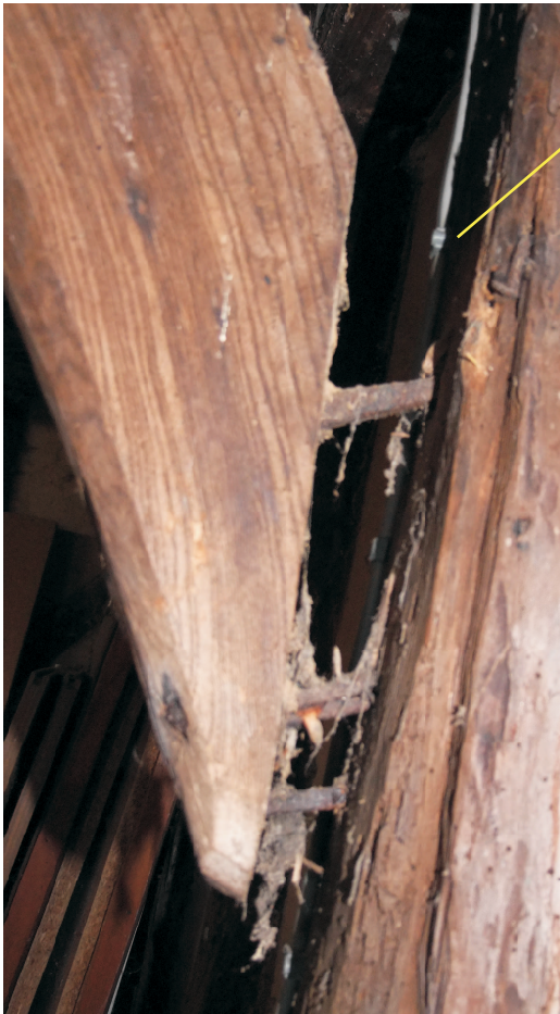
Granary south east wall showing post, plate, tiebeam & brace joint with joist for inserted floor under tiebeam.
