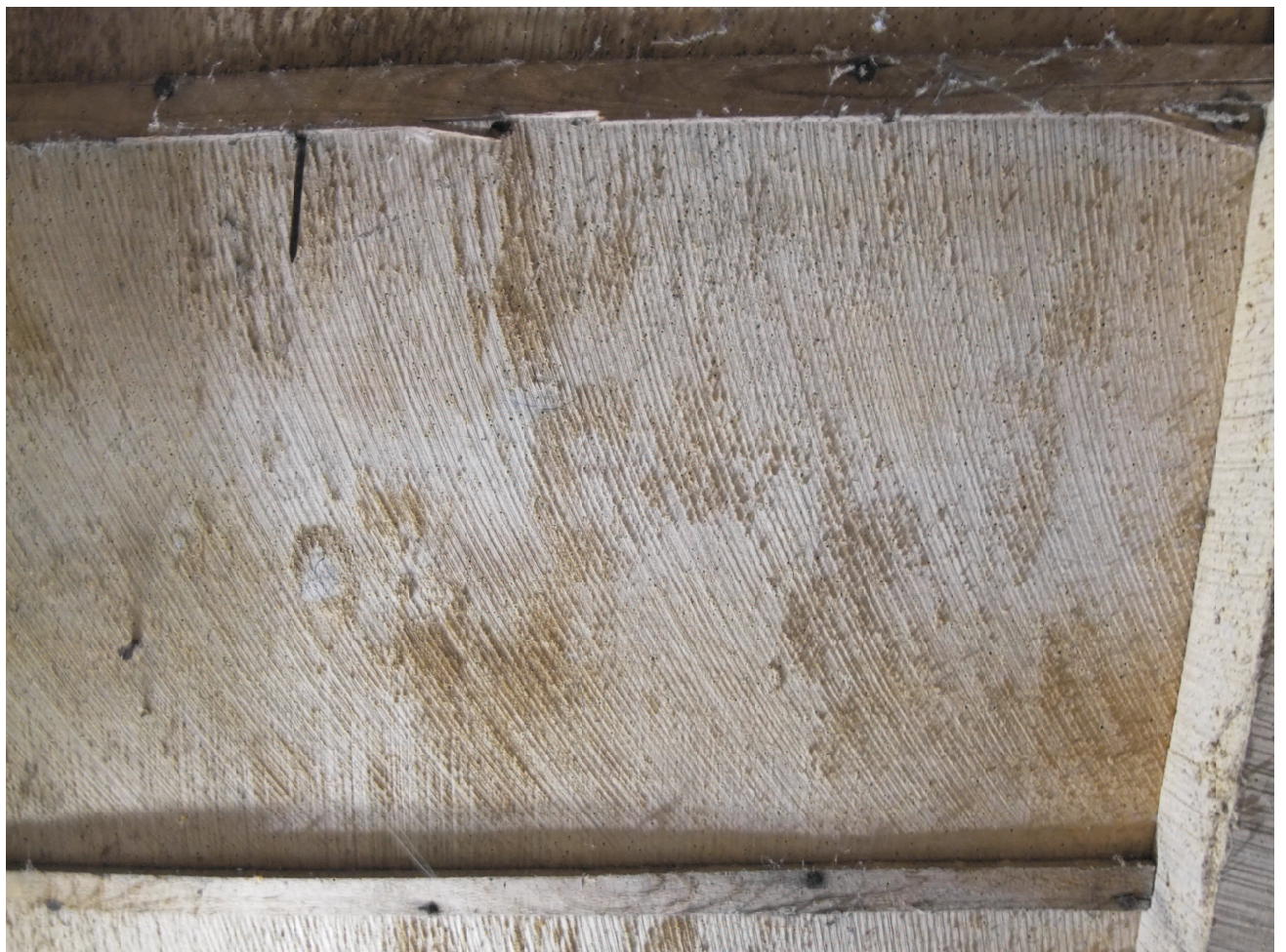
Detail of floor boards cut with very large diameter early circular saw.
