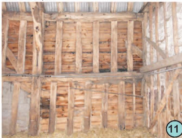
Typical section of walling to the barn with reused timbers and some bits of bracing surviving not in original positions from original use. This section to south east shows added division to south and end of late lean-to added to midstrey.
