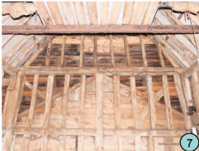
View inside east barn looking north. Roof form of attached stable shows below tiebeam and cut in entrance door at lower right hand side. Roof above tiebeam modified to a gable end when stable built.
