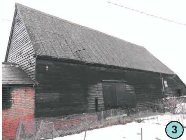
View of west side of East Barn looking south with Stable/Loose box at the north. Stable extension to south of barn with a window added to last bay of barn when converted to stabling.
