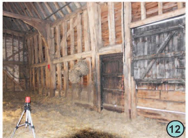
View along west wall of barn showing walling to south and doors opposite the midstrey. Small door original but large doors are into a lower opening than the reused framing originally had and this barn as rebuilt. Possibly changed to lower opening in second half of C19 when yard to west was completed.
