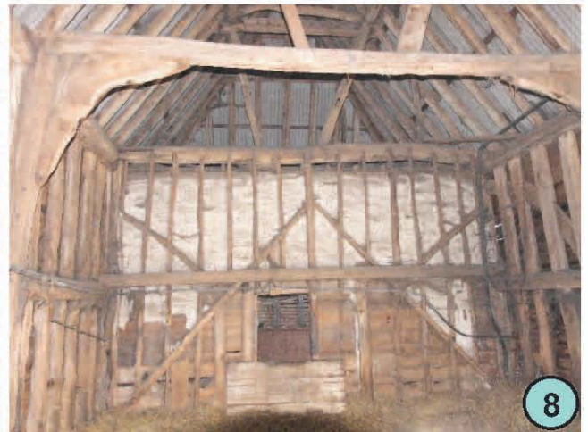
View inside east barn looking south. Shows inserted late nineteenth century partition when southern bay converted to stable when the southern extension to the barn was added.
