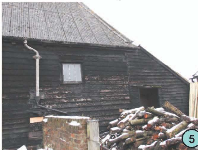
Southern end of East Barn with lean-to stable extension added when southern bay of barn also converted to stabling. Window is an addition from that time to light the stable bay.
