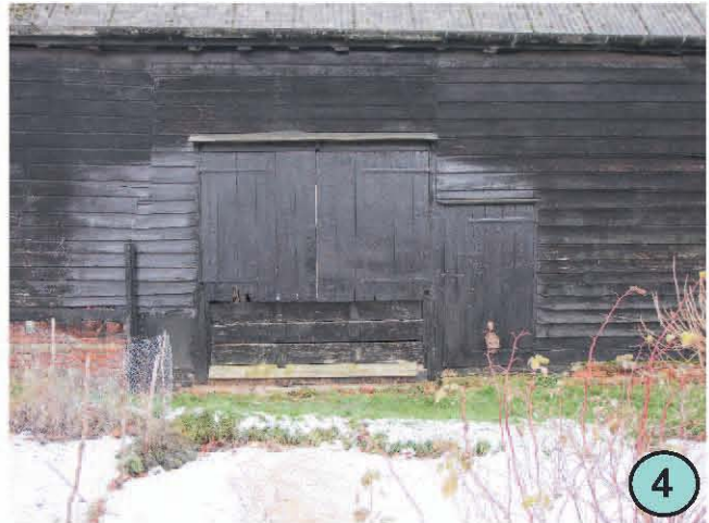
West lower doors to east barn possibly from C19. Leap boards in position below doors. Small door fully framed into barn structure. Brick plinth height varies around barn.
