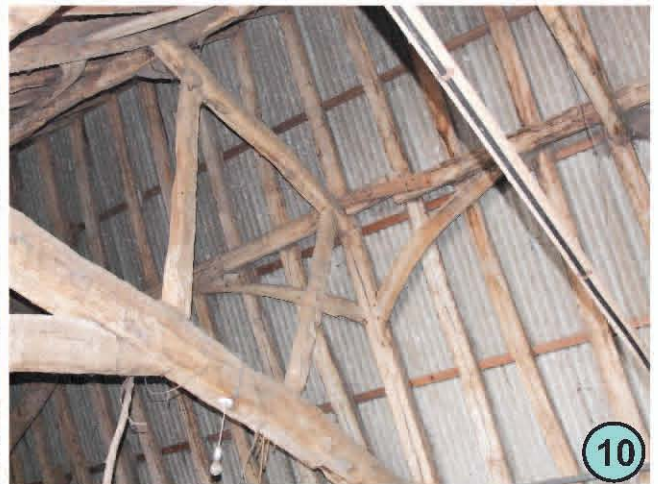
View up to roof showing wind braces, queen struts and collar on reused tiebeam with partial arch bracing. Purlin with simple half lap joints has failed. Wind braces only fitted to either side of midstrey.
