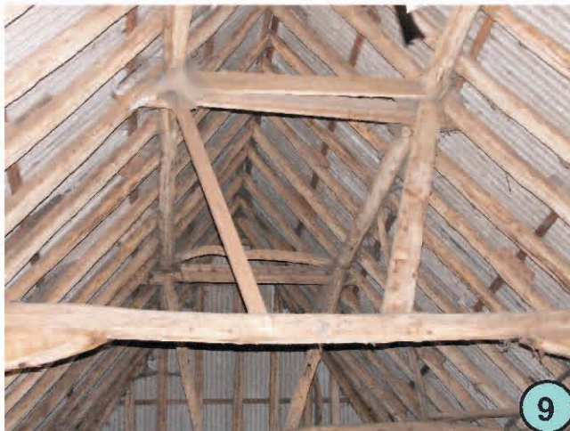
Typical view of roof construction, here looking south to original hipped end. Queen strut roof using many reused timbers and later strengthening. Reused tiebeam shows original brace mortises and knees from C18 repair.
