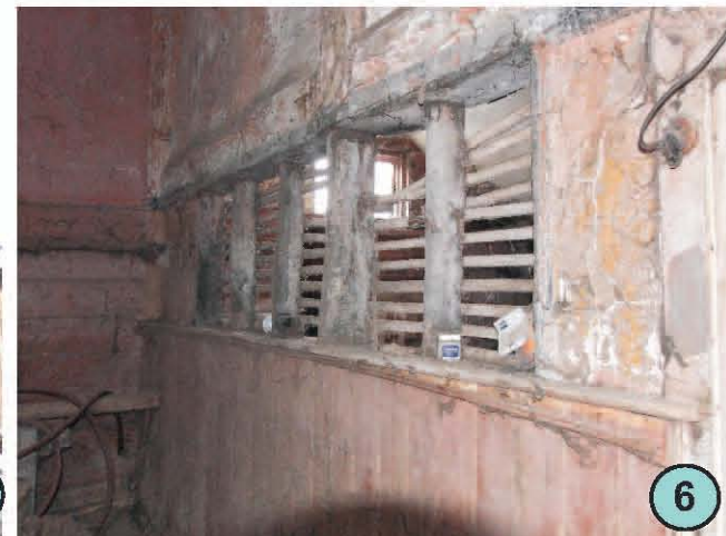
Converted end wall of barn when stable extension added. Existing wall studs worked to form mullions for ventilation window between stables. Some board lining and parts of feed trough survive in end bay, the rest was plastered and ceiled at tiebeam height.
