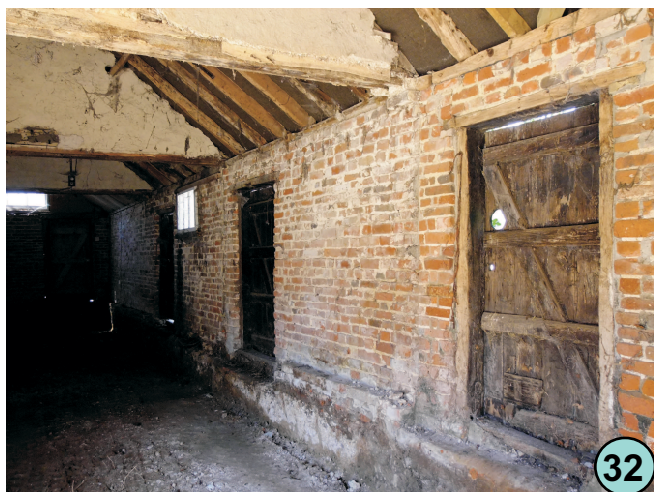
View to south in C19 shelter/storage sheds with minimal partitions removed but plastered area of gables left in place. Both windows are late insertions. Brickwork only fair faced to outside west.
