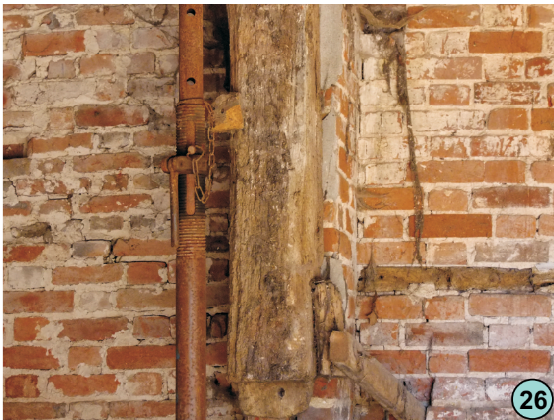
Junction of walls to the north showing later build on the left tending to fall away.
