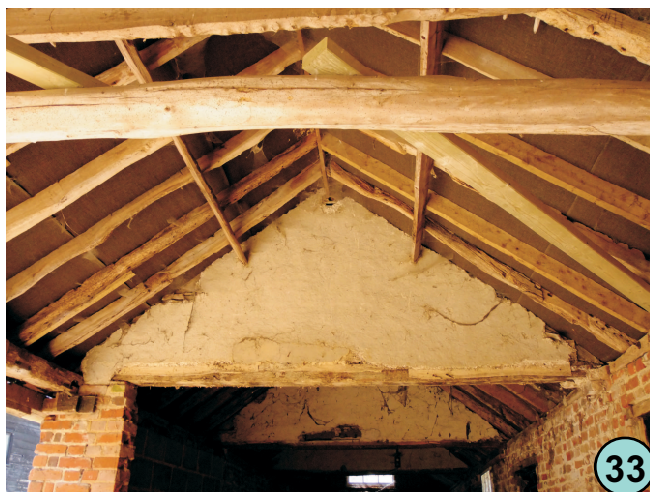
Typical area of roof structure with re-cut reused timber and all reworked in twentieth century. Was closed brick end wall under gable against start of open area to the north.
