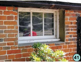
Window in the west wall of the range cut into the brickwork at a later date. This is beyond the area of conversion.
