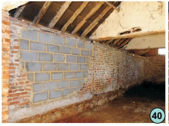
East wall of closed section of the west range, previously repaired with blockwork. Note vertical lines at cross divisions where end timber of infill was mortared to wall.
