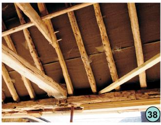
View in C19 west range looking up to show typical roof Detail in roof showing some reused timbers that have construction with reused timbers. Simple scarf joints but collars are pegged.
