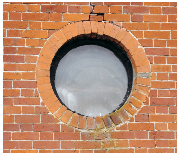
Circular window to upper floor from rubbed bricks.
