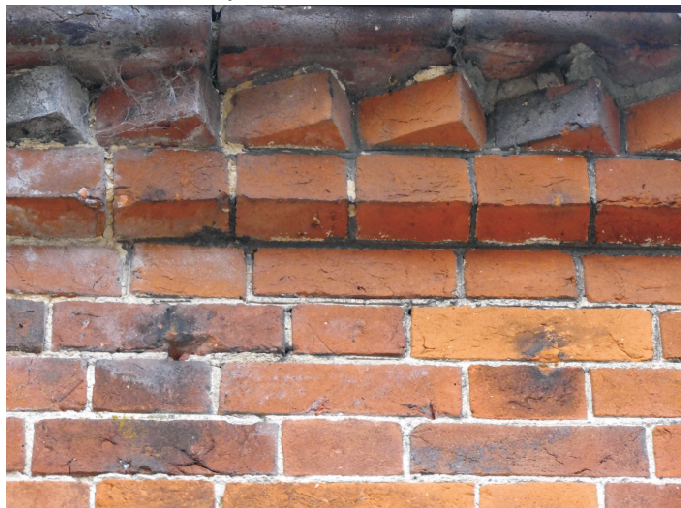
Dog tooth detail under eaves. Flemish bond brick below.
