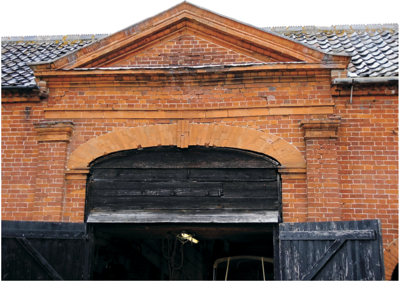
Detail at main opening with rubbed semi-elliptical arched head flanked by pilasters with string course above surmounted by pedimented head detail in rubbed and moulded brick.
