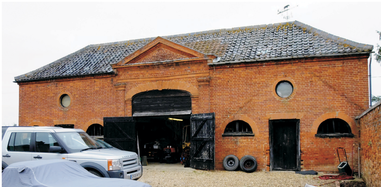
Front south easterly view of the coach house. Note scar from C19 shelter shed roof and lowered main doorway.
