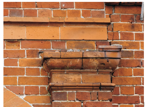
Detail at main opening with rubbed semi-elliptical arched head flanked by pilasters with string course above surmounted by pedimented head detail in rubbed and moulded brick.
