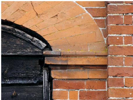
Detail at main opening with rubbed semi-elliptical arched head flanked by pilasters with string course above surmounted by pedimented head detail in rubbed and moulded brick.
