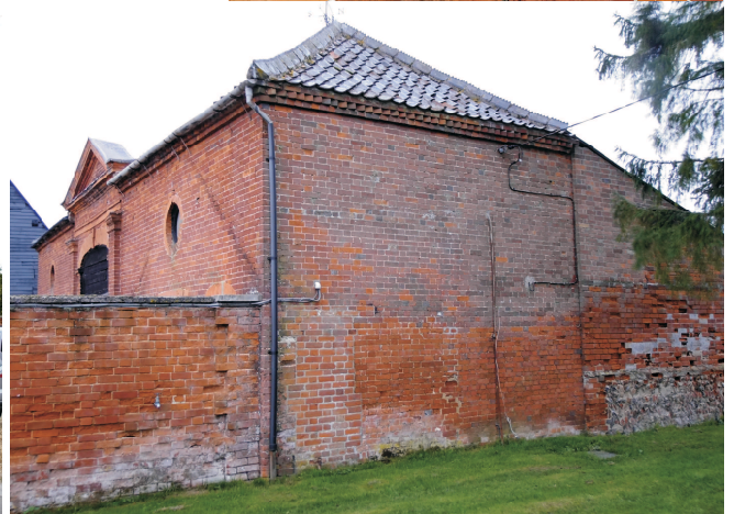
North east elevation from moated area. Infilled doorway at lower left hand side. Brick wall to lean-to most likely part of garden wall. Wall to left is nineteenth century rear wall of shelter sheds now removed.
