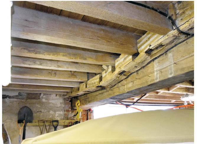
Head beam for lower floor partition to side of central carriage area. This side (to right of opening) is on the opposite side of the main beam. On the other side it is fitted to the inside of the main beam suggesting that the floors to this side went in later. Note elm joists.
