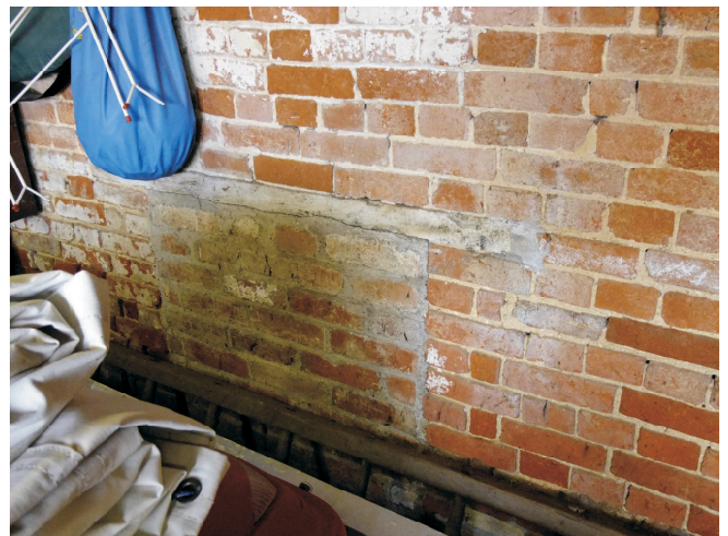
Example of filled in mucking out hole in north west wall. These are situated to either side of the central bay.
