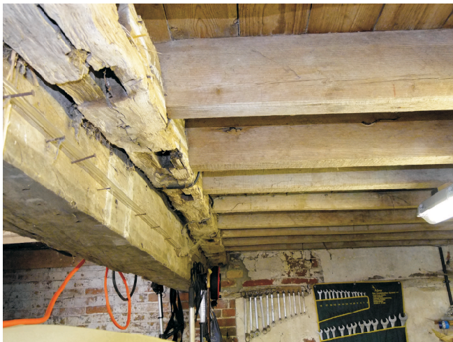
Head beam for lower floor partition to side of central carriage area. This side (to right of opening) is on the opposite side of the main beam. On the other side it is fitted to the inside of the main beam suggesting that the floors to this side went in later. Note elm joists.
