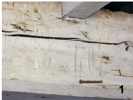
Examples of 'bracking' marks, or Scandinavian shipping marks on softwood floor beams. These marks made with a race knife here show some recognisable similarities between the various marks.
