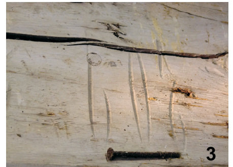
Examples of 'bracking' marks, or Scandinavian shipping marks on softwood floor beams. These marks made with a race knife here show some recognisable similarities between the various marks.
