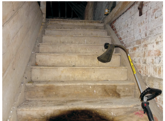
View up staircase show the width and well constructed detail.
