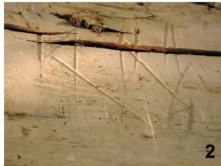
Examples of 'bracking' marks, or Scandinavian shipping marks on softwood floor beams. These marks made with a race knife here show some recognisable similarities between the various marks.
