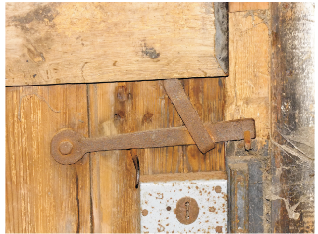
Example of door catch.
