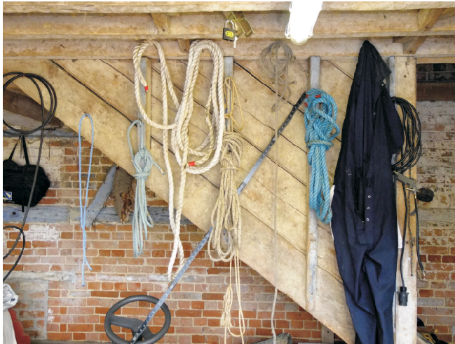
Inserted staircase at rear of main opening. Framed at same time as floor inserted over this area.
