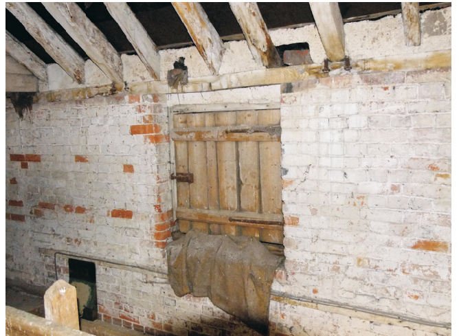
Detail of 'Pitching' door showing boarded construction with two ledges and lighter hinges than those on the main doors. Brickwork shows wear areas to the lower sections of the opening.
