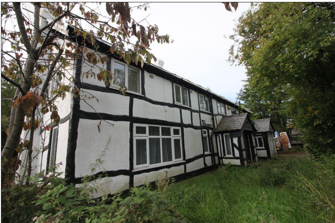
Plate 17: Eastern end of the northern elevation, facing south-west
