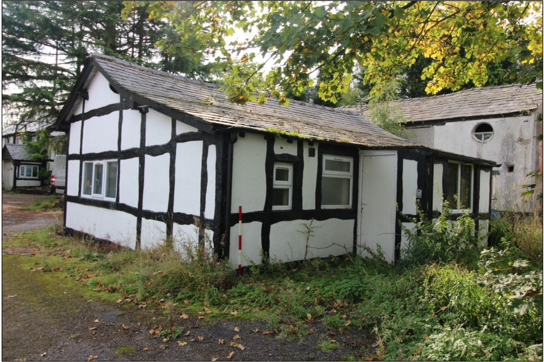
Plate 6: Western elevation and northern gable facing south-east, 1m scale
