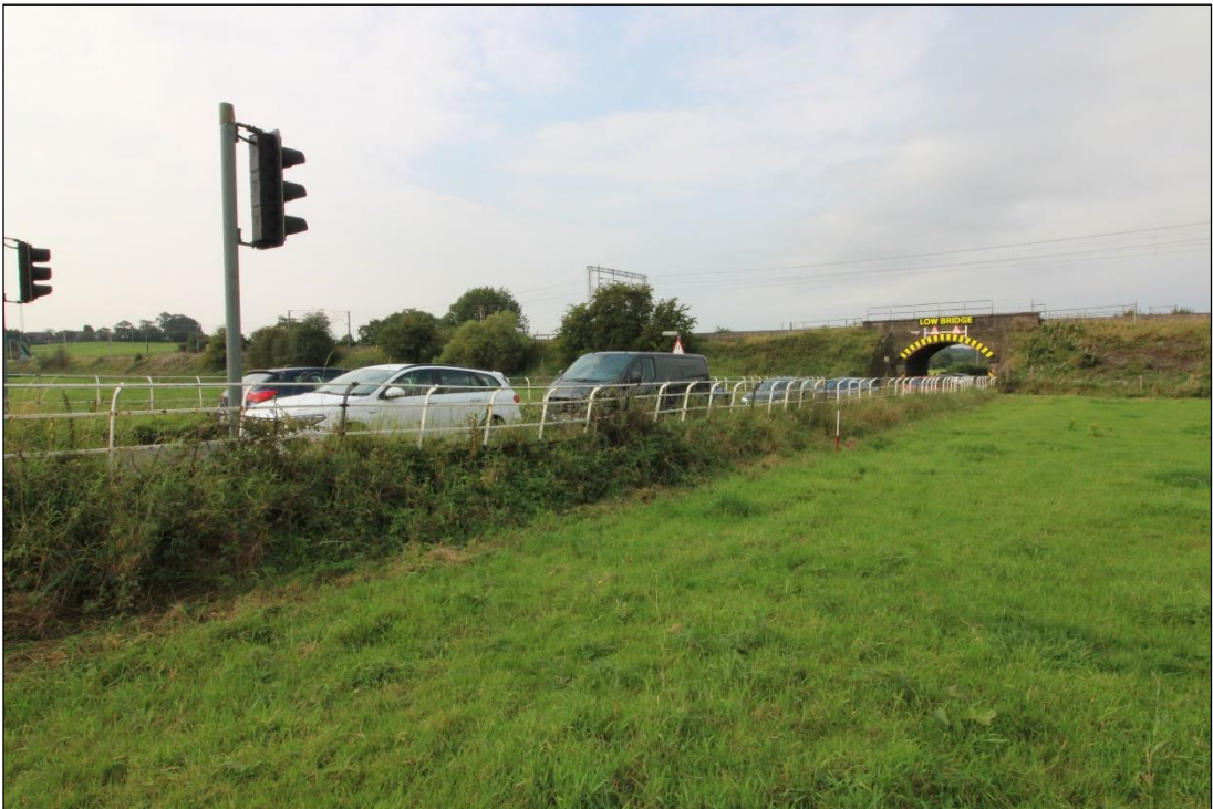
Plate 71: Iron railings, facing south-west towards railway bridge, with 1m scale
