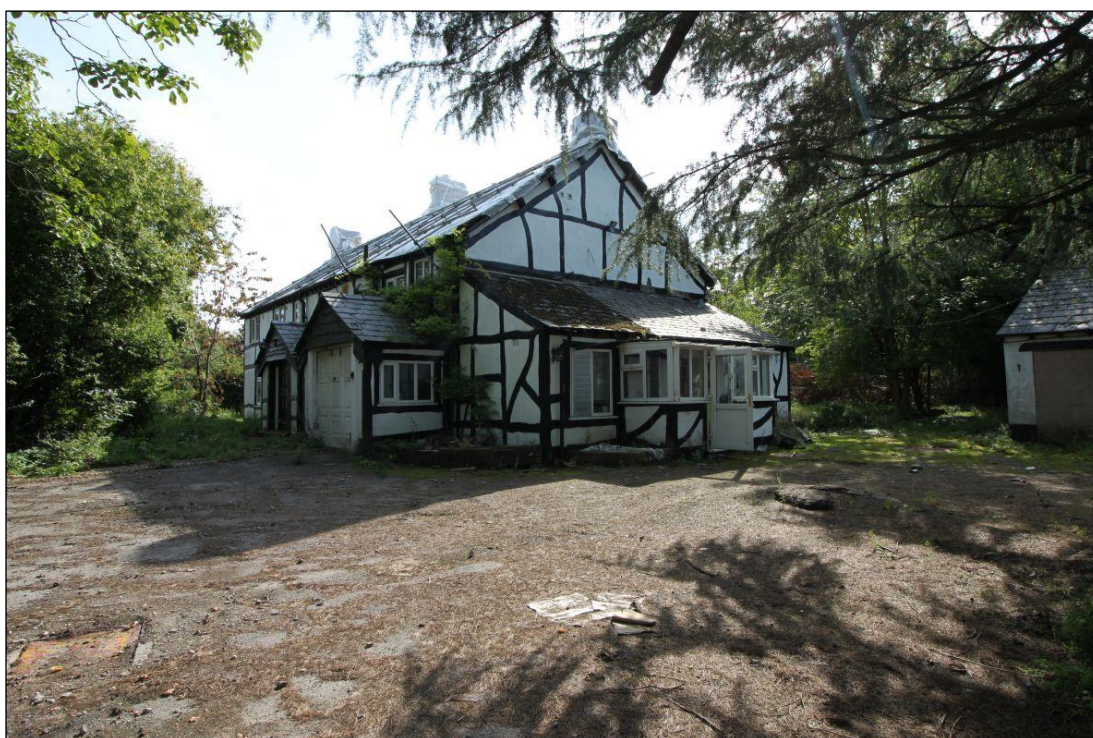
Plate 15: Walnut Tree Farmhouse, facing south-east
