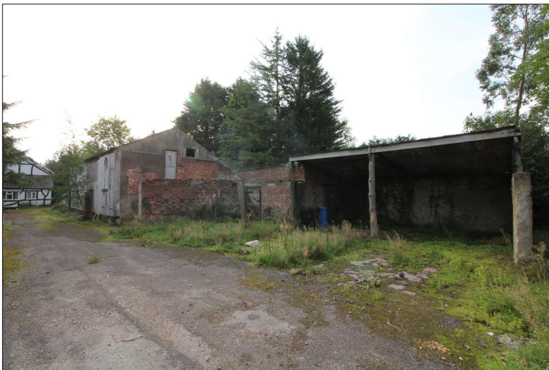
Plate 12: Open-fronted Sheds to west of Shippon, facing south-east
