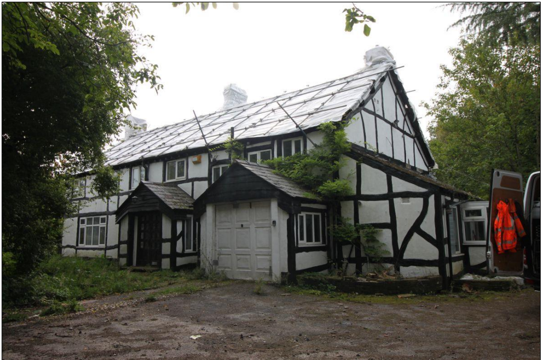
Plate 16: Northern elevation, facing south
