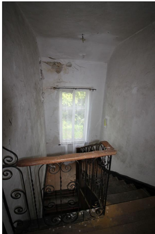
Plate 33: Staircase, facing north
