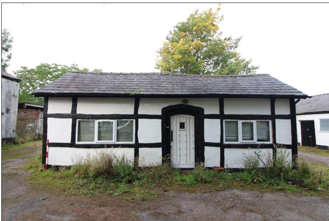
Plate 4: Eastern elevation, facing west
