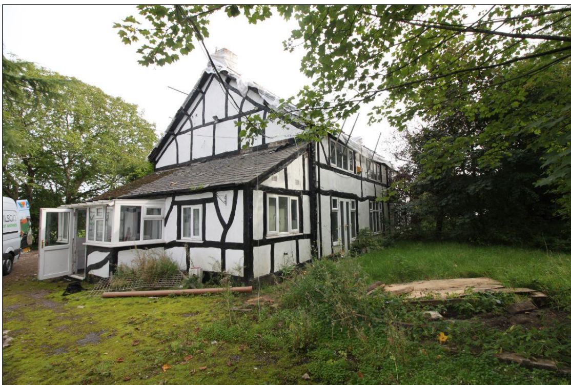
Plate 19: South-western corner, facing north-east
