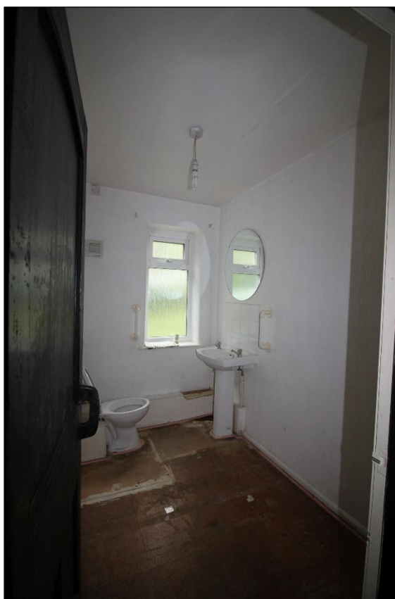
Plate 27: Ground Floor bathroom, facing north
