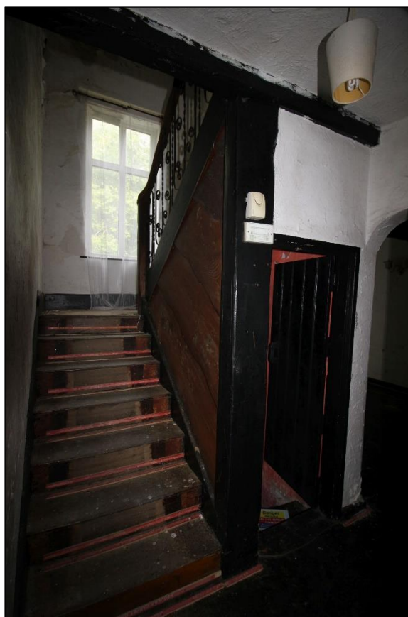
Plate 25: Staircase to first floor
