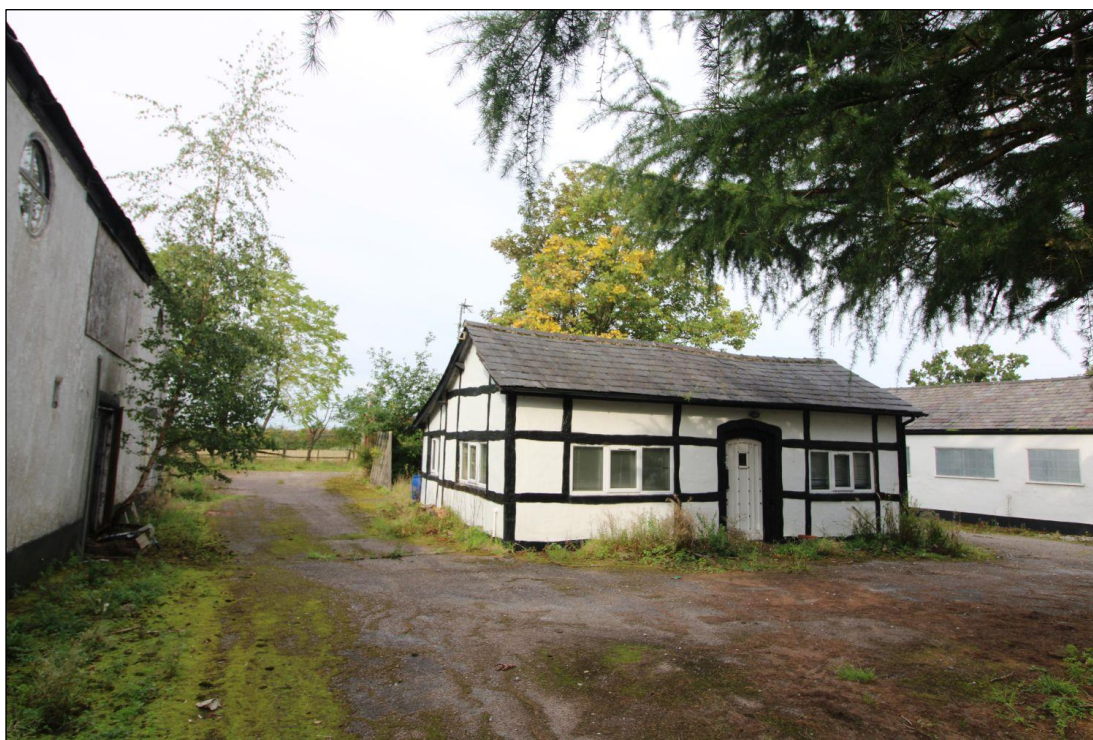
Plate 3: Walnut Tree Farm Cottage, facing north-west
