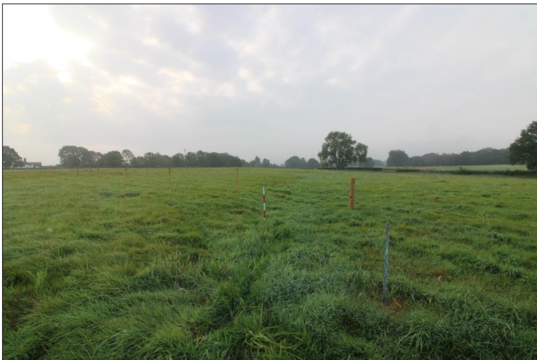
Plate 79: Earthwork, facing south-west, with 1m scale
