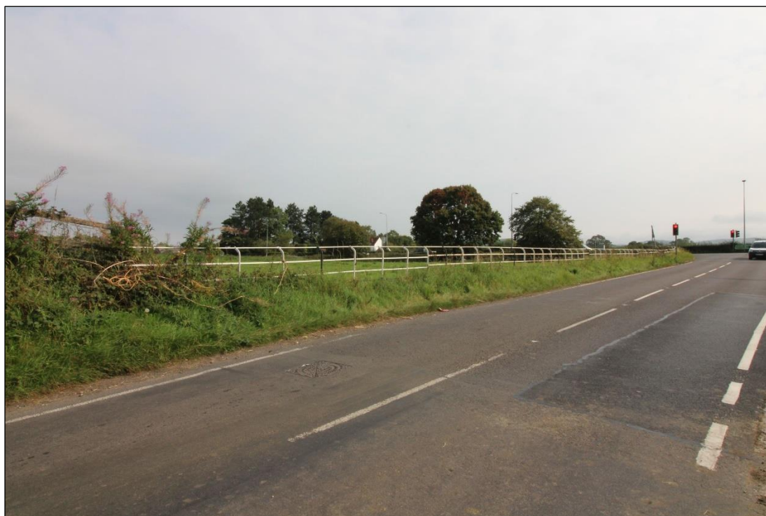
Plate 70: Iron railings, facing north-east along Bonis Hall Lane
