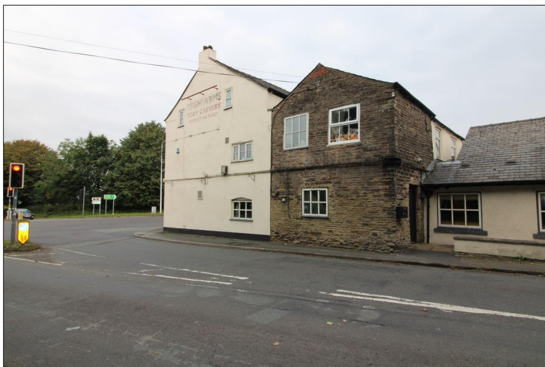
Plate 59: Legh Arms, facing north-west
