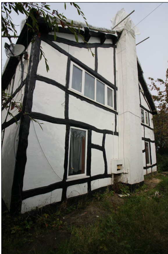
Plate 20: Eastern elevation, facing north-west
