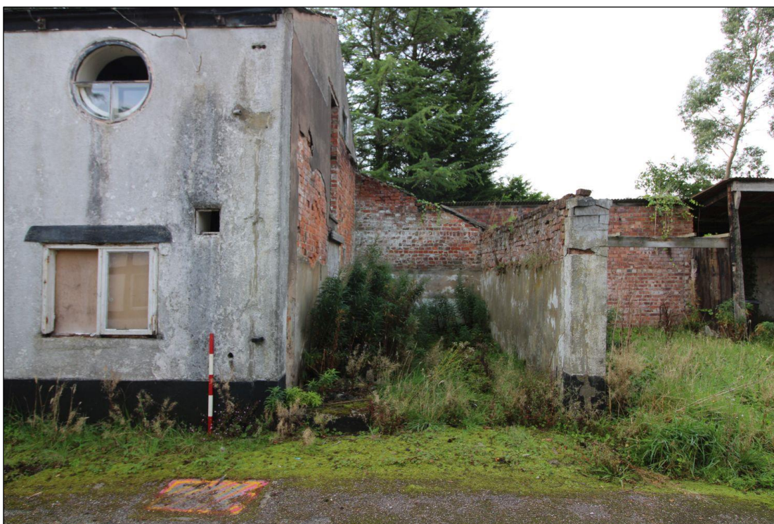
Plate 11: Unroofed western Lean-to extension, facing south with 1m scale
