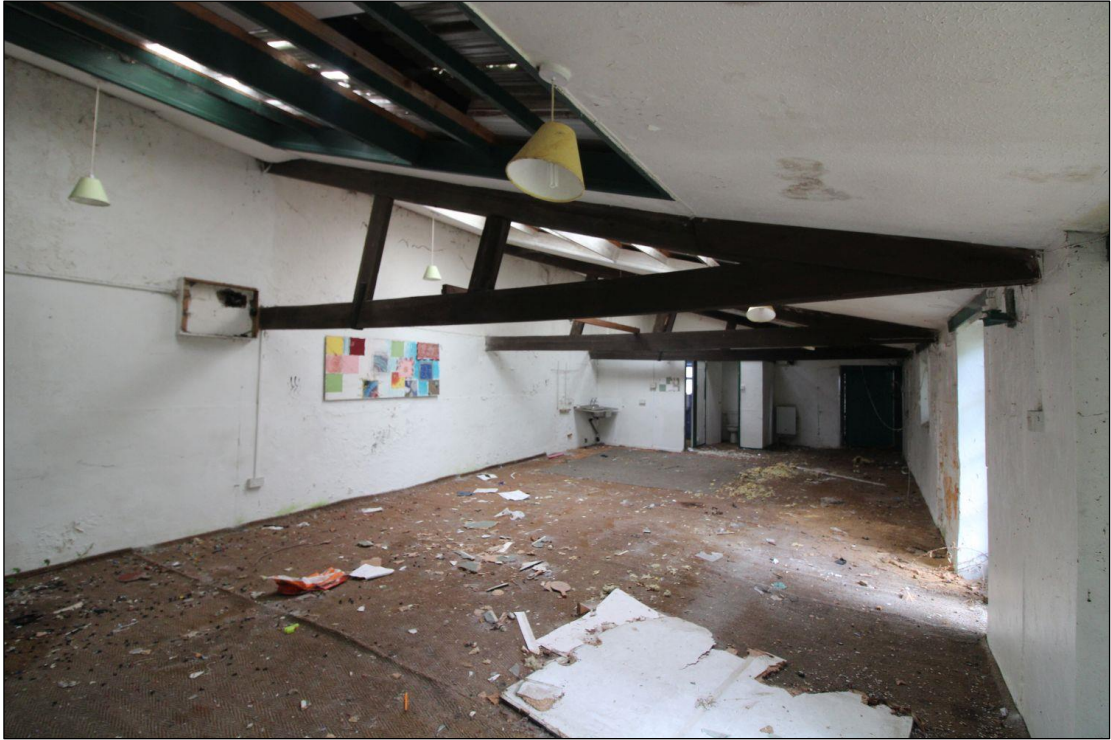
Plate 14: Interior of Lean-to, facing east
