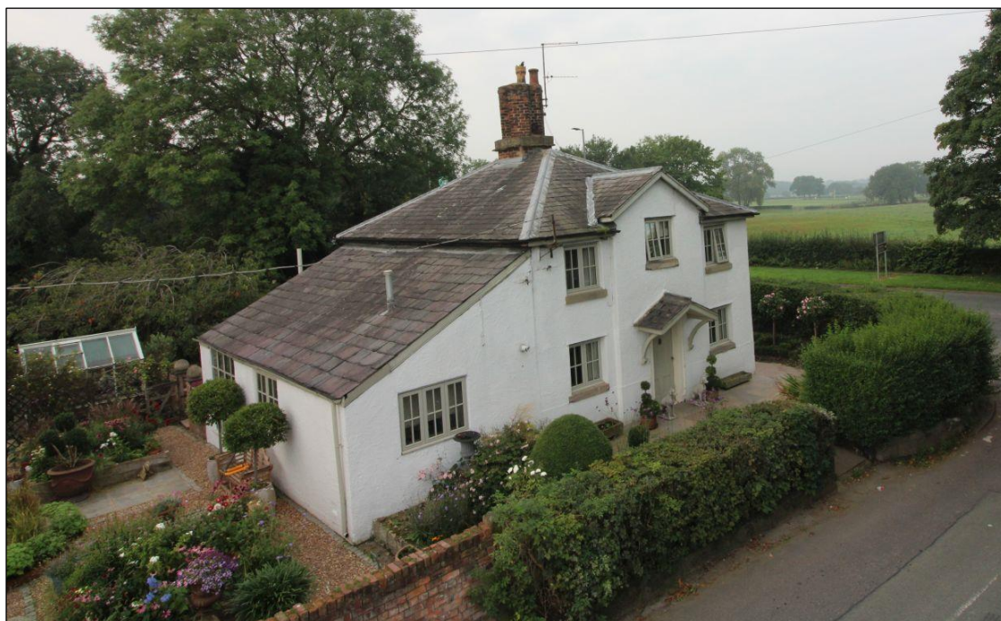
Plate 54: Street Lane Farmhouse, facing south-west
