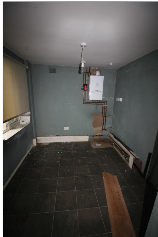
Plate 23: Utility Room, facing north
