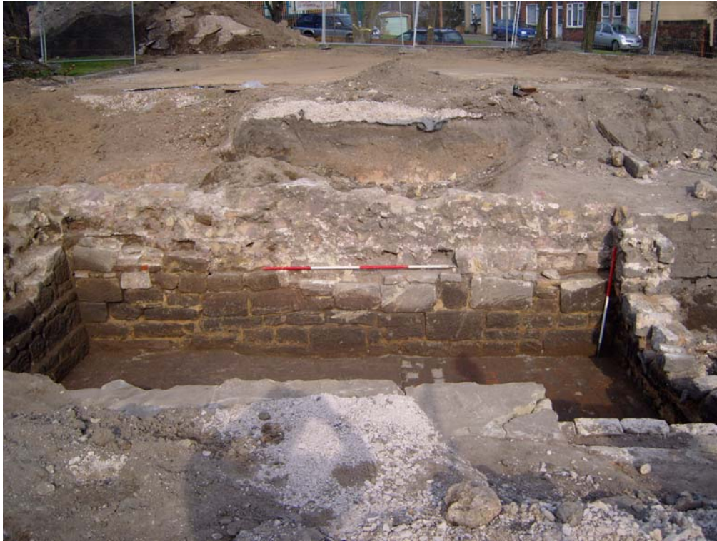
Plate 13: The north-eastern cellar wall, showing the contrast between the earlier wall, 3050 , bonded with pink mortar, and the later cellar wall, 3133 , bonded with yellow mortar
