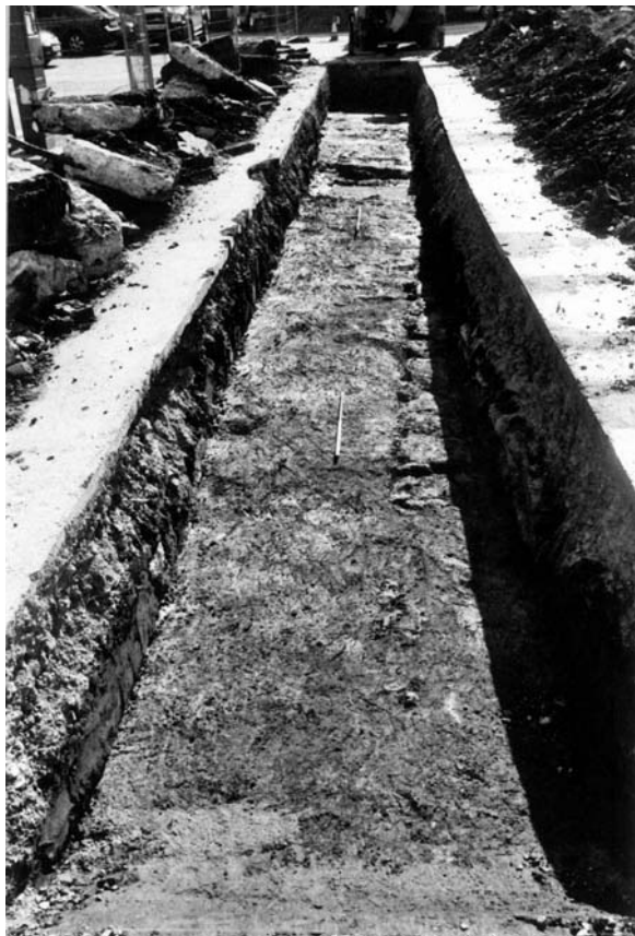
Plate 6: Trench 24, viewed towards the south-west, with culvert 2404 extending towards the centre right
