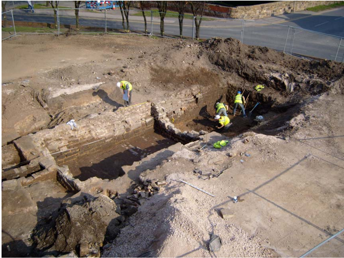
Plate 19: General view of the cellared building during excavation, viewed from the west
