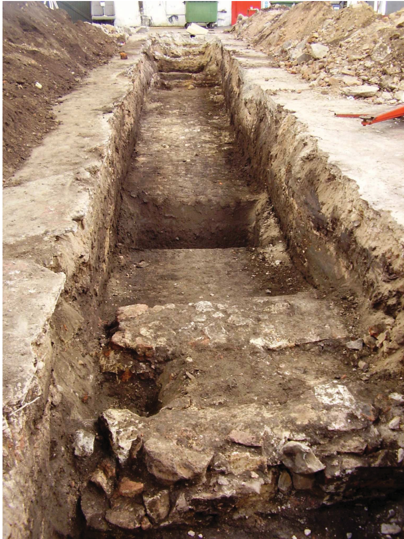
Plate 1: Trench 1; viewed toward east, showing culvert 104 .
