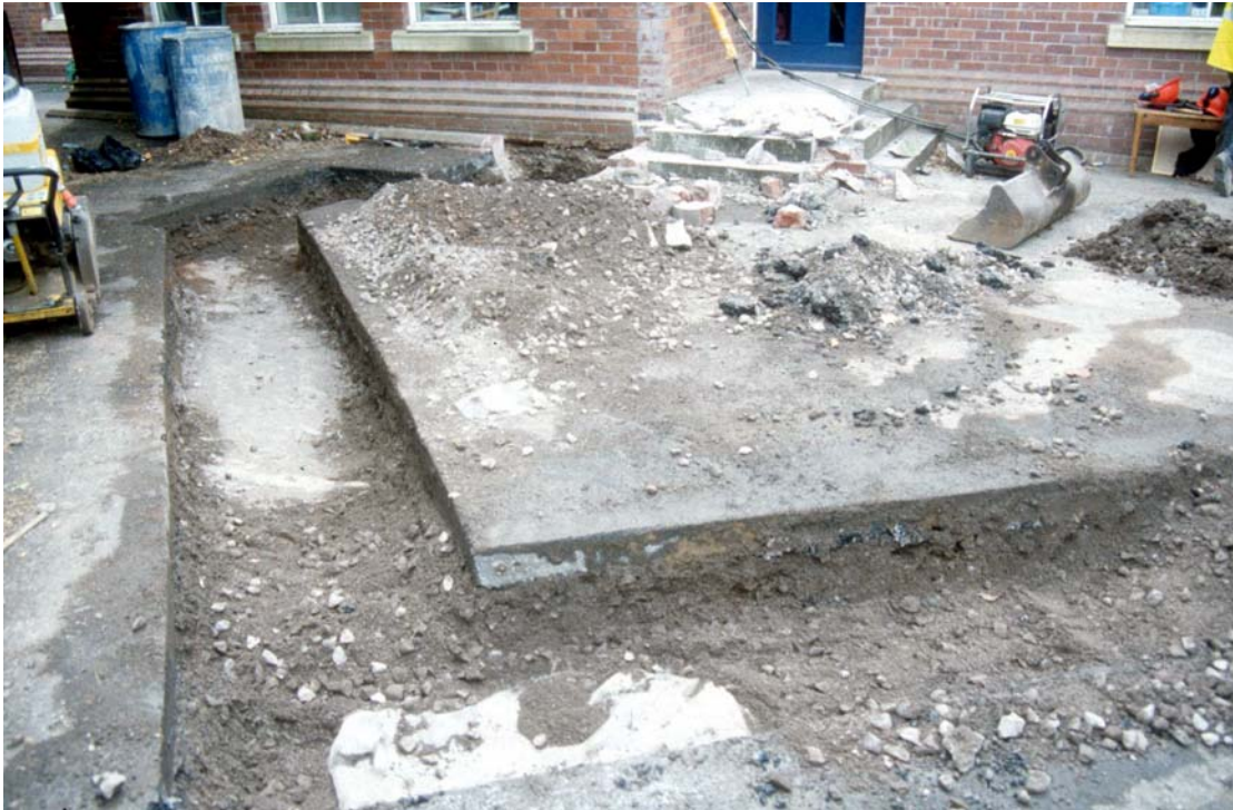
Plate 1: Showing excavated foundation trench
