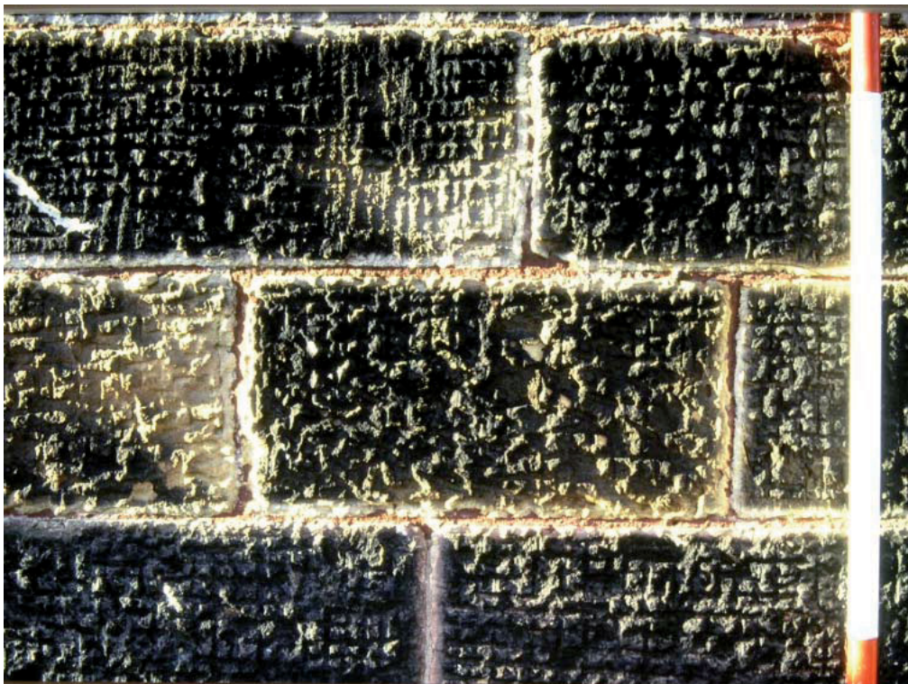
Plate 3: Tooling on main elevations
