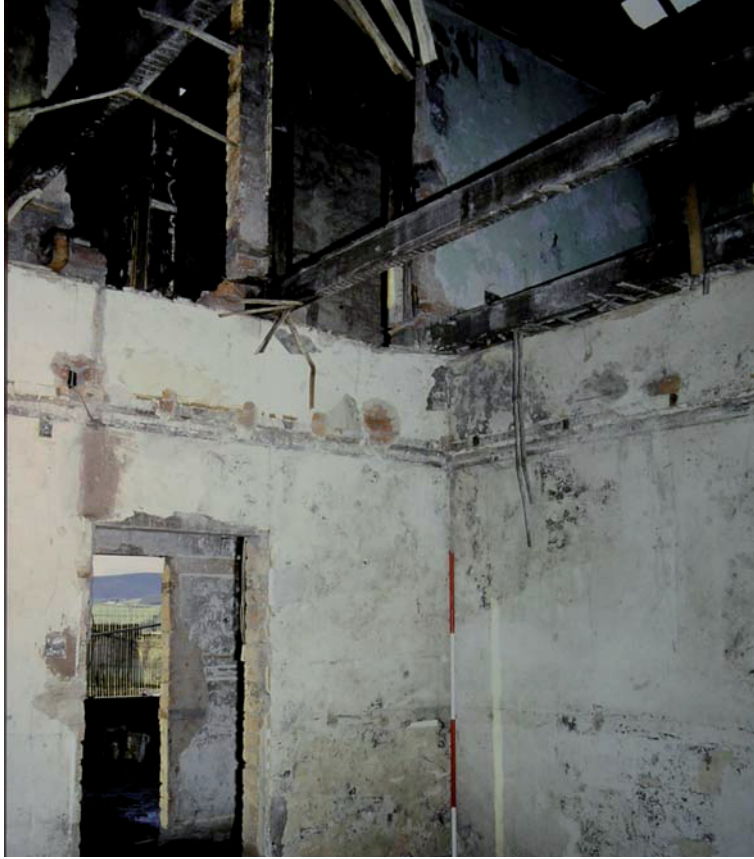
Plate 12: Room 2 facing north-west
