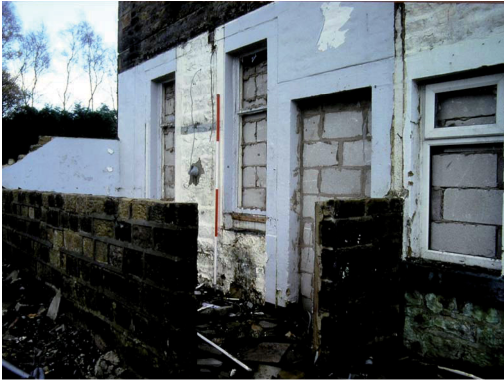
Plate 6: Detail of rear outshut
