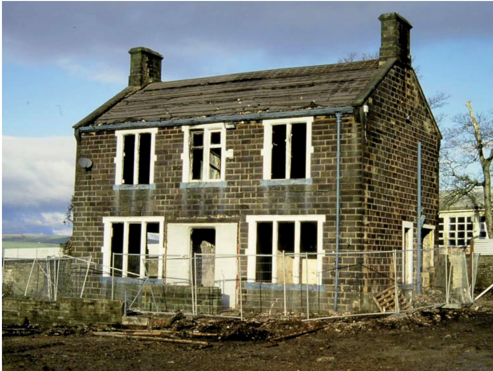
Plate 2: General view of front of house
