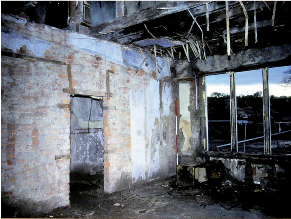
Plate 4: General view of Room 4
