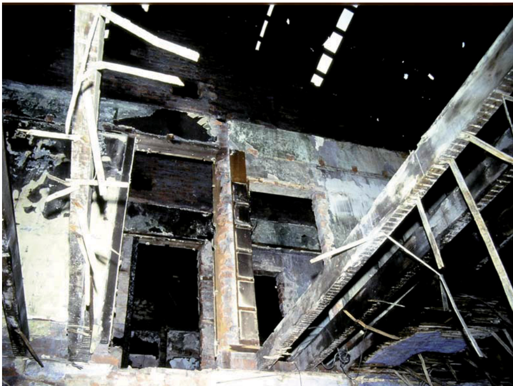
Plate 15: Doorways on first floor
