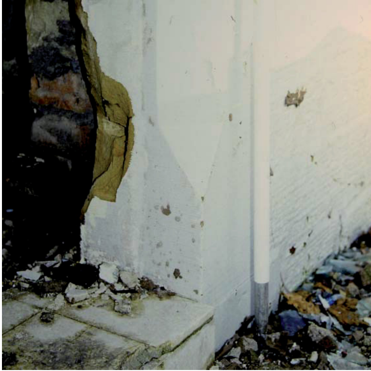
Plate 8: Detail of base of front door
