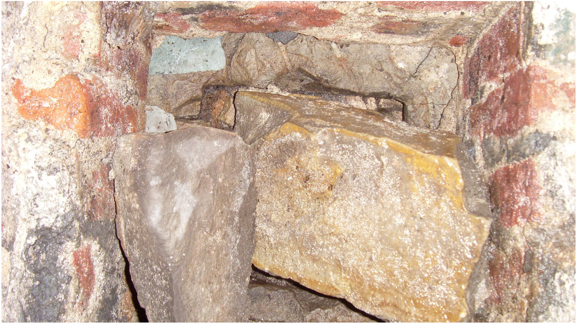
Plate 12: Blocked coalhole 1040 access to Church Lane, approximately 0.4m square
