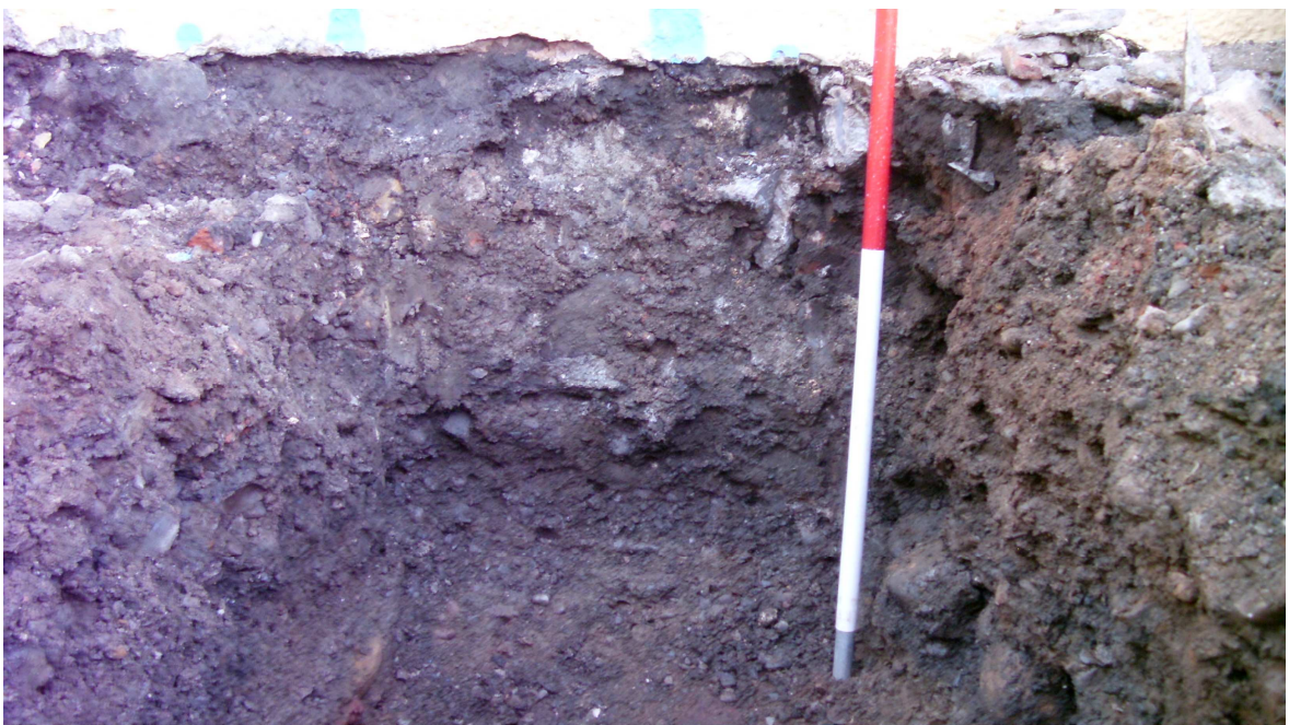
Plate 5: View to the west of the foundations of 111 Church Street and underlying made ground 1032 overlying natural 1001
