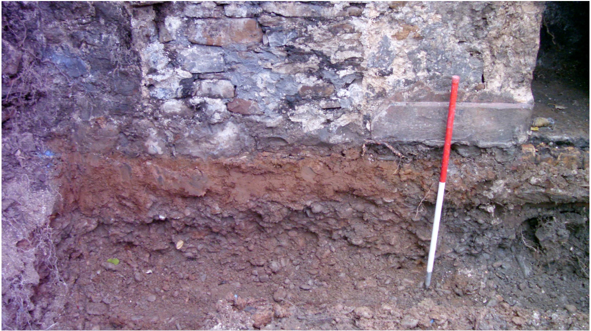
Plate 8: View to the south of the tenement wall 1024 , skirting board 1021 , foundation stones 1025 , and clayey sand levelling deposit 1027 , on natural ground 1001
