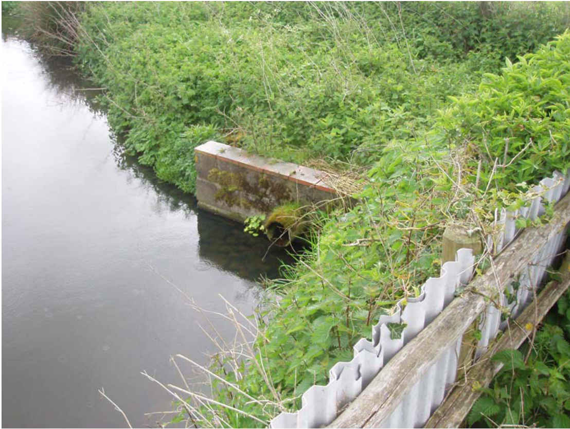
Plate 3: Site 11, drainage pipe discharging into pond
