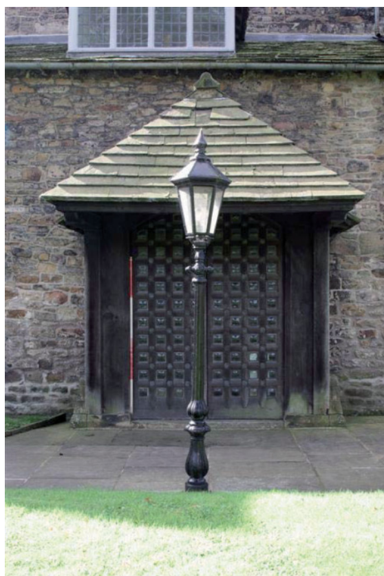
Plate 6: Exterior of north porch prior to works
