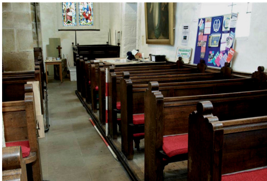
Plate 7: General layout of north aisle prior to works
