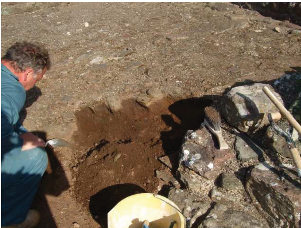
Plate 6: Working shot of remedial works
