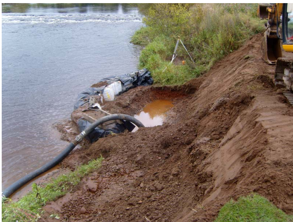
Plate 2: General shot of the river bank and foundation trench, looking north-east
