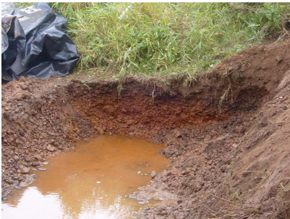
Plate 3: Close-up of the south-west-facing section through the foundation trench
