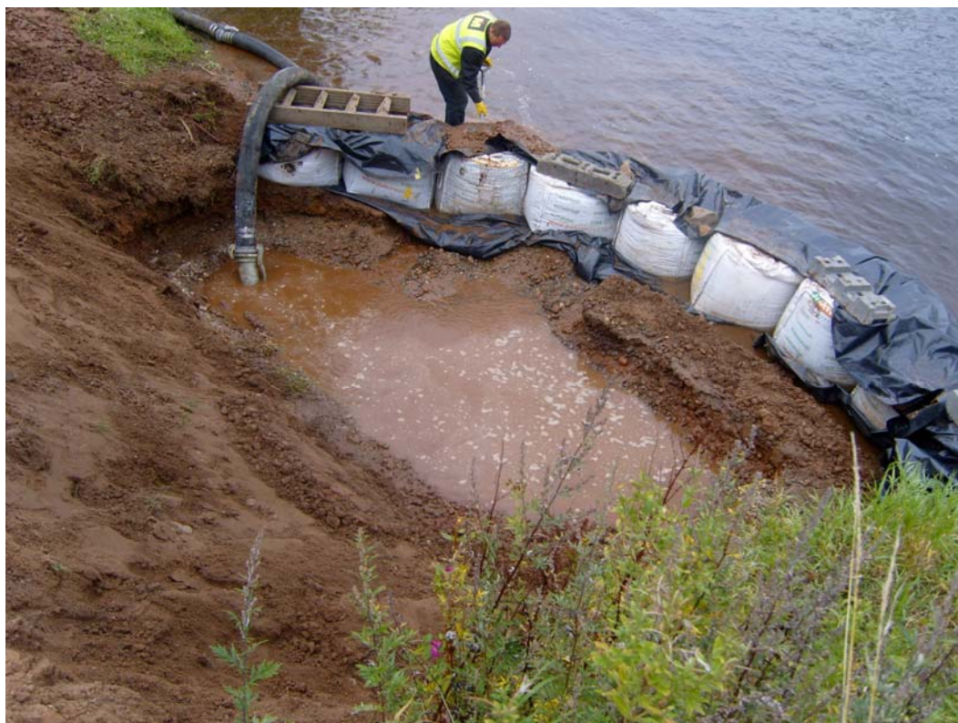
Plate 1: Working shot looking south-west
