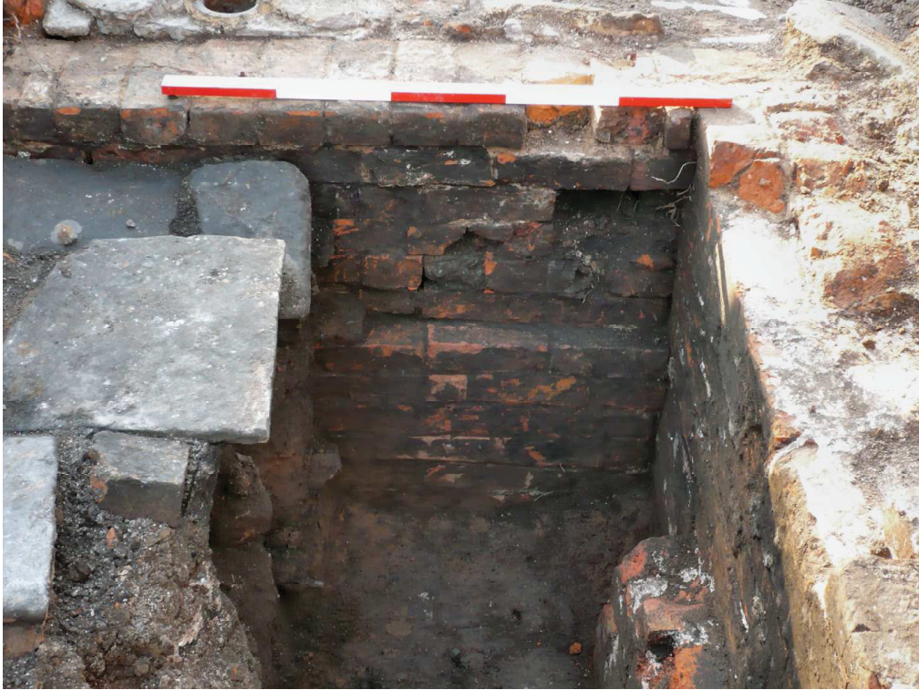
Plate 3: Trench 17, slot through the western end showing walls 114 , and 115 to the right, looking west
