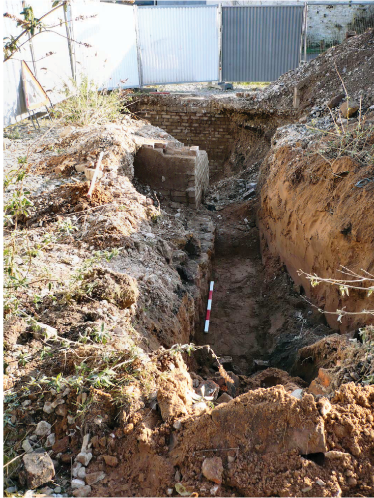
Plate 7: Trench 29, general shot looking south-west
