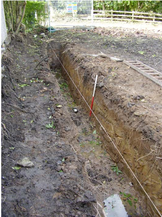
Plate 3: Southern east/west aligned footing trench for Plot 2, west-facing
