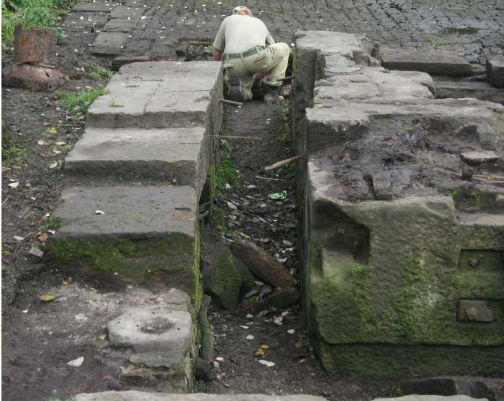
Plate 13: The engine flywheel pit
