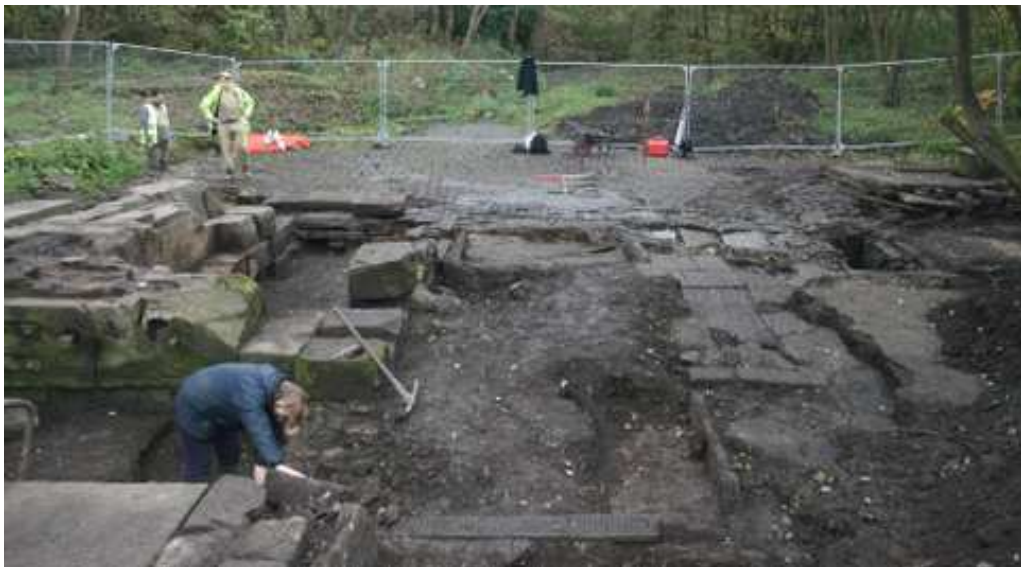
Plate 17: General view from the west showing engine house (left), bleaching tanks (centre), Phase 1 and 2 floors and culvert (right), Phase 3 platform (top right), and yard (top)
