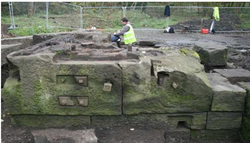
Plate 11: Fixing bolts in the engine bed, for column (top) and condenser
