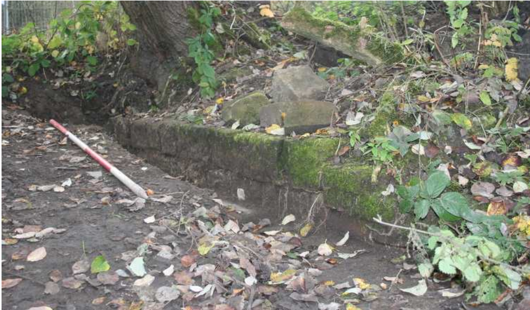
Plate 21: East wall of bleachworks, 022, with dressed and coursed external stone facing
