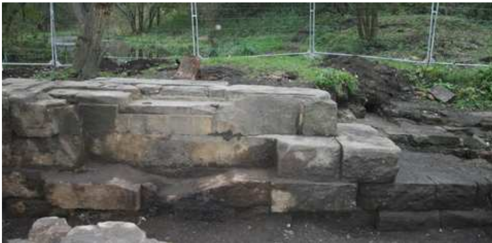
Plate 10: Dressed stone blocks of the engine bed, with cut-away for the crank
