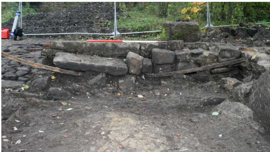
Plate 20: East wall of bleachworks, with possible tramway rails, overlain by platform 015
