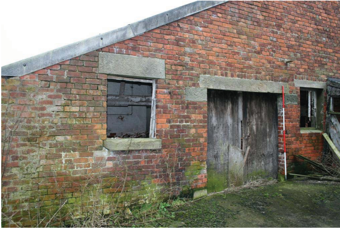
Plate 9: North end of the west elevation of Barn B
