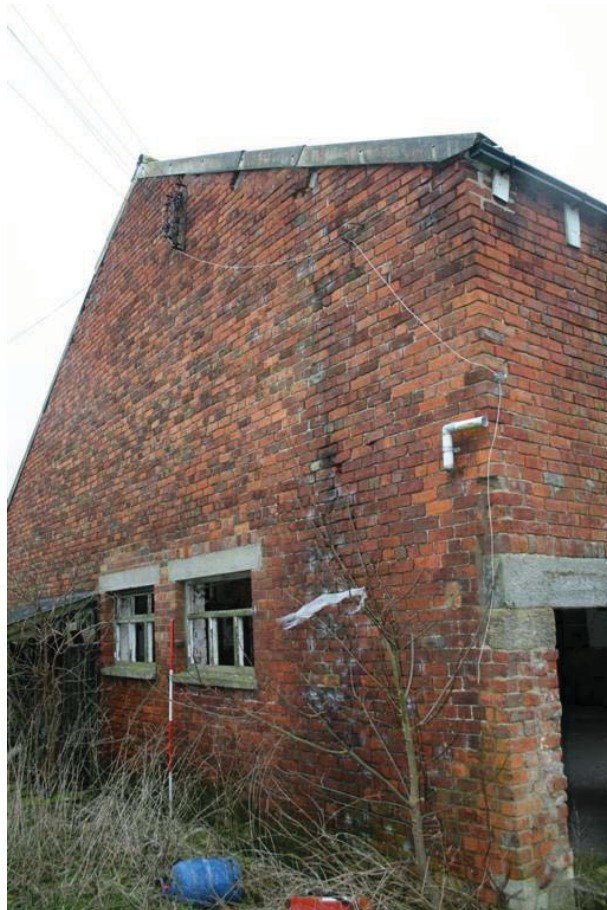
Plate 10: East end of the north elevation of Barn B
