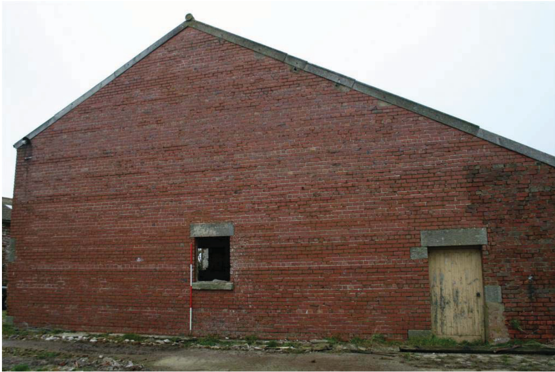
Plate 11: South elevation of Barn B
