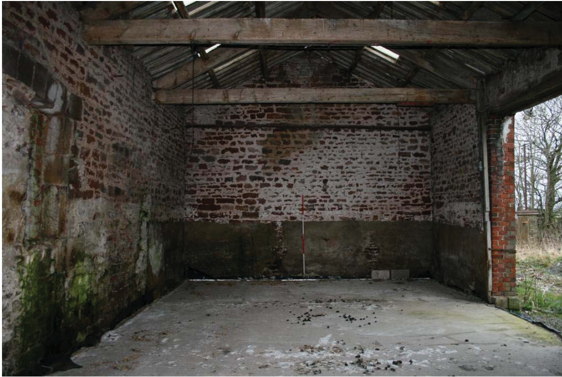
Plate 13: Internal view of Barn A
