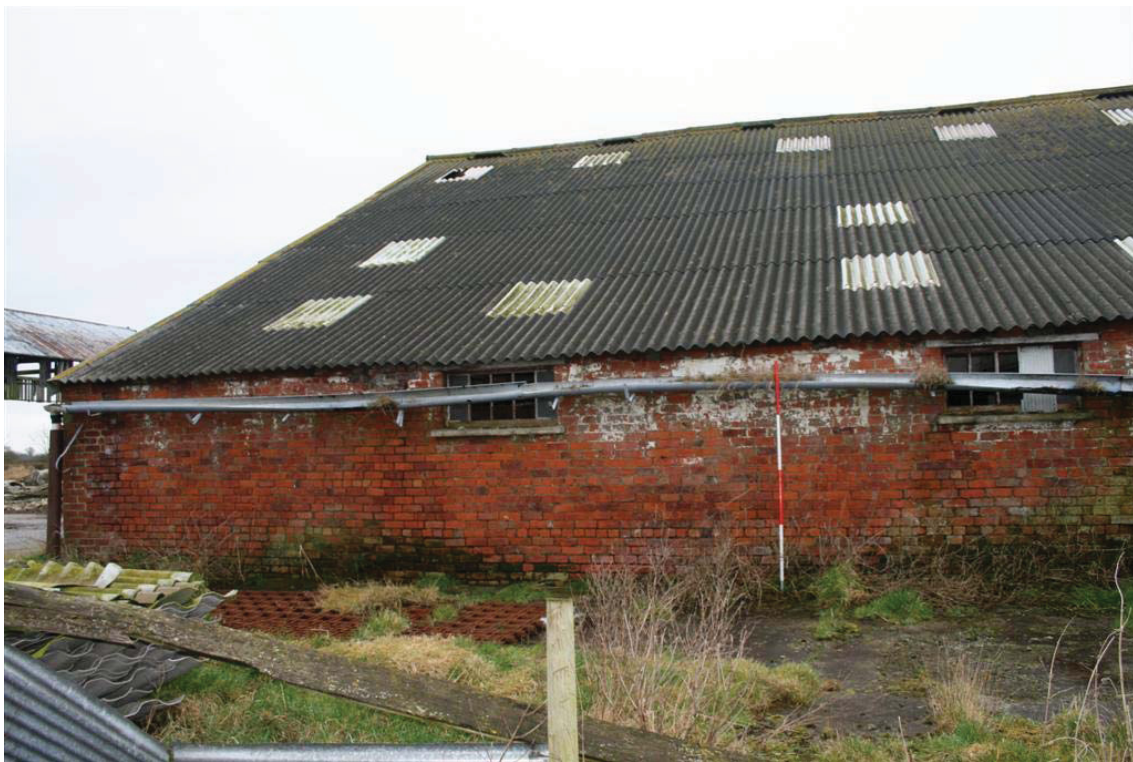
Plate 12: East elevation of Barn B
