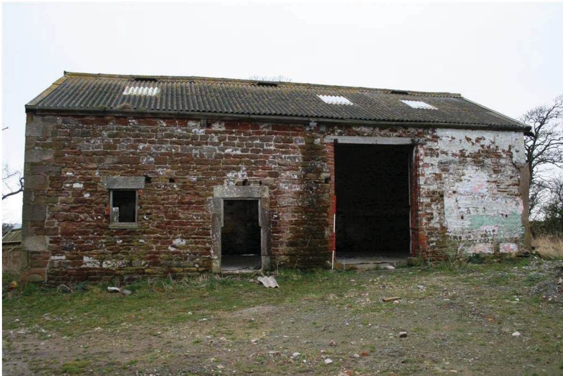
Plate 2: East-facing elevation of Barn A
