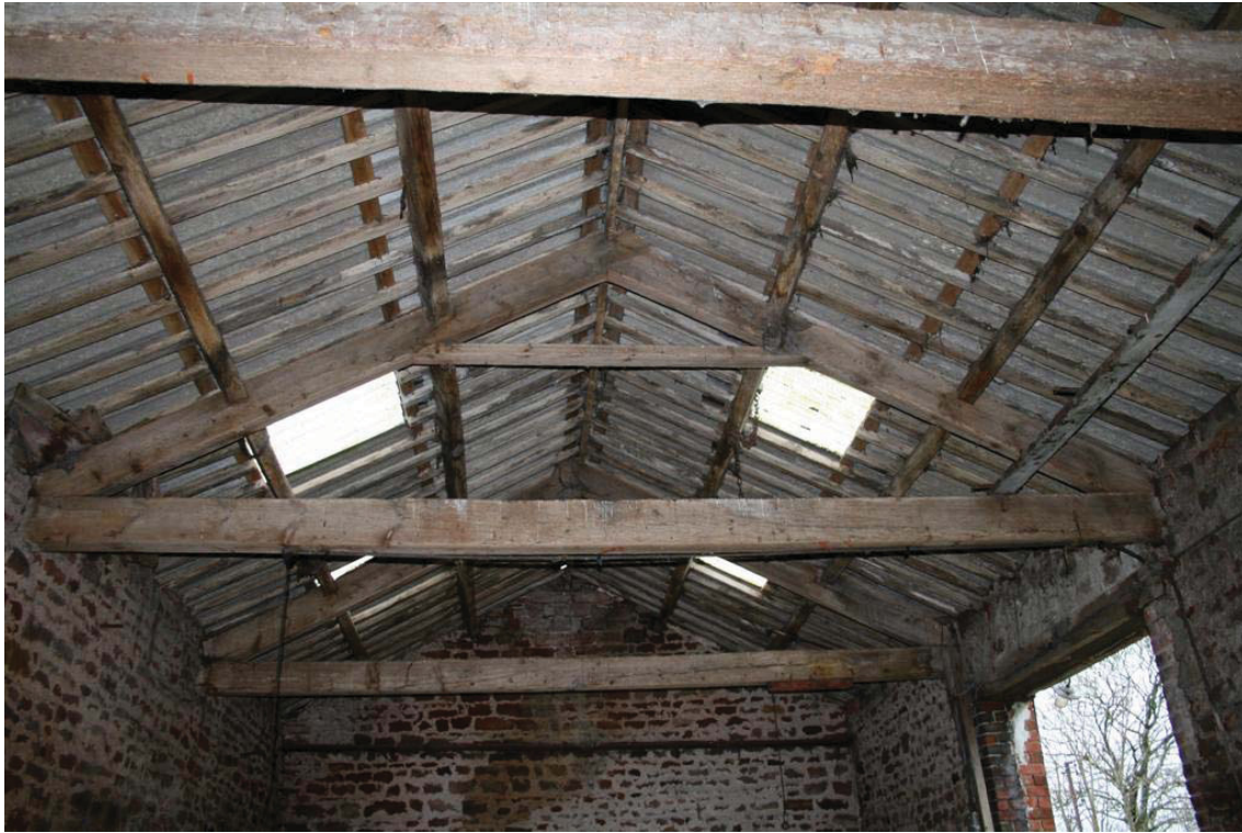
Plate 3: Roof truss in Barn A
