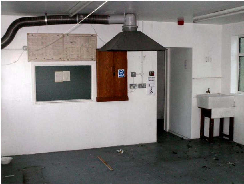
Plate 53: Example of an internal room within the military structures
