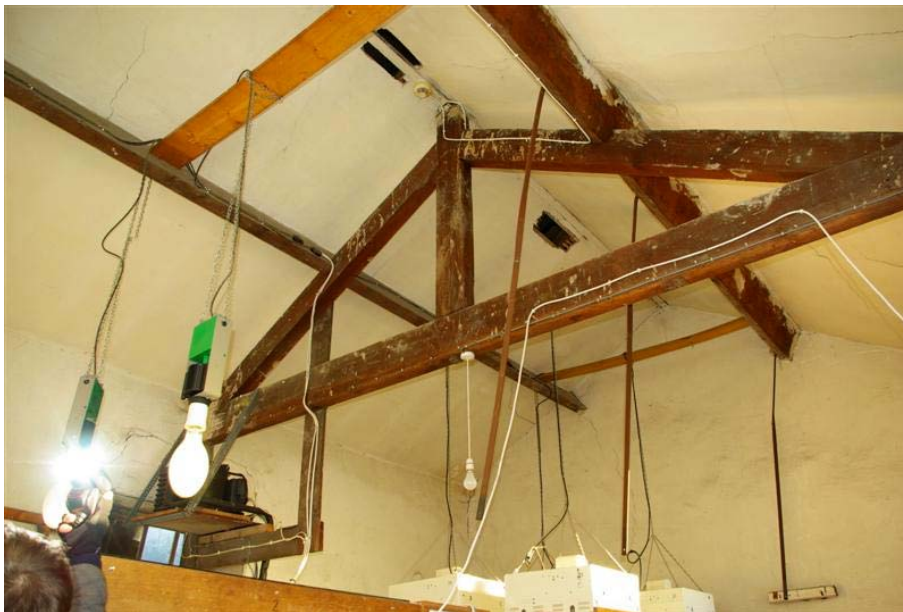
Plate 38: Truss in Room B3-14
