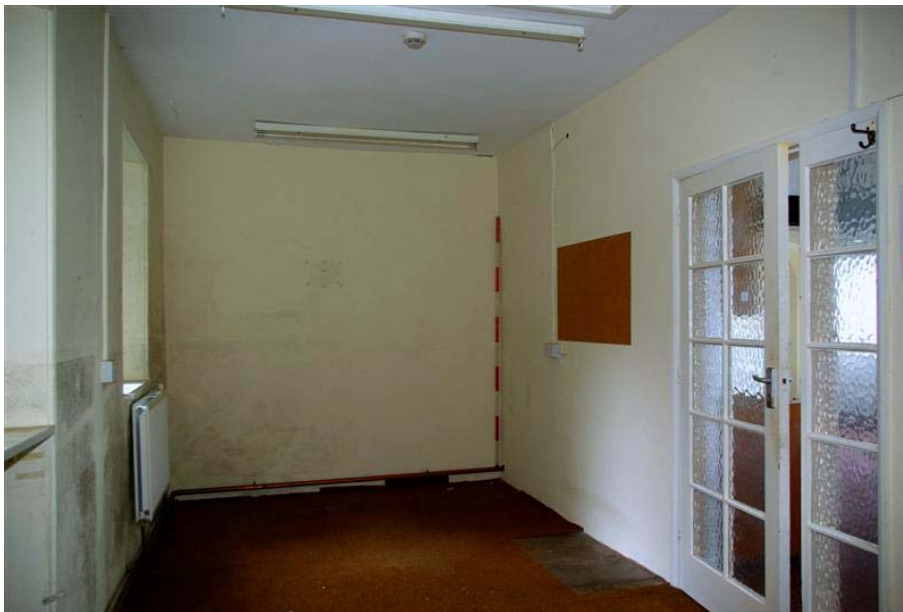
Plate 18: General view of Room B1-10 , facing north
