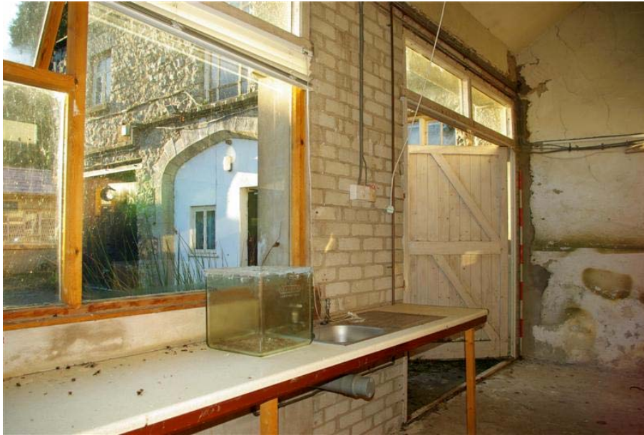
Plate 39: Rebuilt south elevation of the 'Growth Rooms', Building 3
