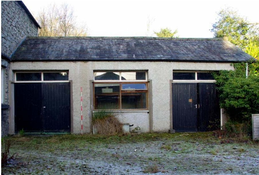
Plate 37: South elevation of the 'Growth Rooms' Building 3
