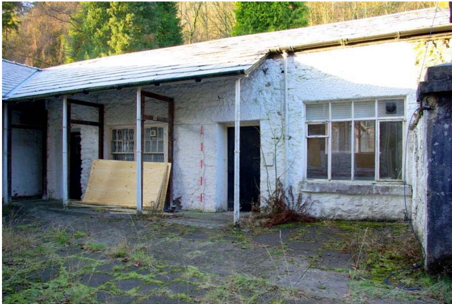
Plate 20: View of the east-facing elevation of Building 2
