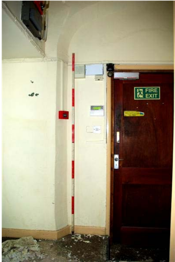
Plate 31: Internal view of entrance arch within Room B3-1
