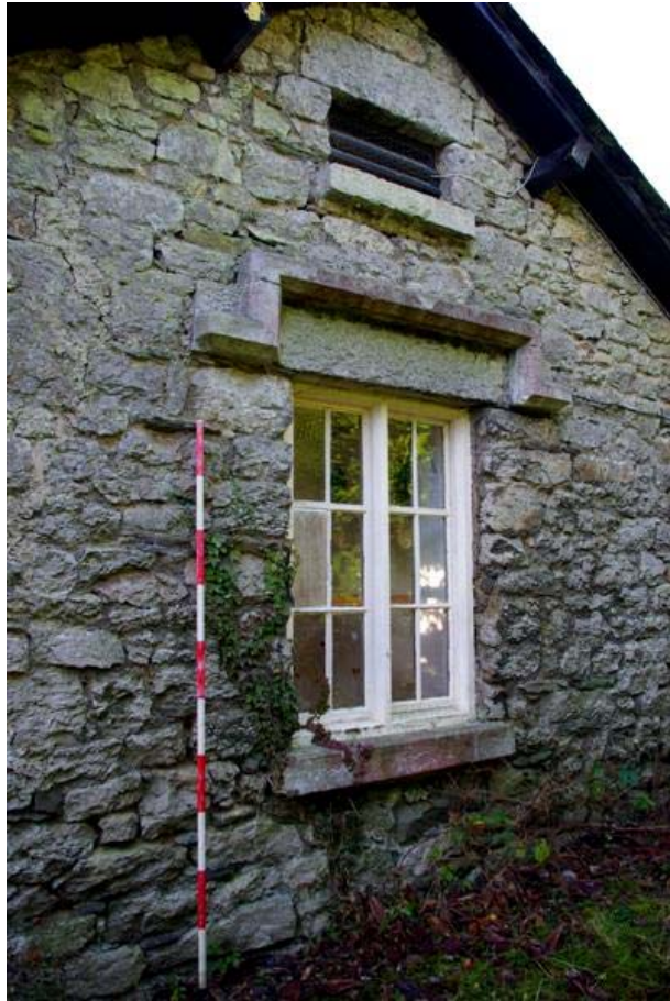
Plate 30: East gable elevation of the 'Growth Rooms', Building 3
