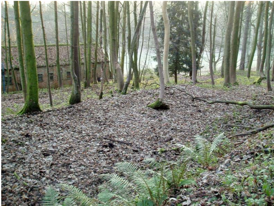
Plate 55: Further example of a concrete foundation platform, Building 8 in the background
