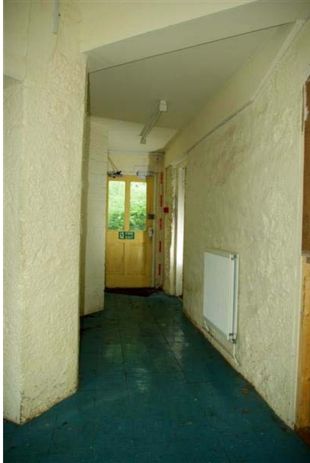
Plate 11: General view of Room B1-7 , facing east
