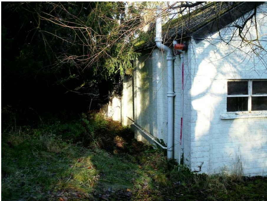
Plate 50: West elevation of Building 6
