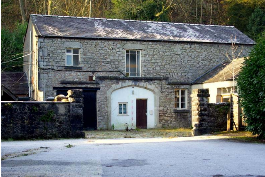
Plate 25: General view of Building 3, facing west
