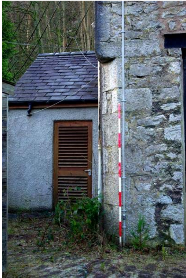
Plate 28: Chamfering at south-east corner of the Building 3
