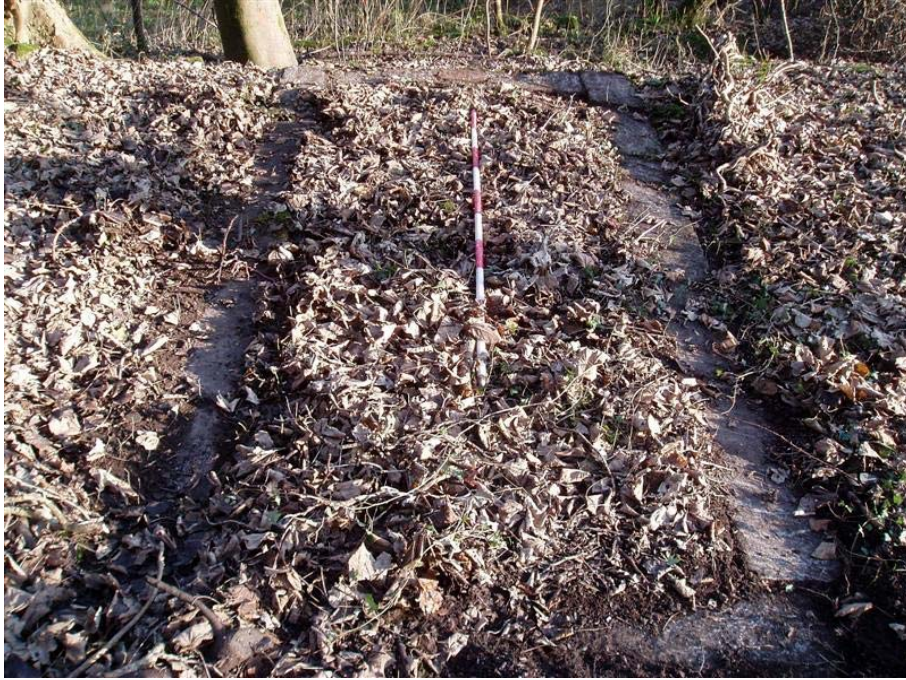
Plate 58: Rectangular concrete foundation on the terrace
