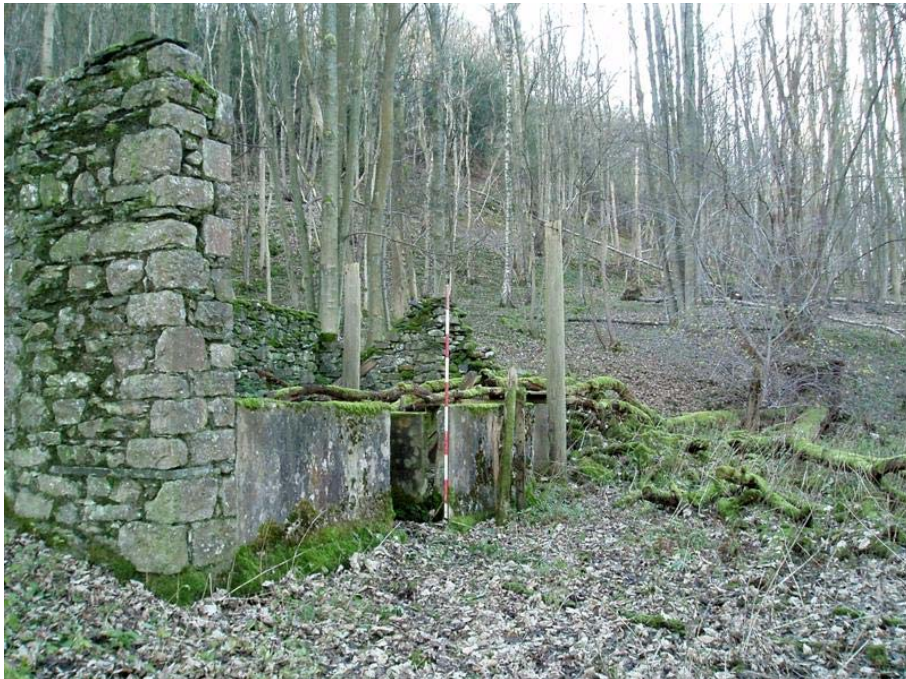
Plate 44: Derelict structure (Building 5 ) at the northern limit of the development area
