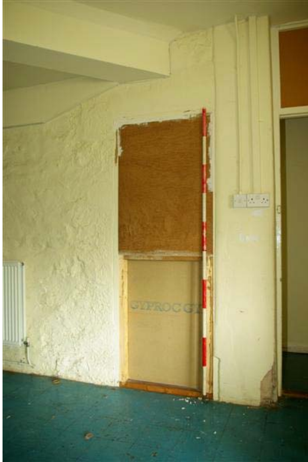
Plate 9: Blocked door between Rooms B1-5 and B1-7 (from Room B1-7 )
