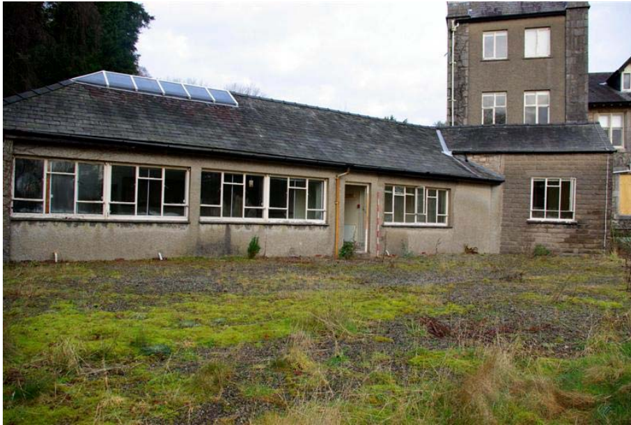
Plate 1: General view of Building 1, facing north
