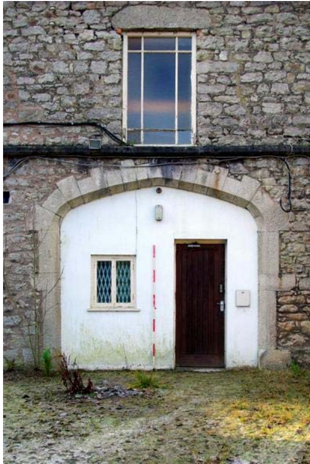
Plate 27: Main doorway, Building 3
