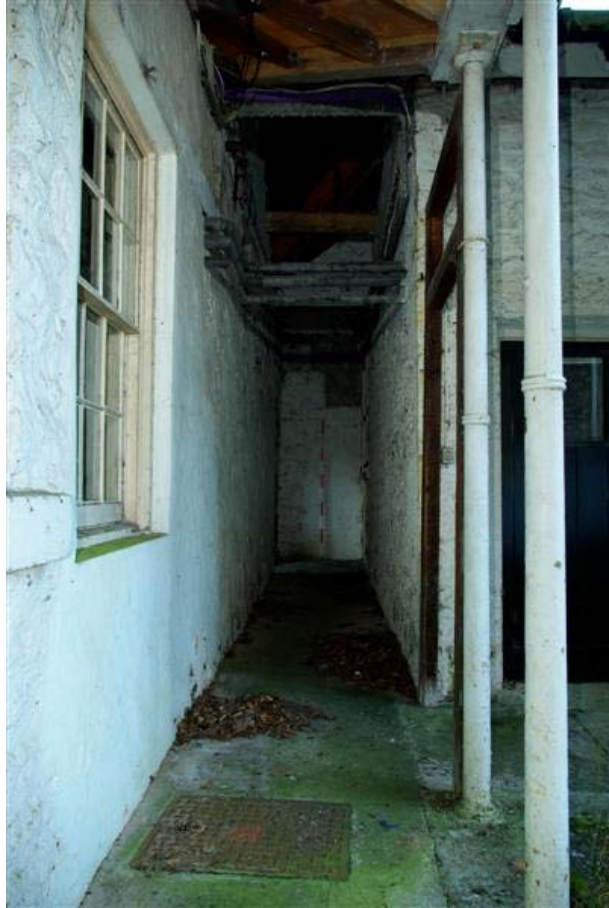
Plate 7: Walkway between Buildings 1 and 2
