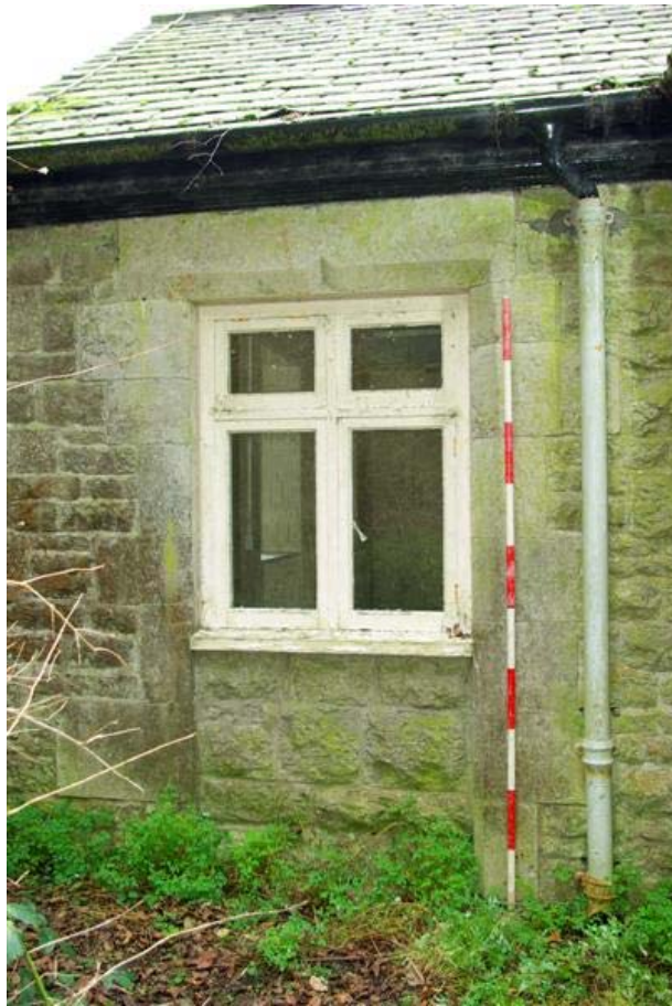
Plate 5: Partially blocked doorway on the south-west elevation of Building 1
