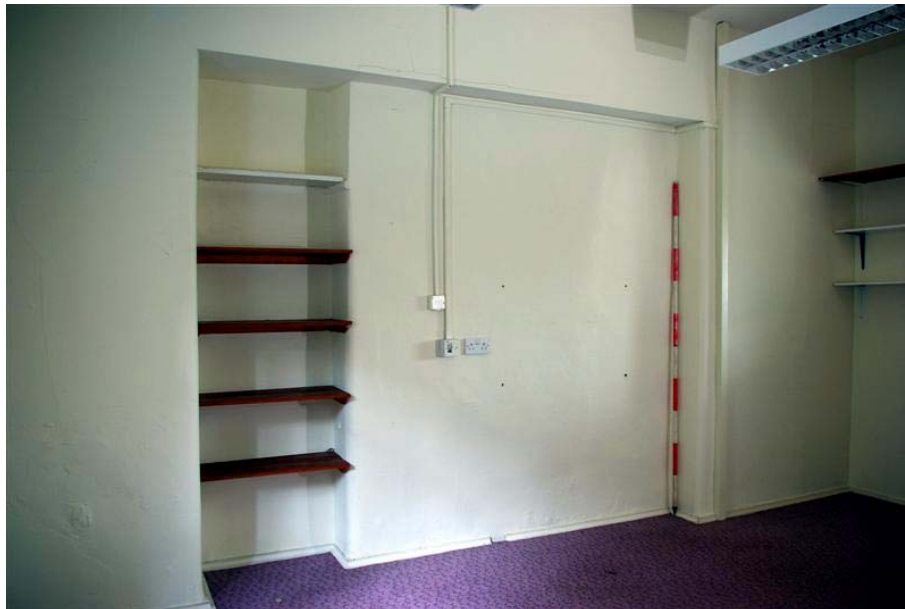
Plate 34: Recesses within Room B3-11 , Building 3
