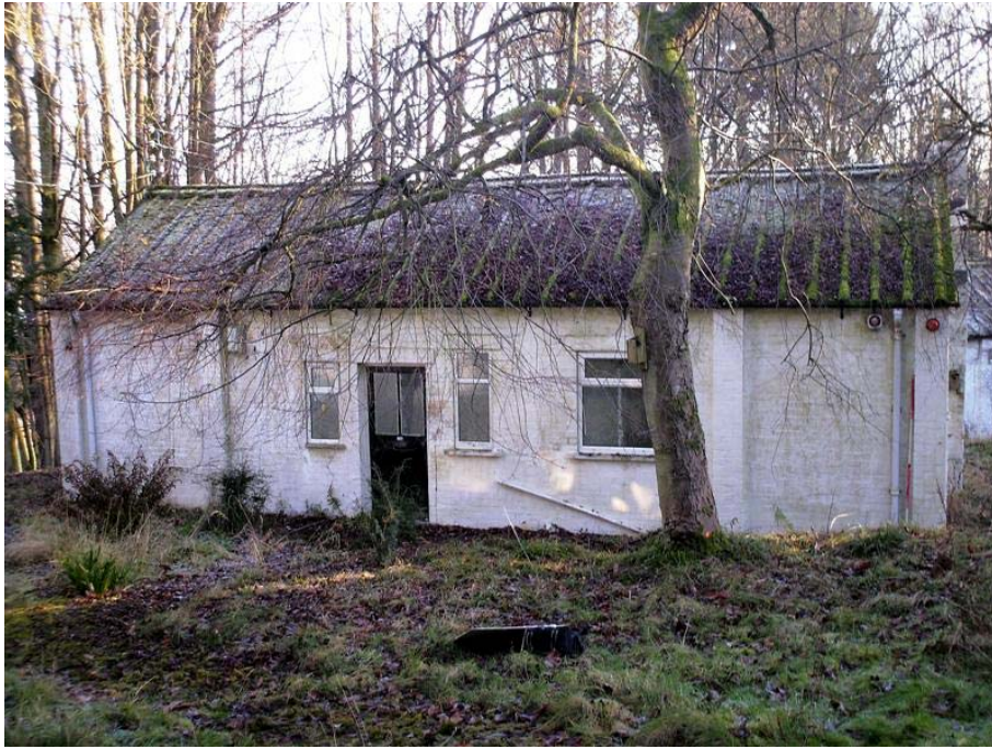
Plate 51: West elevation of Building 7
