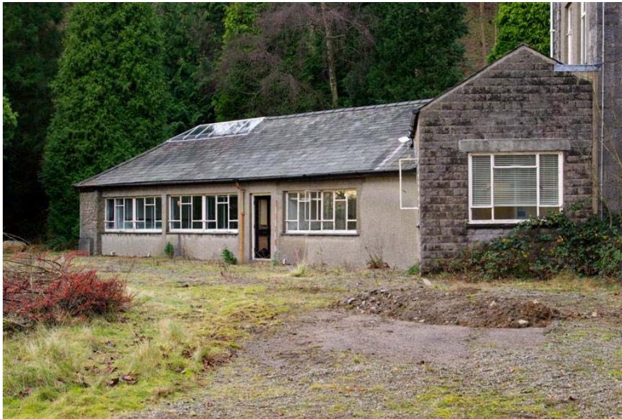
Plate 2: General view of Building 1, facing west
