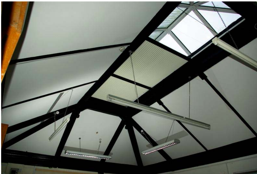
Plate 14: View of the roof in Room B1-9
