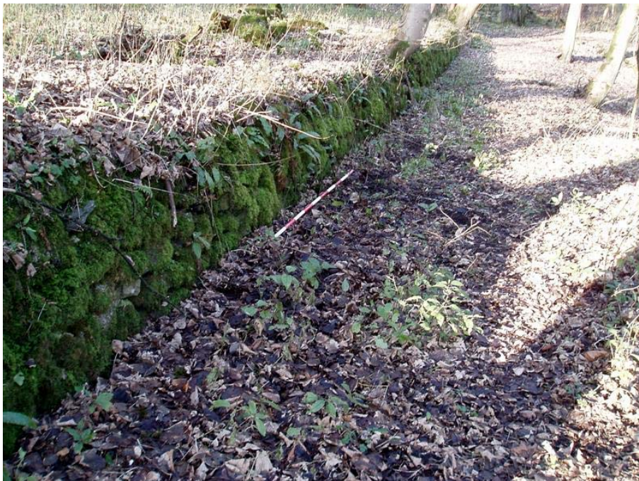
Plate 57: Revetment wall of the terrace looking north
