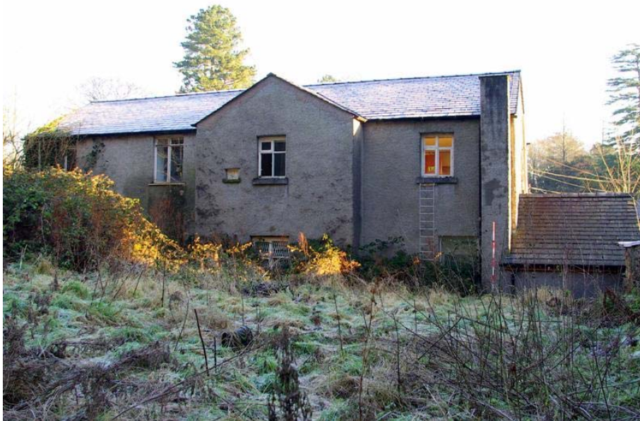
Plate 26: Rear view of Building 3, facing east
