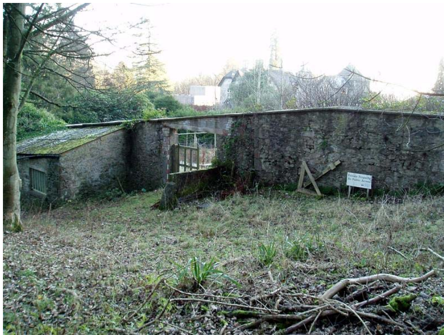
Plate 42: General view of the north wall of the walled garden, with lean-to building 4J to the left
