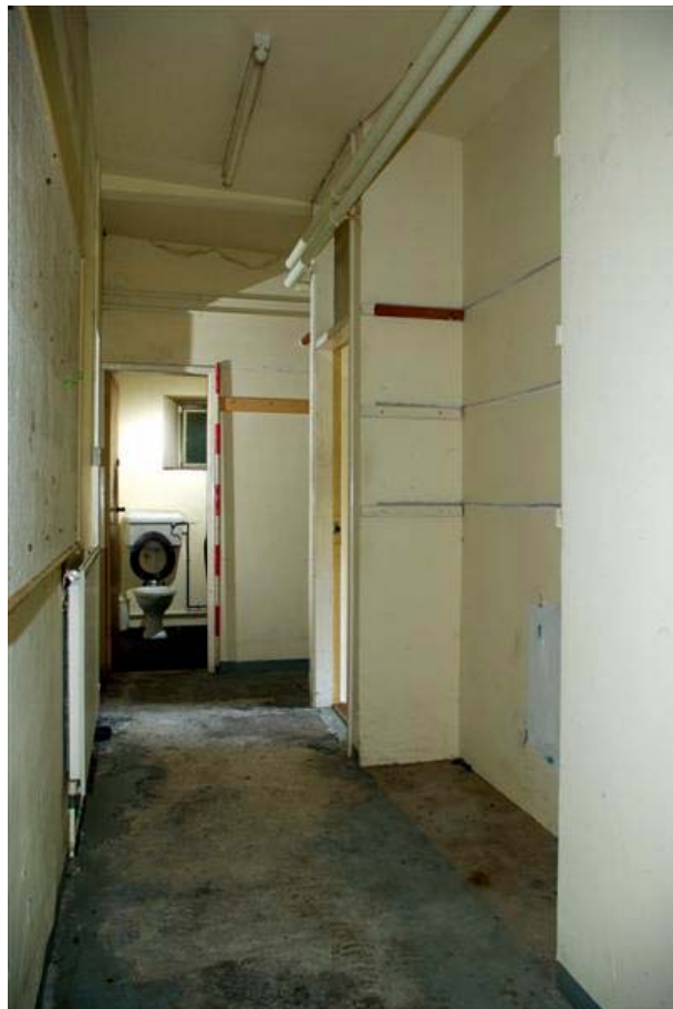
Plate 24: General view of Room B2-10 , facing west
