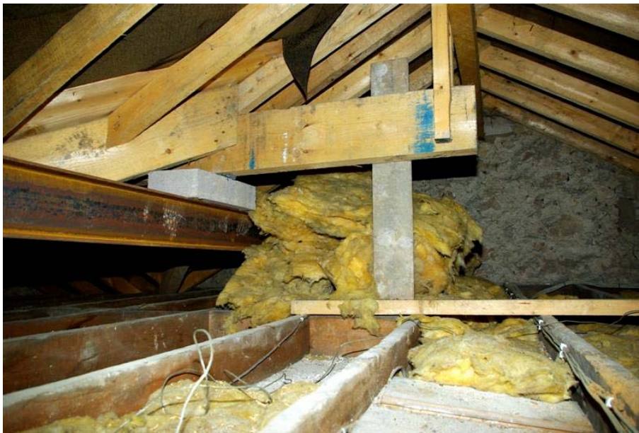
Plate 36: Roof space in Building 3
