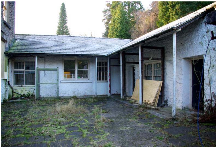
Plate 6: Courtyard between Buildings 1 and 2
