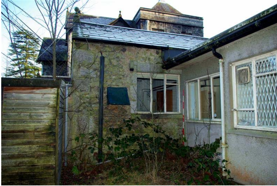
Plate 21: View of the west-facing elevation of the northern part of Building 2
