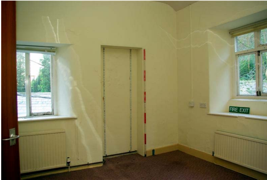
Plate 35: Room B3-12 in Building 3
