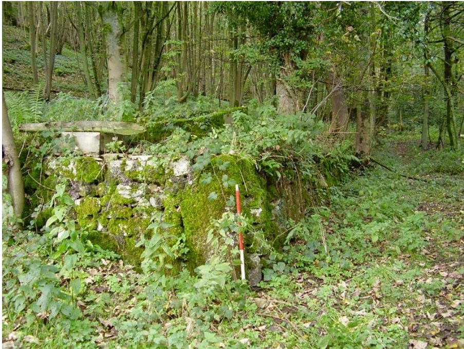
Plate 56: Revetment wall of the terrace looking north
