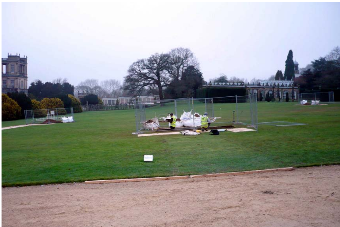
Plate 20: Trench 3 during excavation viewed towards the north. The surviving element of the terrace can be seen to the left of the Rose Garden marked by the large tree
