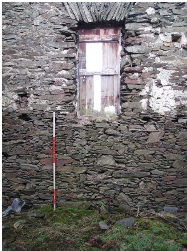
Plate 15: North-facing view of Room 4
