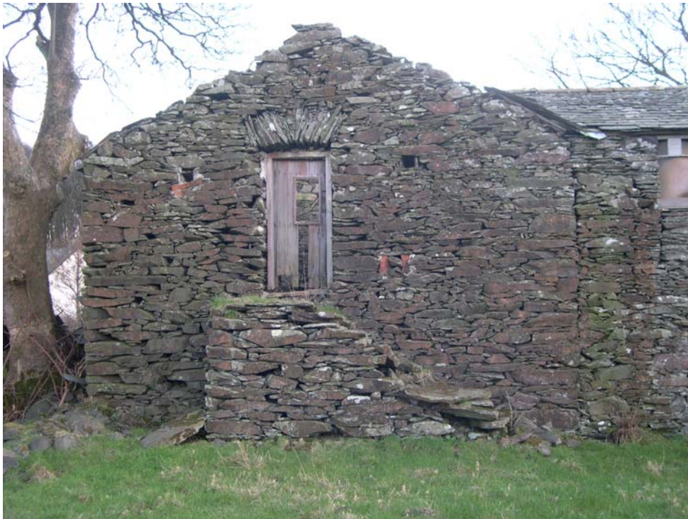
Plate 5: East end of Elevation 1
