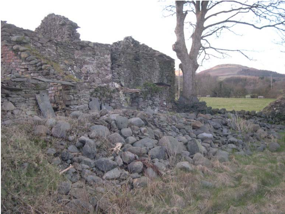
Plate 6: North-west-facing view of Elevation 3
