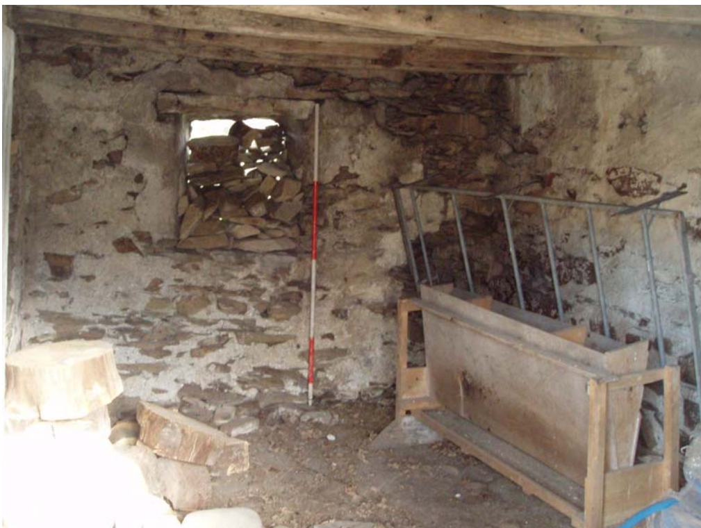
Plate 13: North-facing view of Room 2
