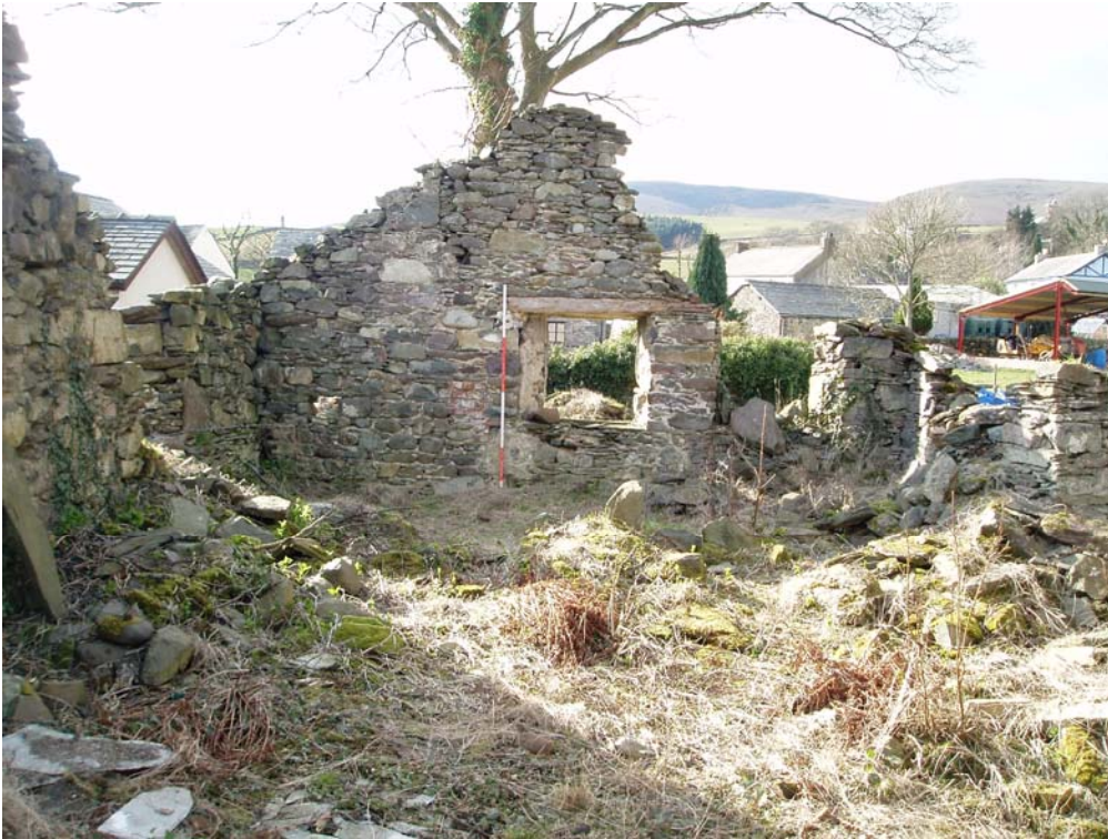
Plate 18: West-facing view of Room 7
