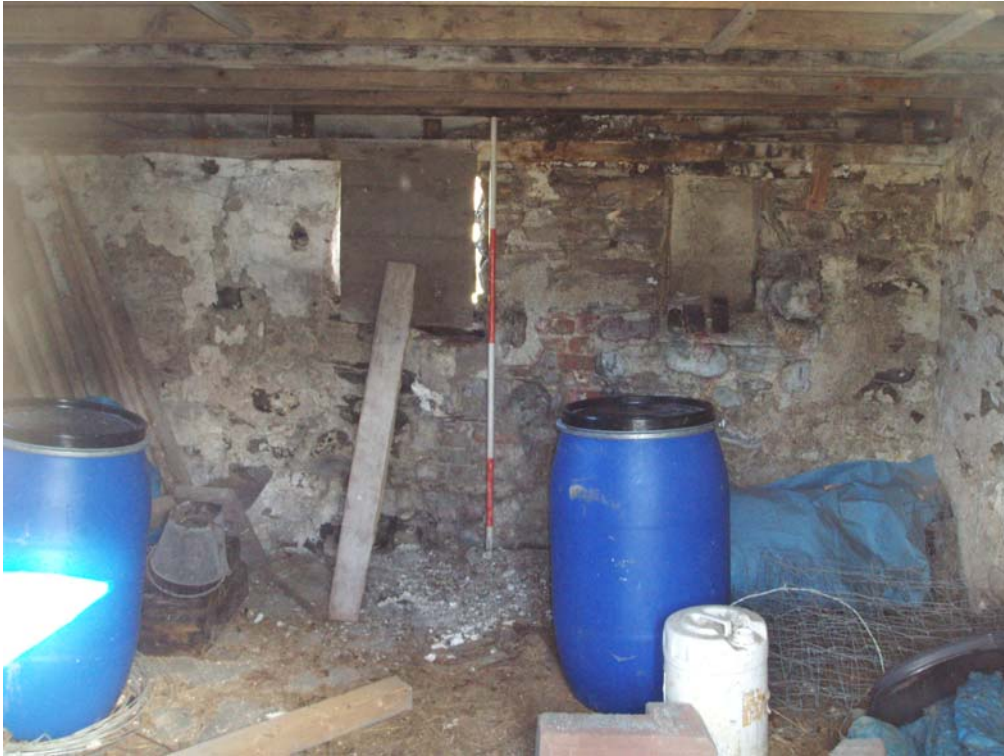
Plate 12: North-facing view of Room 1
