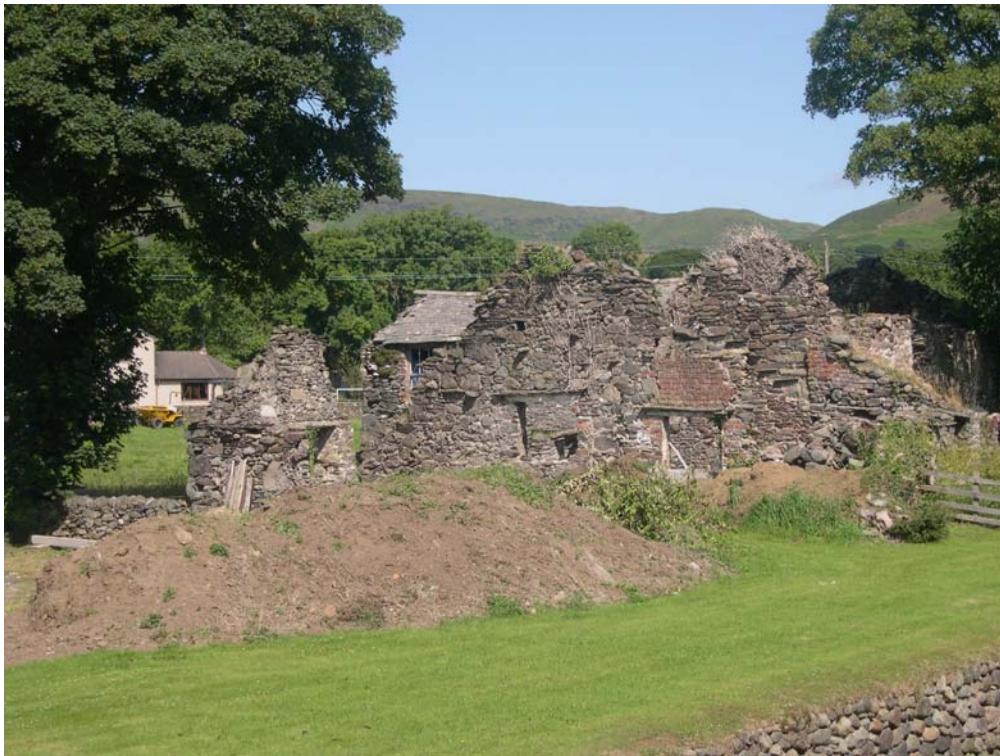
Plate 7: North-west-facing view of Elevation 4
