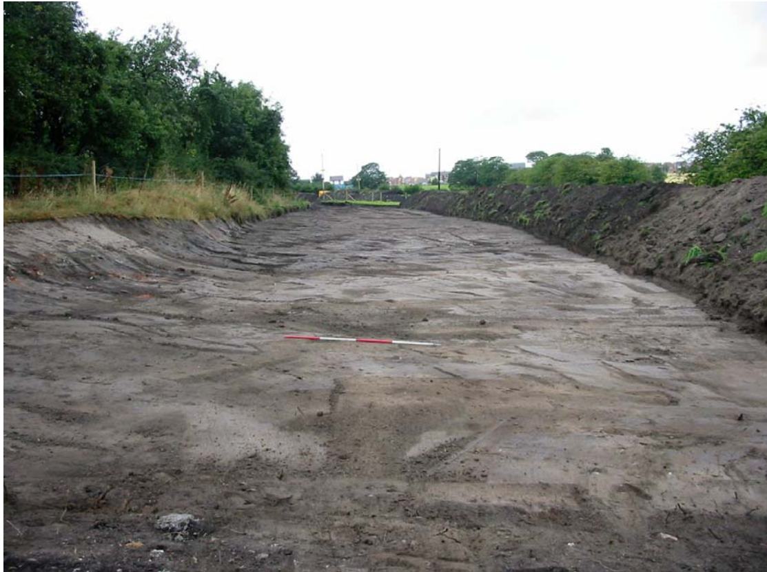
Plate 1: Northern end of Field 3 showing make-up layer 302 on the west side
