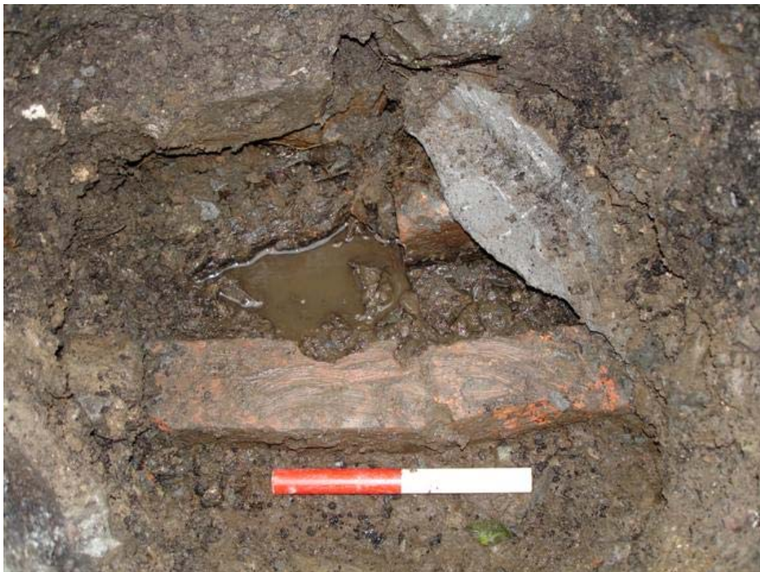
Plate 2: Exposed brick-lining to culvert 103
