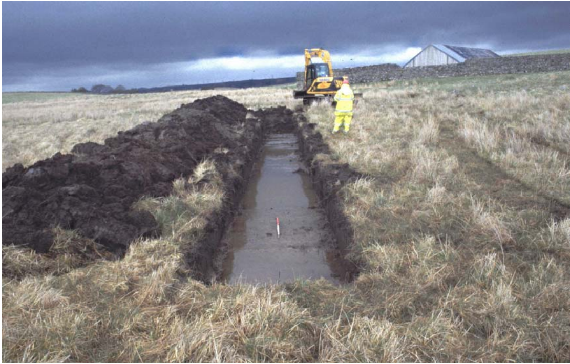
Plate 7: Trench 44 looking north-east
