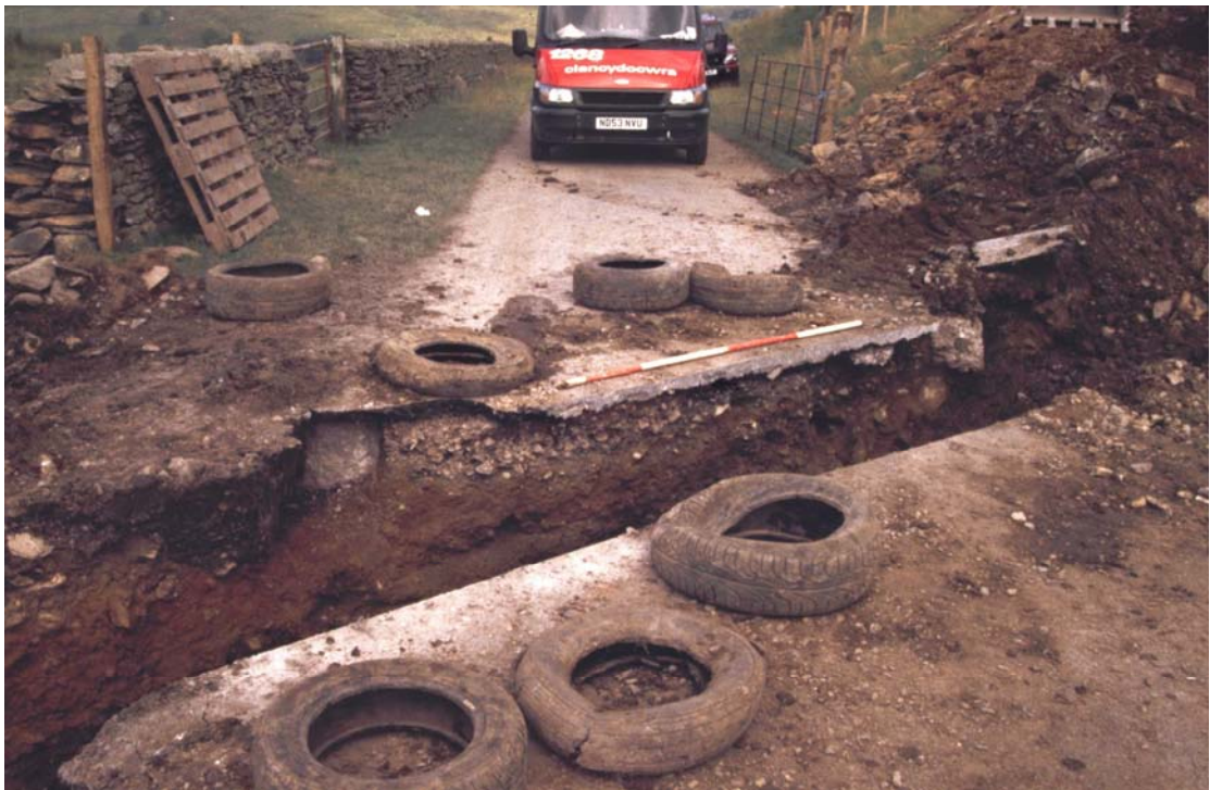
Plate 8: Section through the 1753 turnpike in Area B, looking south
