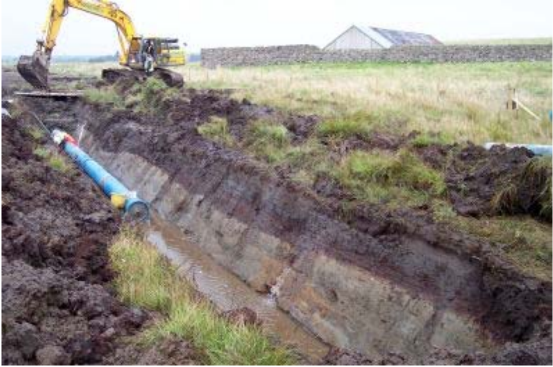
Plate 9: Laying the pipeline during the watching brief in Area E
