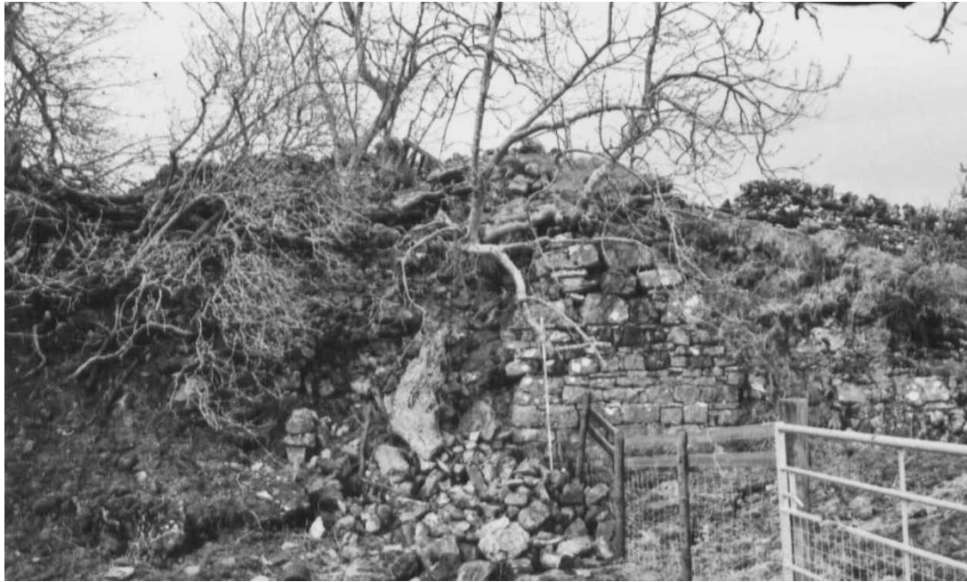
Plate 3: South elevation of lime kiln (Site 34)
