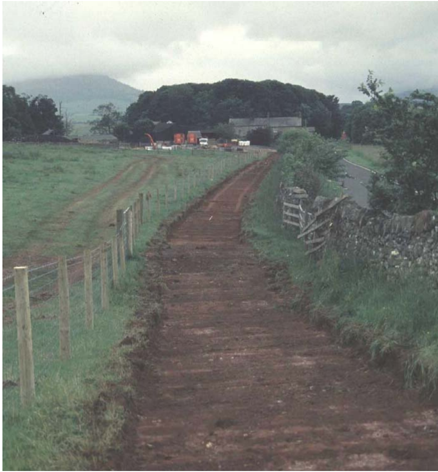
Plate 9: Topsoil stripping at Highgate Farm Access Track
