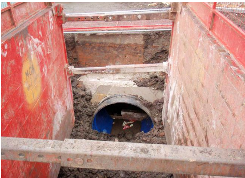
Plate 3: MH-4 with new pipe, looking north-east
