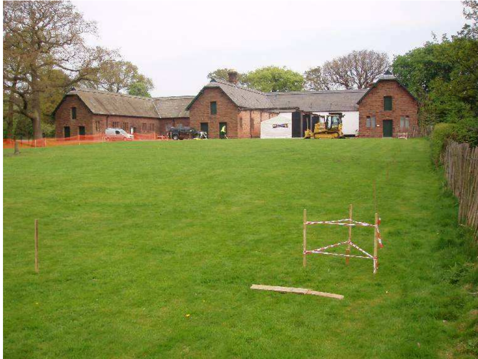
Plate 3: View of the maze site prior to ground works, looking north
