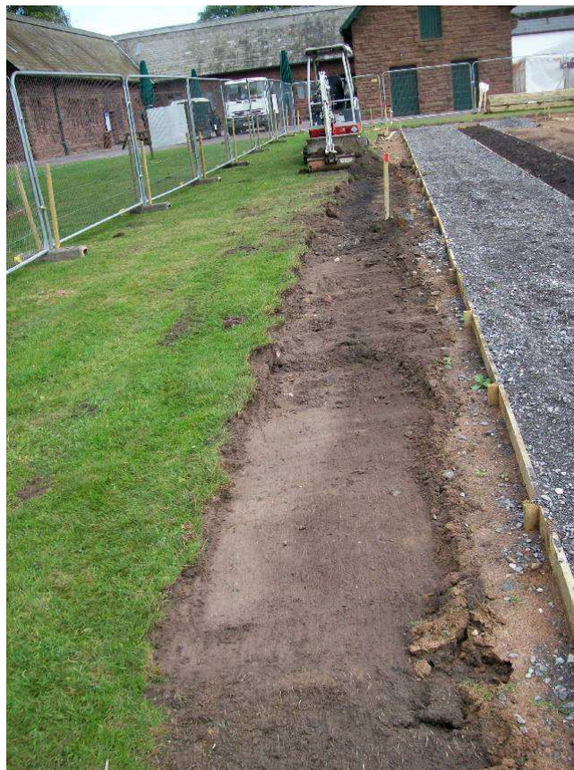
Plate 10: Area of turf stripping at the western side of the site
