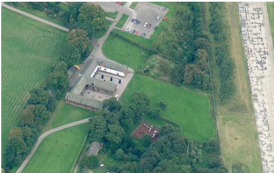
Plate 2: Oblique aerial view of the maze site, facing east
