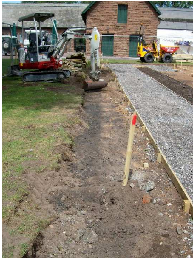
Plate 11: Fuel ash revealed at the western side of the site
