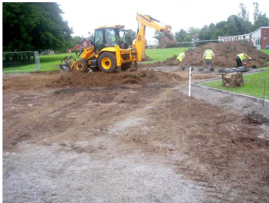
Plate 11: Area stripped during watching-brief on 9 th August 2010, looking north
