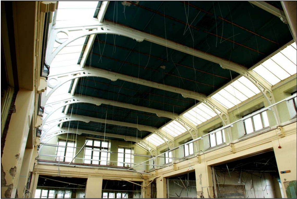
Plate 40: The roof structure in the main hall after stripping
