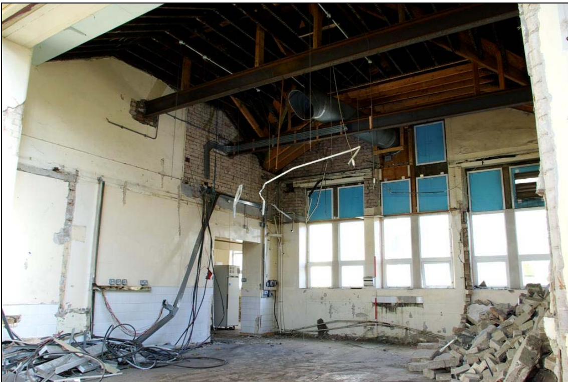
Plate 27: The kitchens (Room JS-C) following soft stripping
