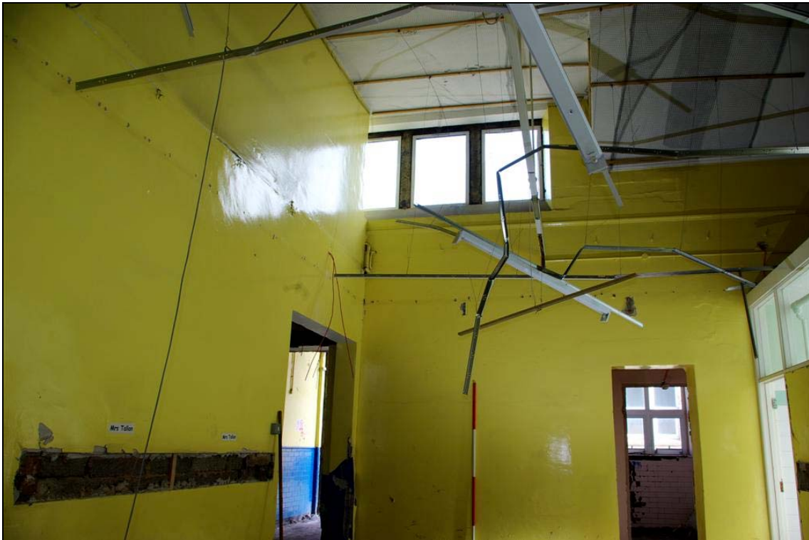
Plate 29: Fenestration revealed above Rooms 71 and 78 (JS-D)
