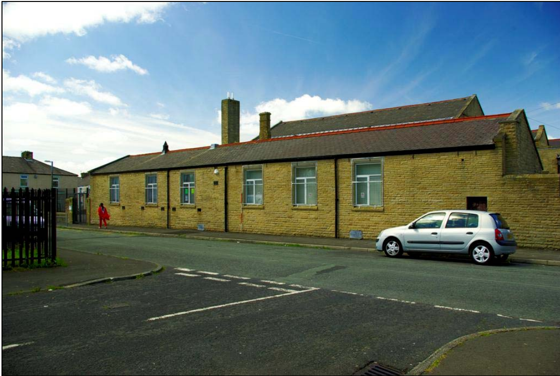
Plate 62: South elevation of the Science Building
