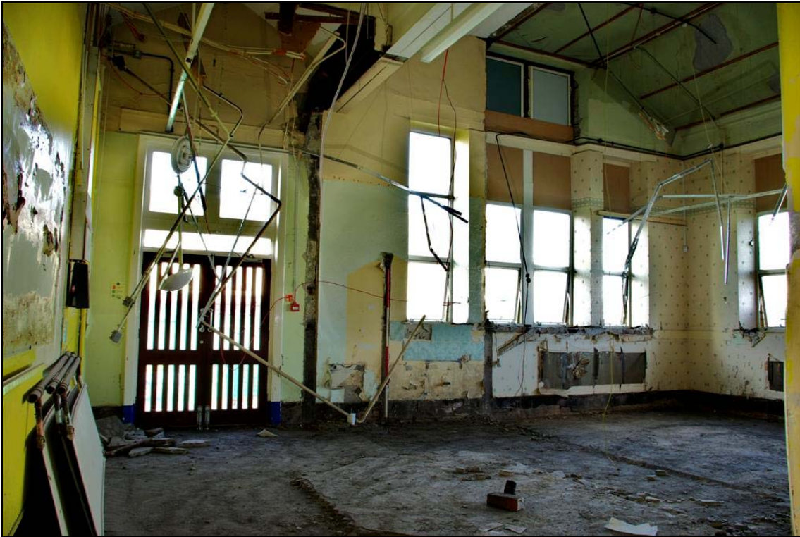
Plate 18: Rooms 46-52 following stripping
