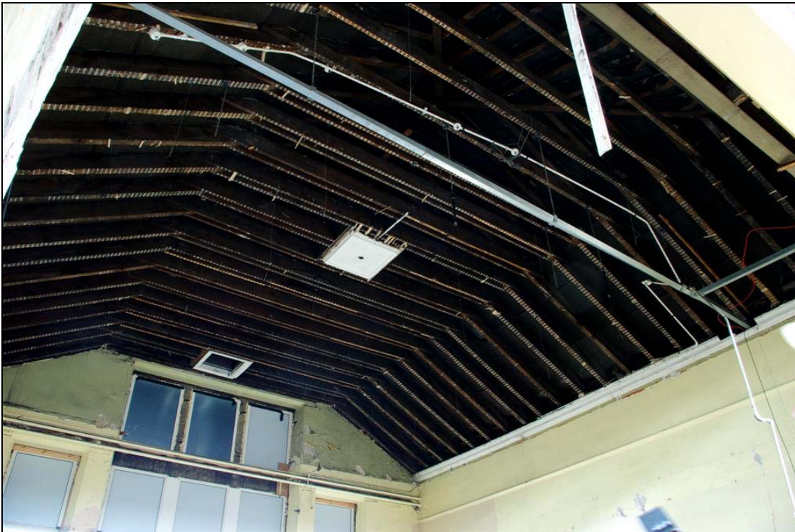
Plate 23: Example of a classroom ceiling following soft strip
