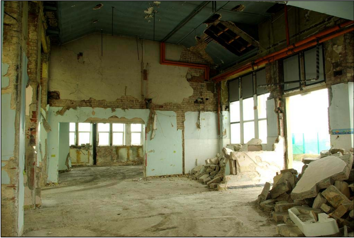
Plate 50: Rooms 17-21 (Room IS-A) following stripping
