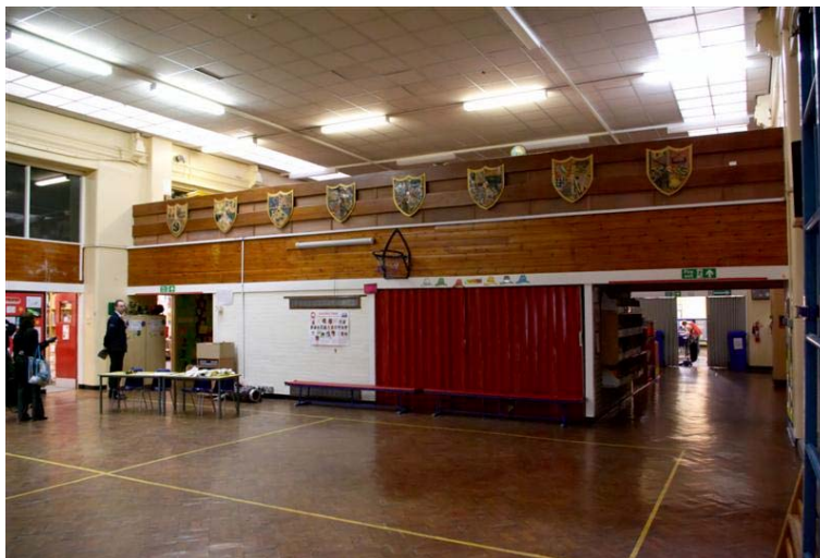
Plate 3 Mezzanine to be removed in the main hall of the senior school
