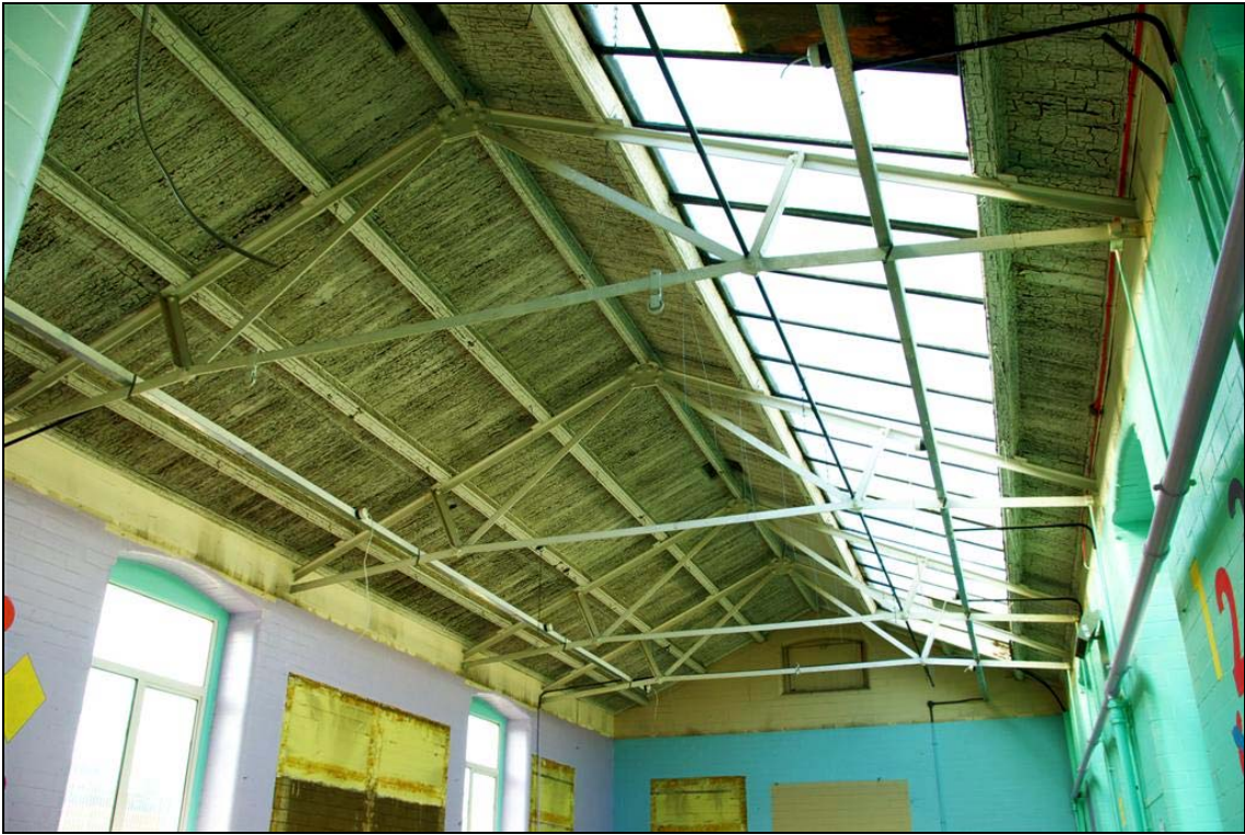
Plate 66: Roof trusses in Room 60 in the Science Building
