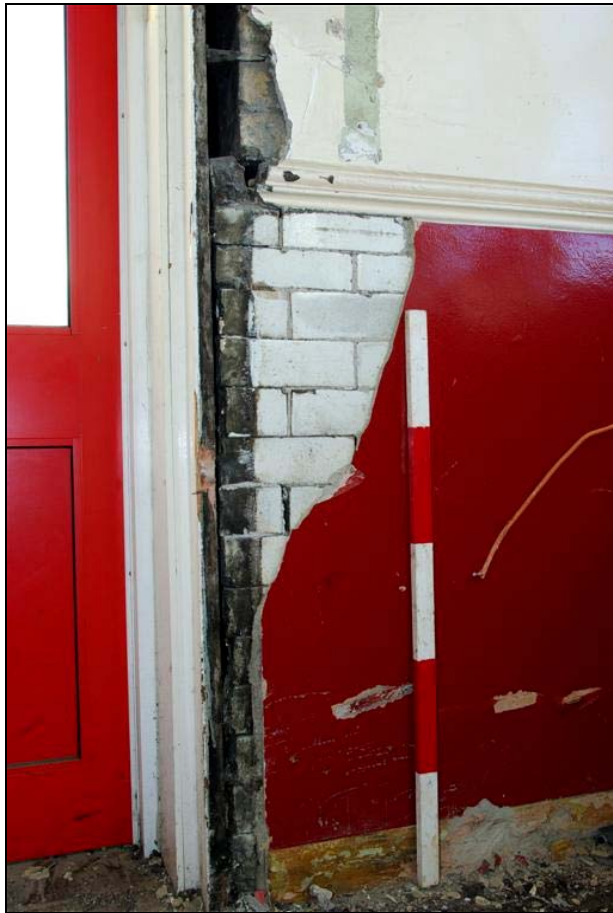
Plate 32: Dado panel in Room 83 (JS-E) following the soft strip
