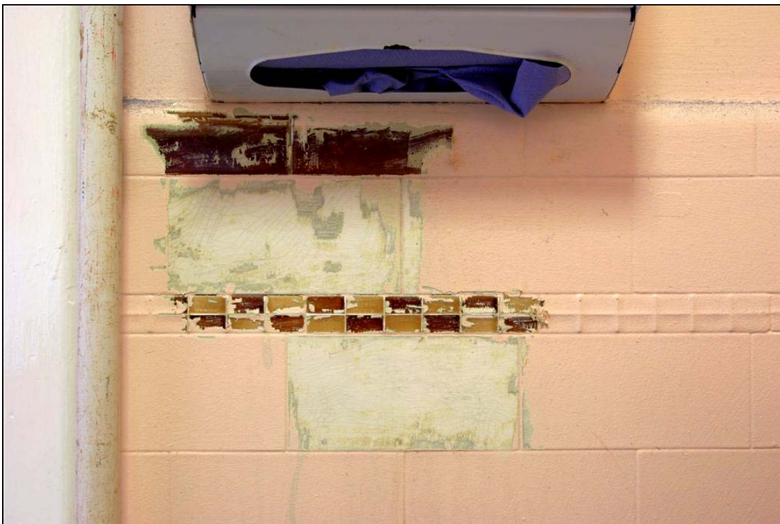
Plate 61: Decorative tiles in Rooms 35 and 36
