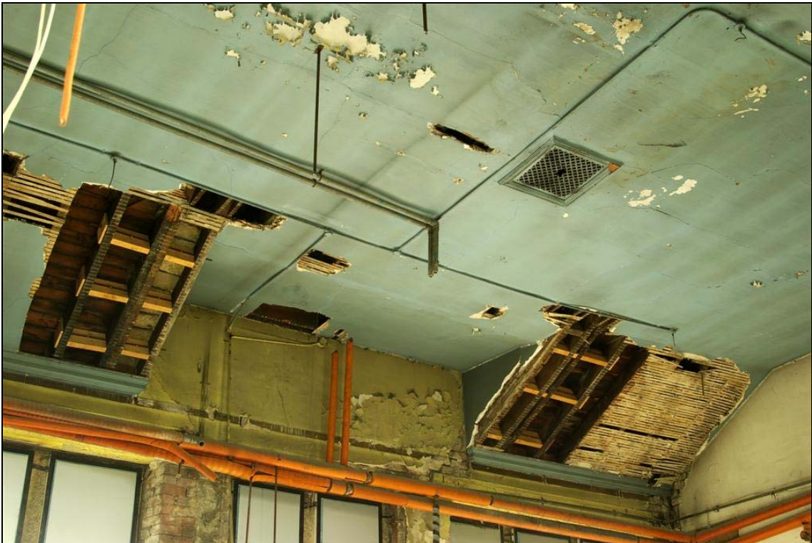
Plate 51: The ceiling in Room IS-A following stripping
