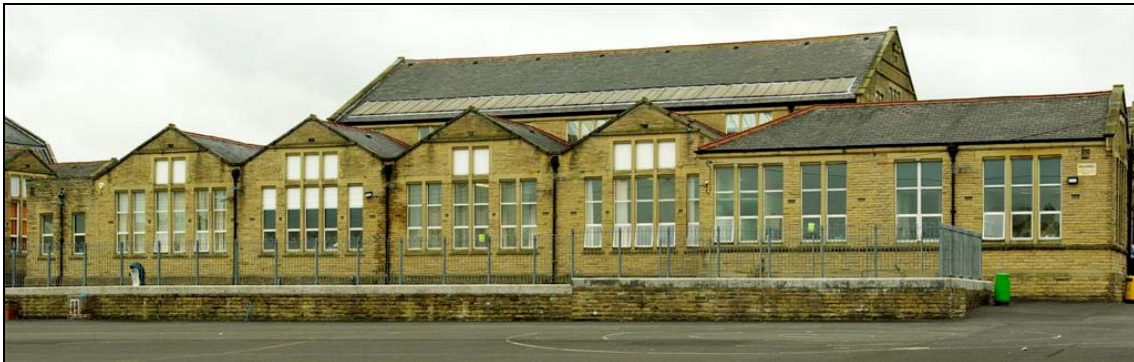
Plate 8: View of the north elevation showing the relationship between the classrooms and the main hall
