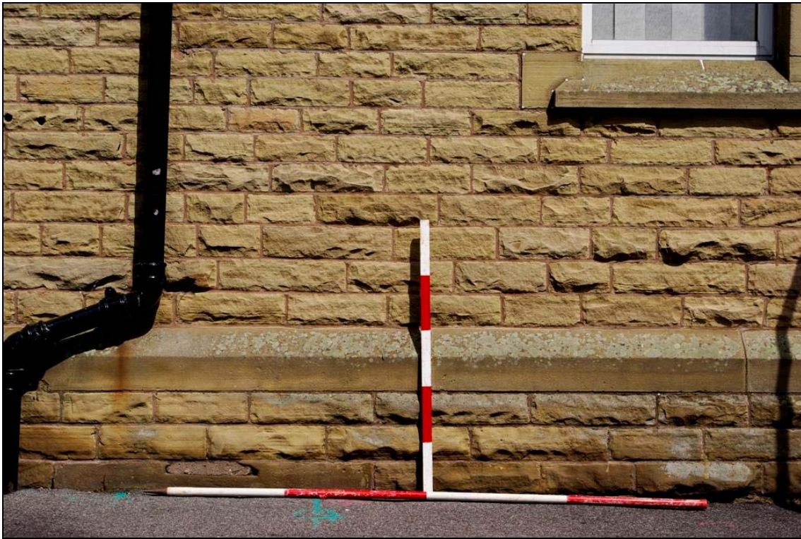
Plate 7: Construction details of the exterior fabric of the Junior and Infant Schools
