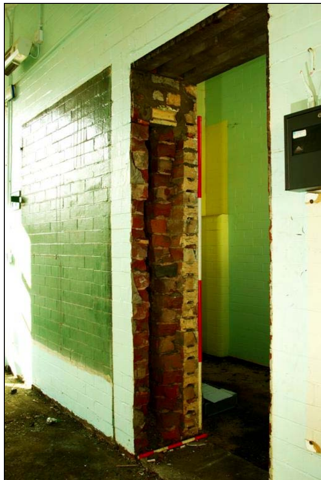
Plate 63: Doorway between Rooms 99 and 100 in the Science Building
