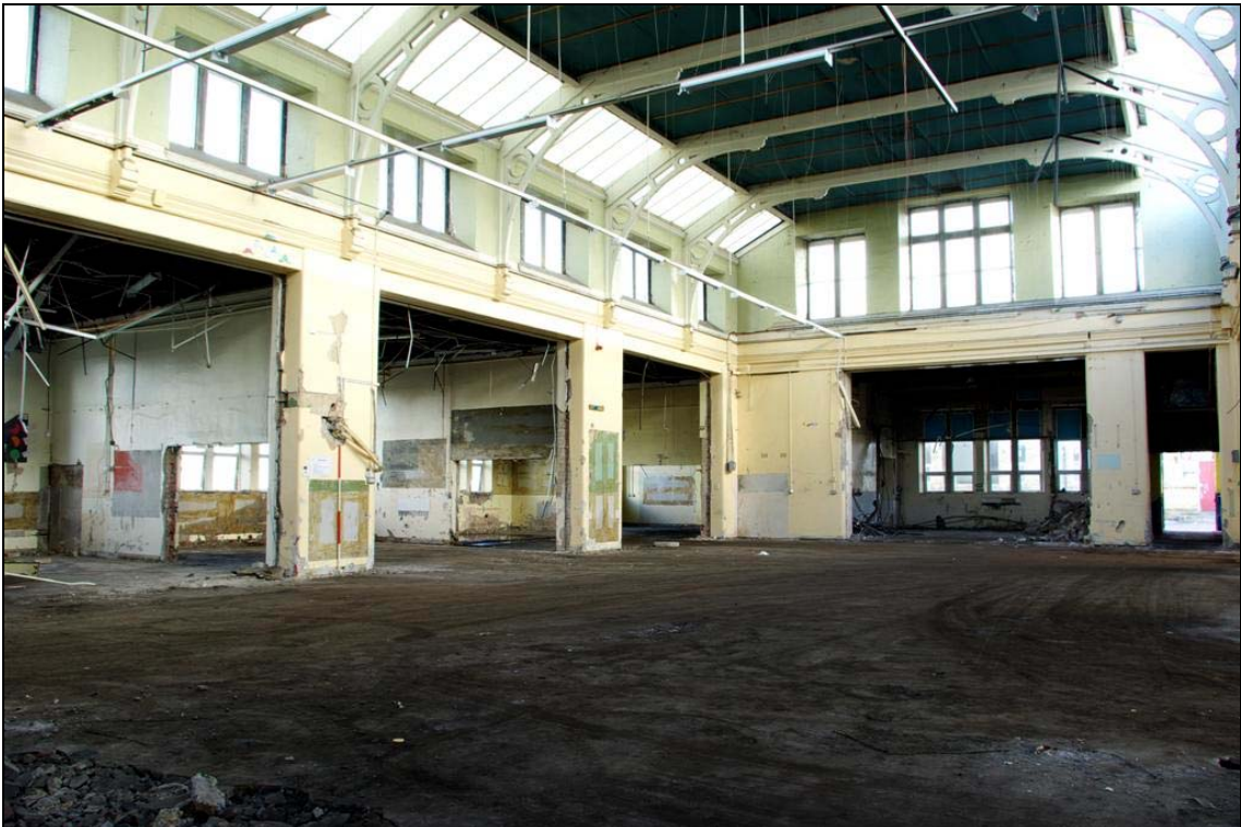
Plate 39: View of the main hall after stripping (facing north-west)
