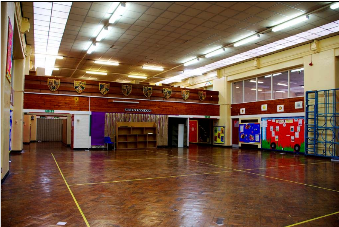
Plate 35: View of the main hall in the Junior School prior to stripping (facing north-west)
