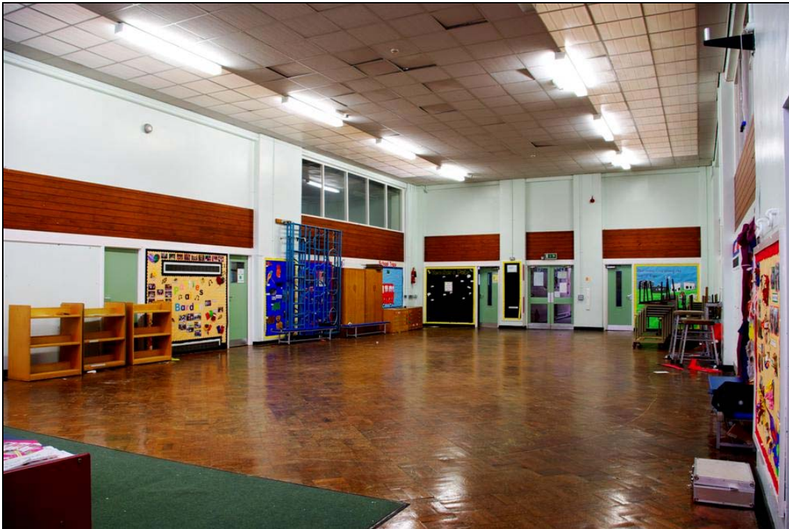
Plate 54: General view of the main hall (Room 29) in the Infants School (facing south) prior to stripping
