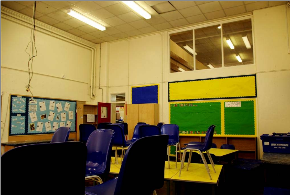
Plate 20: Room 58 prior to strip
