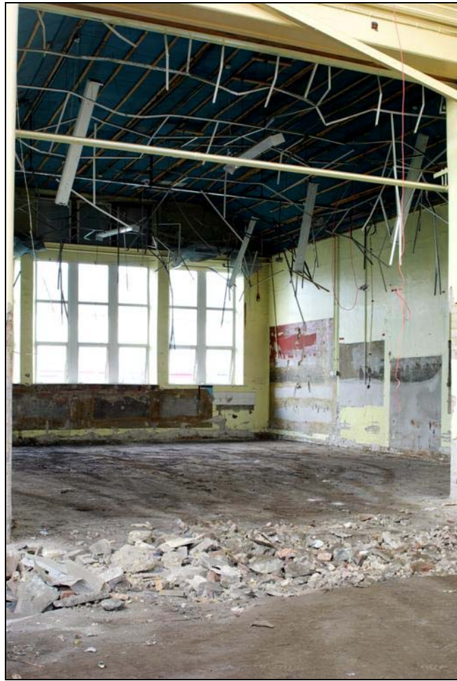
Plate 22: Example of a classroom following soft strip
