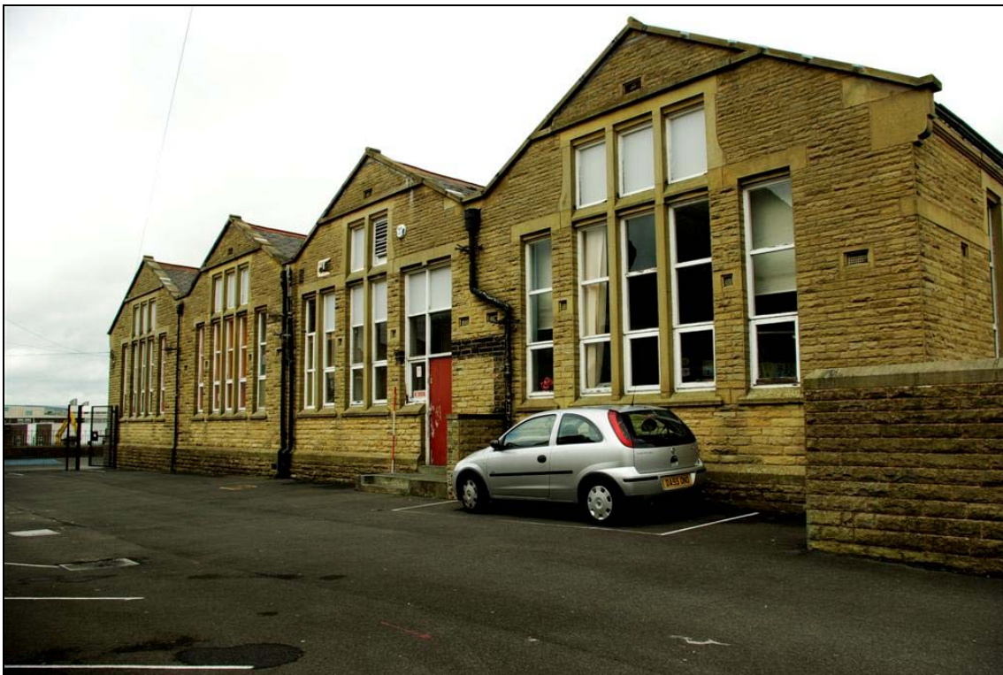
Plate 47: General view of the west elevation of the Infant School
