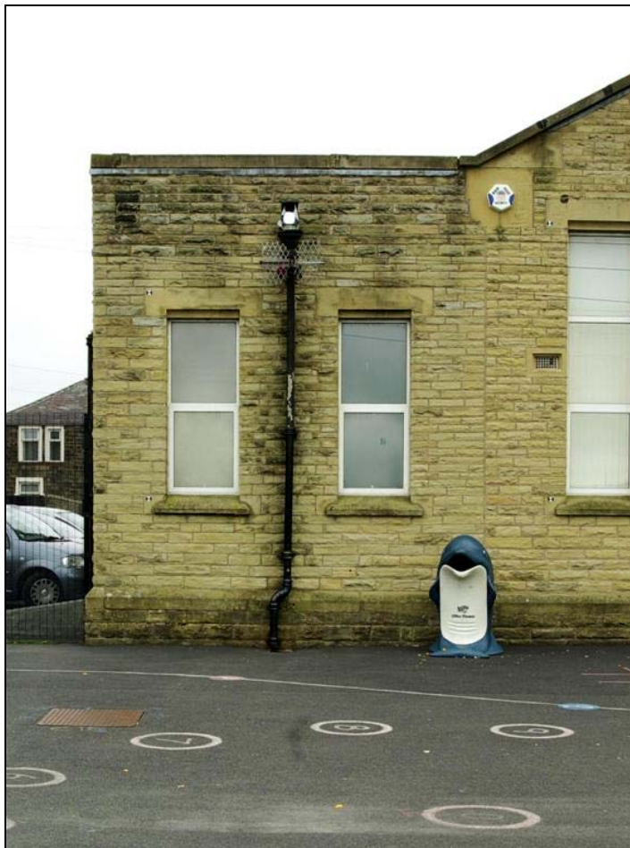
Plate 13: East side of the north elevation of the Junior School showing butt-join
