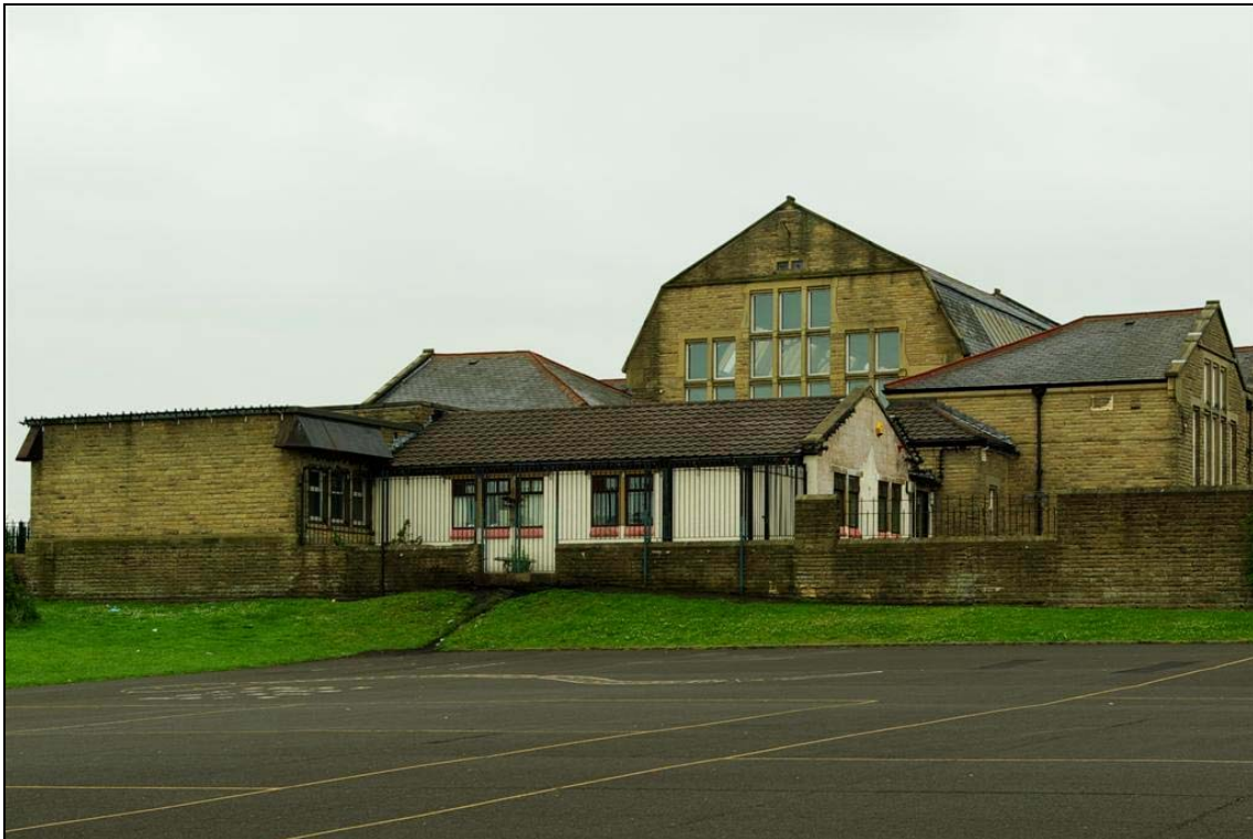
Plate 48: General view of the north elevation of the Infant School
