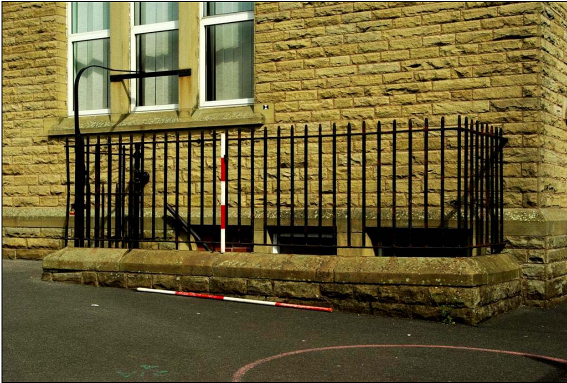
Plate 46: Steps down to basement on the principal elevation of the Infant School
