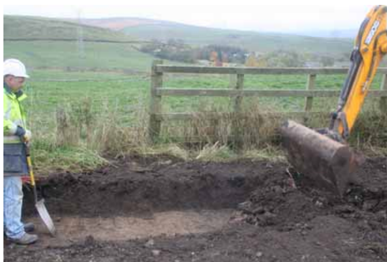
Plate 1: mechanical removal of topsoil under archaeological supervision during construction of the switchgear house at the western end of the pipeline
