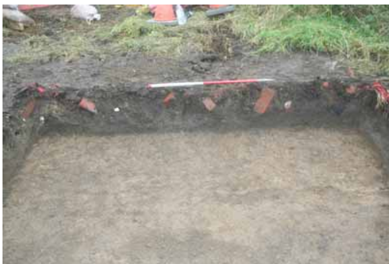
Plate 2: modern topsoil and a buried soil overlying natural clay, observed during ground works for the construction of the switchgear house
