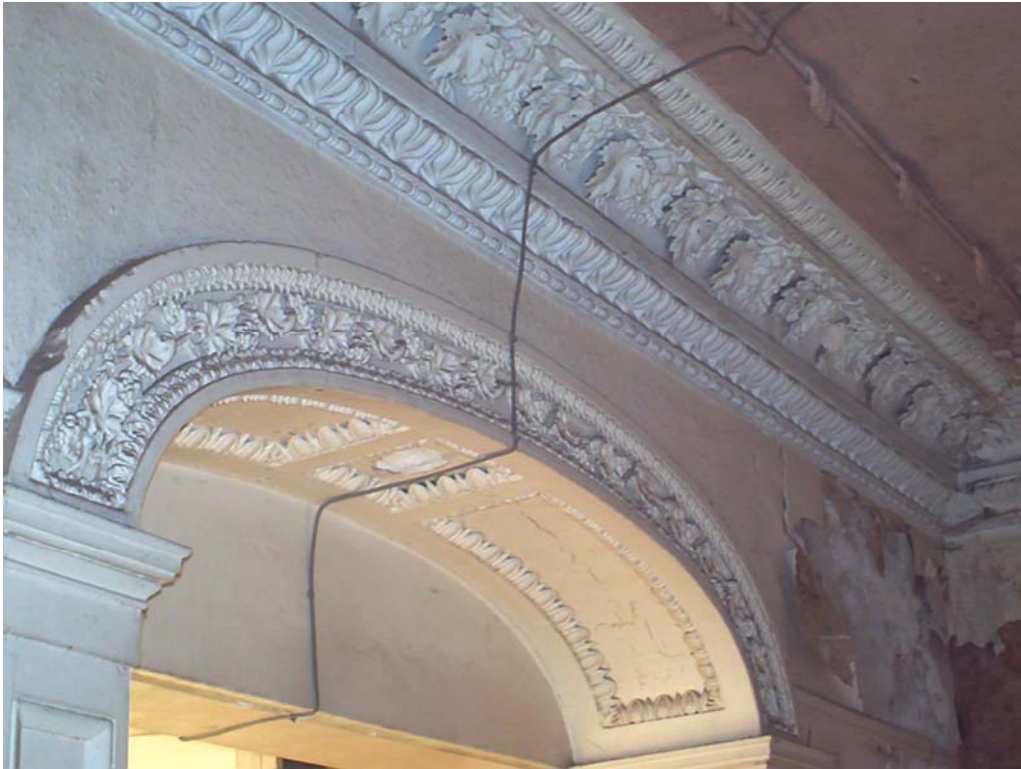
Plate 7: Detail of the segmental arch and cornice in room 5
