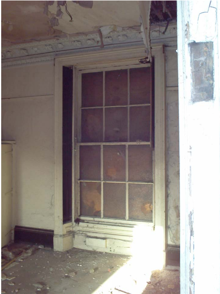
Plate 13: The sash window within room 5
