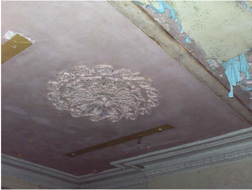
Plate 9: The ceiling rose in room 2, with the scar of the former partition to the right of the frame
