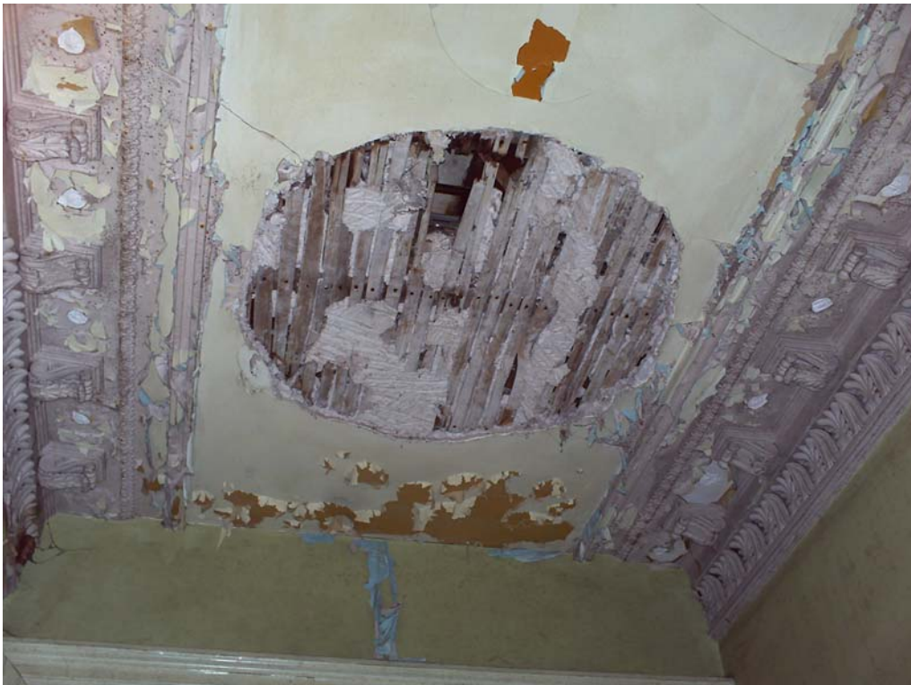
Plate 12: The scar of the former ceiling rose within room 1
