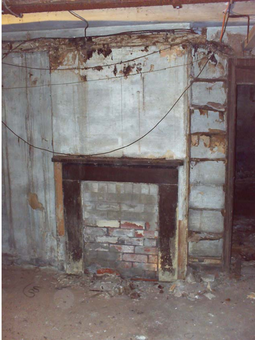
Plate 16: Detail of the fireplace within room 10
