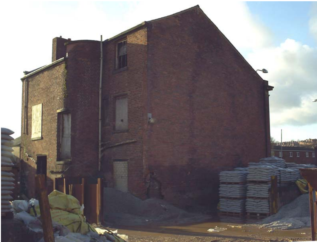
Plate 3: The east elevation
