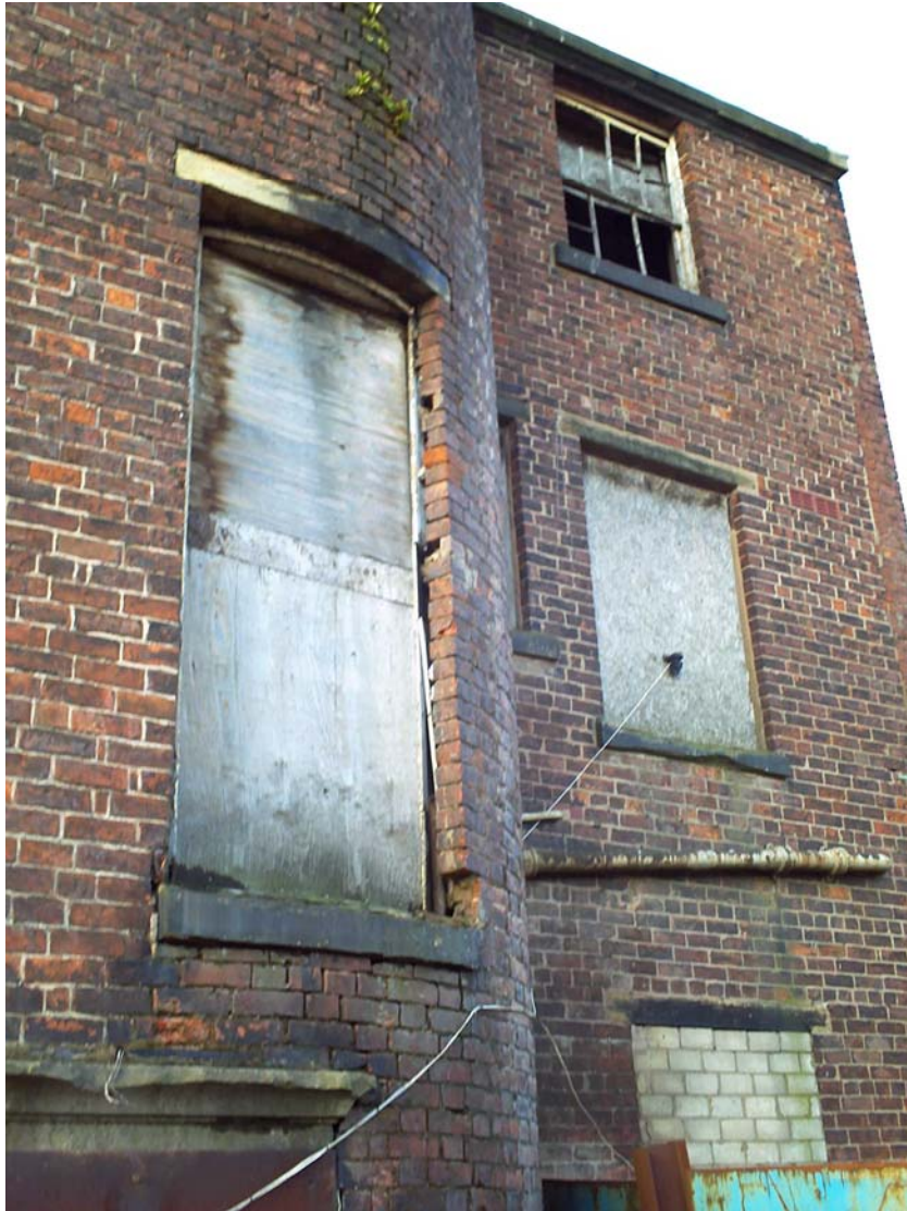
Plate 6: The blocked windows on the rear (south) of the building
