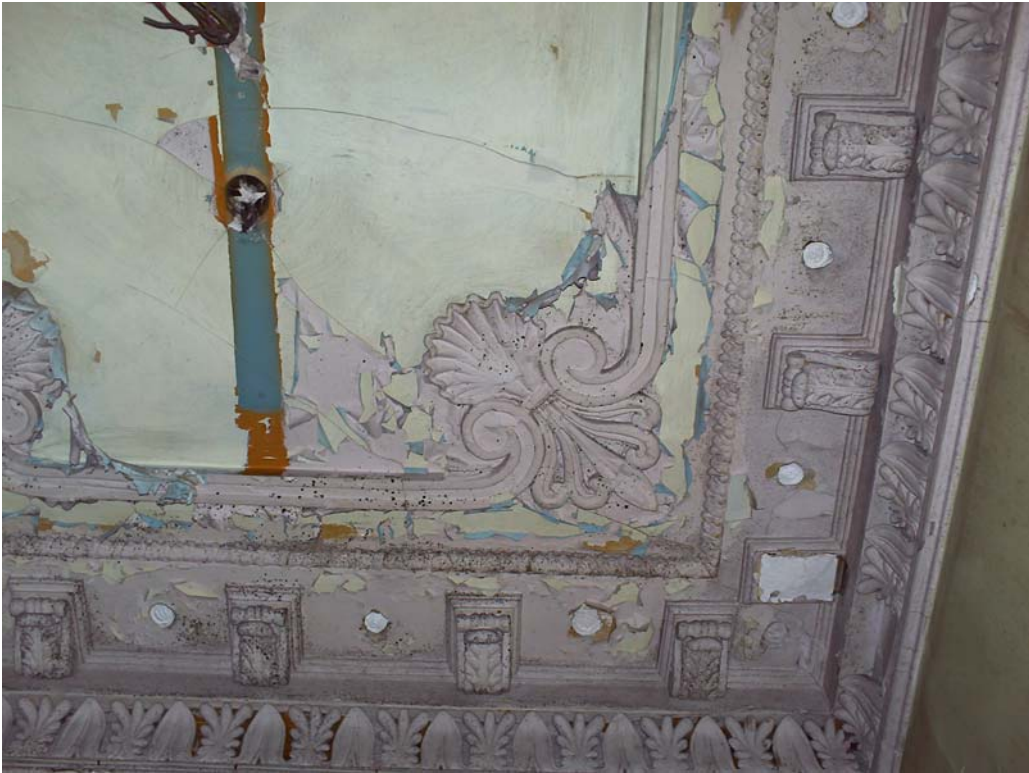
Plate 11: Further detail of the mouldings within the hallway (room 1 )
