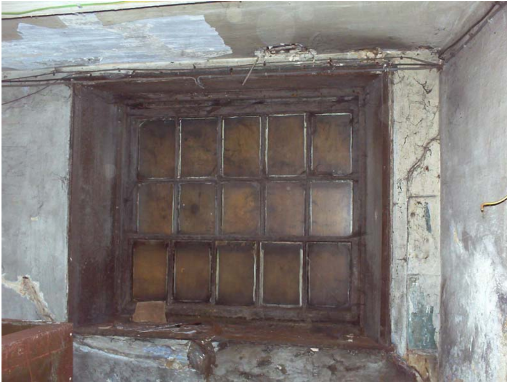
Plate 14: Detail of the cellar-lights in room 10
