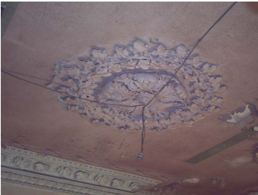
Plate 8: Detail of the ceiling rose in room 5
