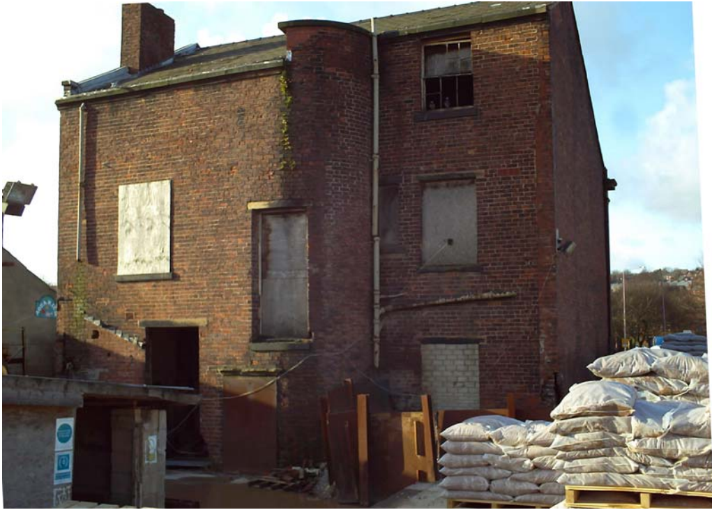
Plate 2: The rear (south) elevation of 53 King Street
