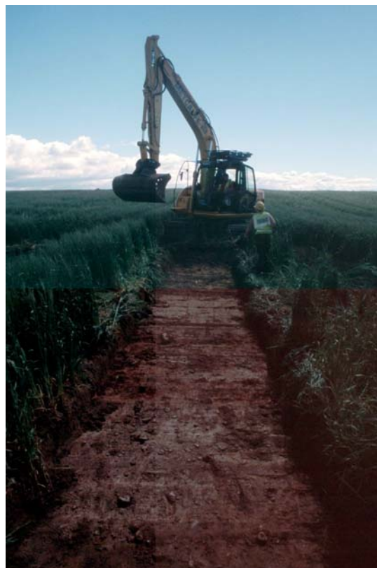
Plate 4: Working shot machining Trench 56
