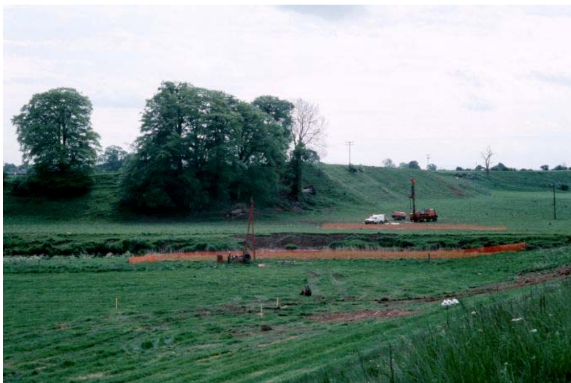
Plate 2: Working Shot, looking north-west across the River Eden
