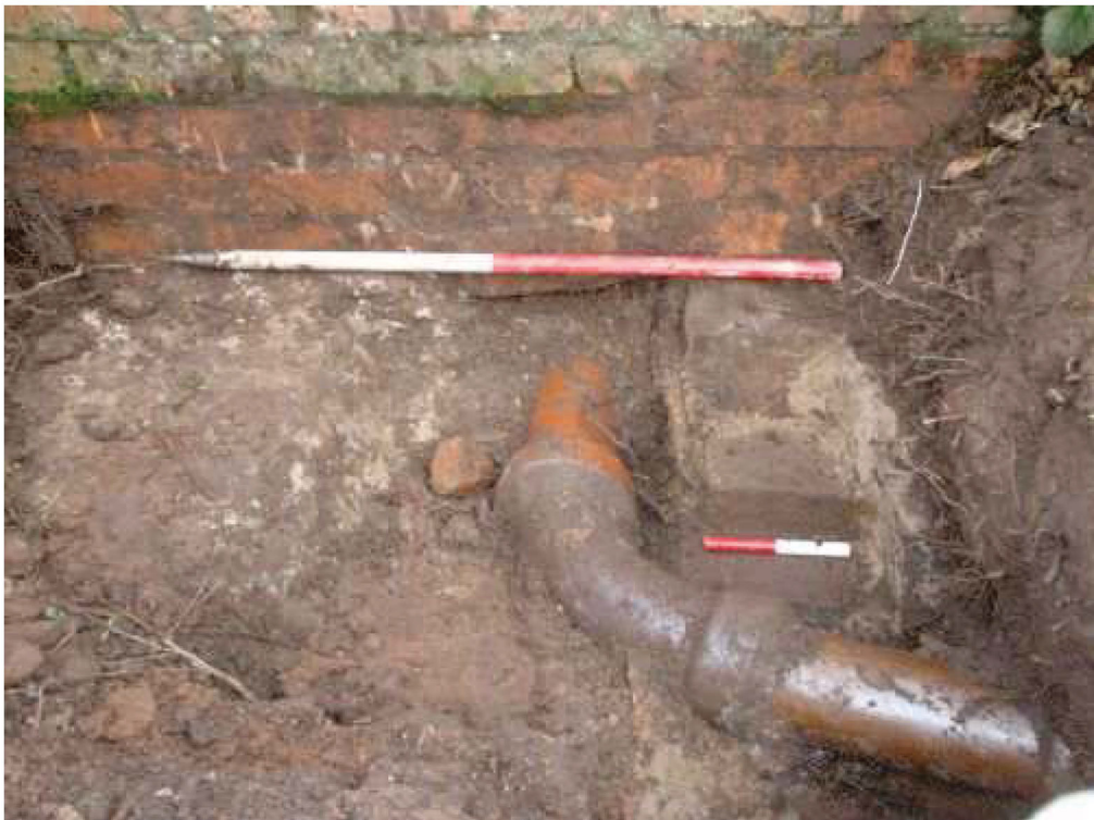
Plate 8: Test pit D showing the steps and sewage pipe, looking north
