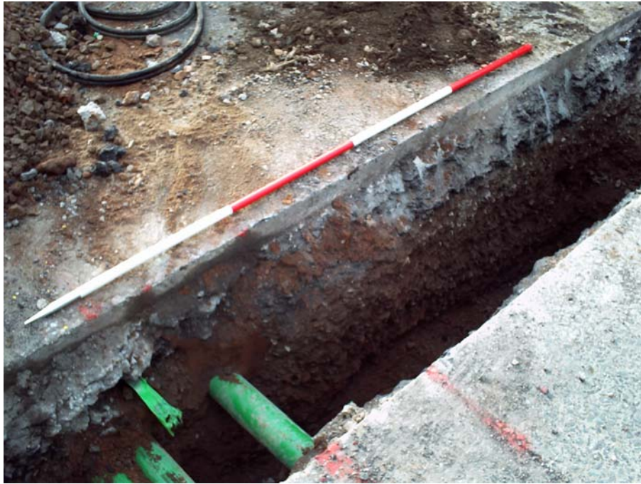
Plate 2: The north-facing section of the trial trench
