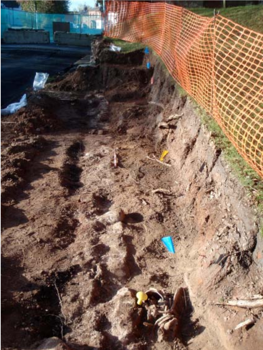
Plate 5: Foundations of the levelled churchyard wall and the battered-back churchyard deposits, revealing a charnel deposit in the foreground
