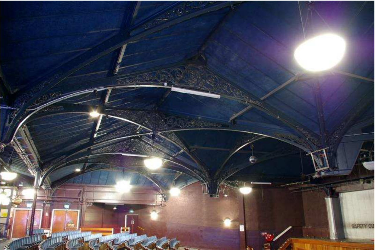
Plate 16: View of the cast-iron roof structure in the auditorium
