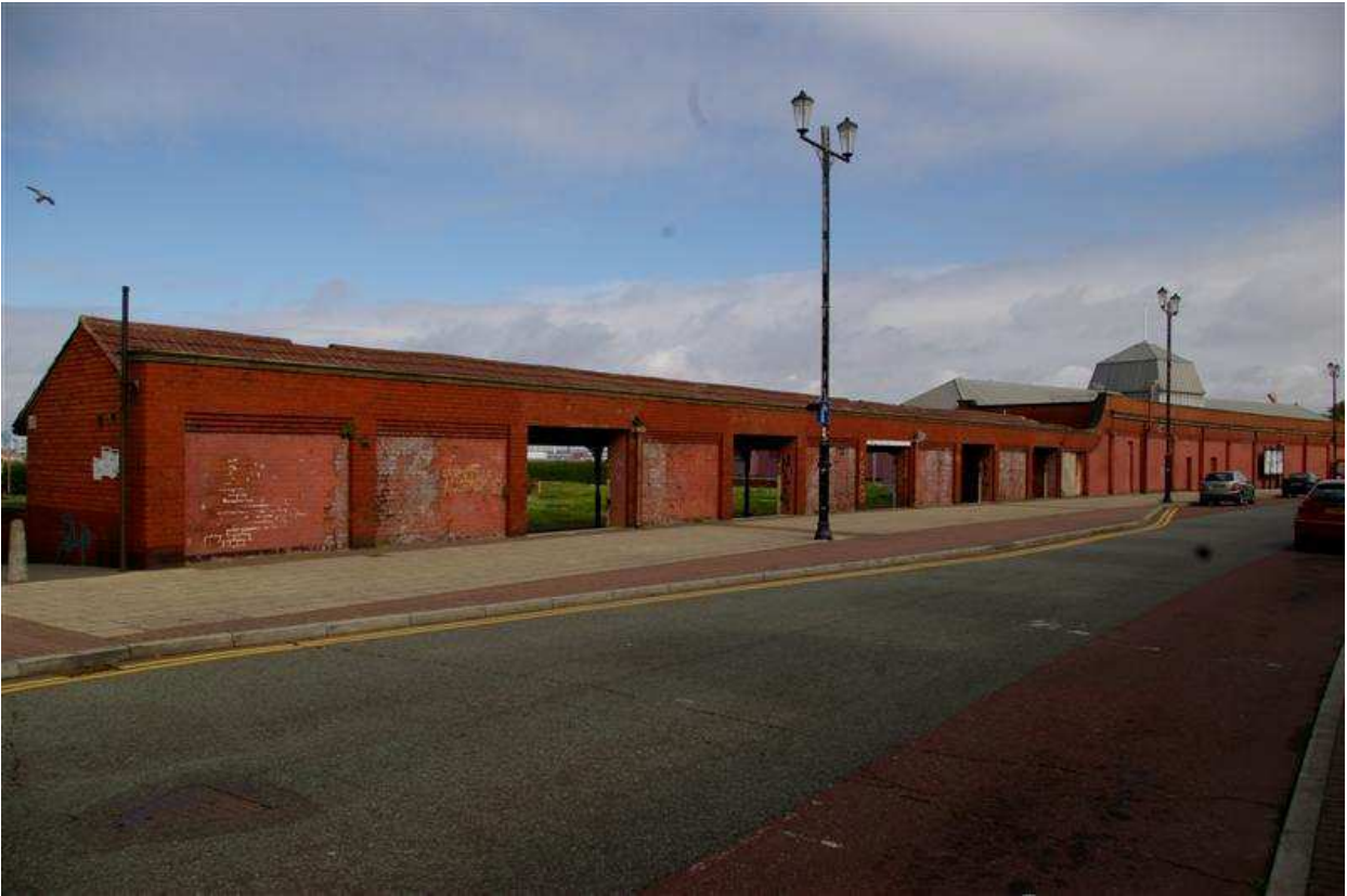
Plate 10: Covered arcade attached to the west of the building
