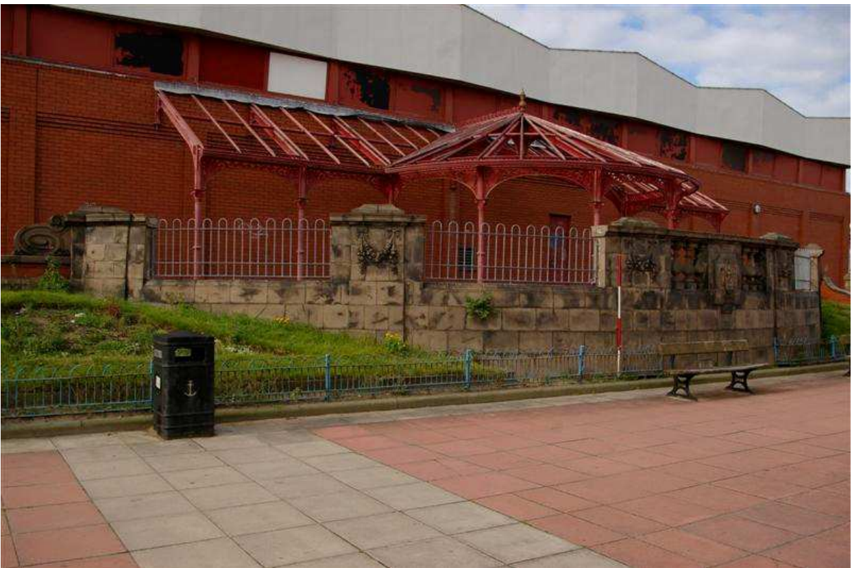
Plate 4: Terrace and cast iron canopy
