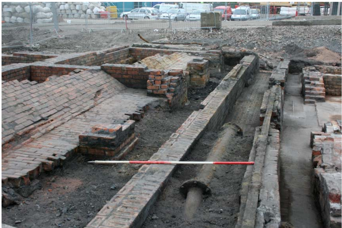
Plate 45: north-east-facing view of coal loading floor, 2436 , and water pipe chamber 2433 .
