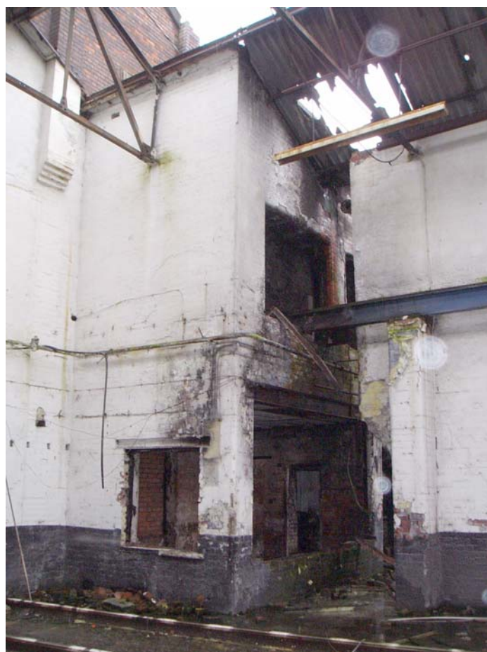
Plate 12: Building 7, and corbelled central dividing wall, Building 9
