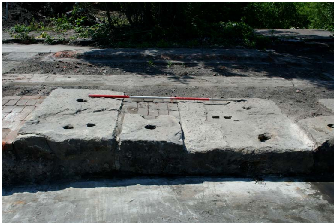
Plate 41: detail of mounting bolt settings in engine house 2429
