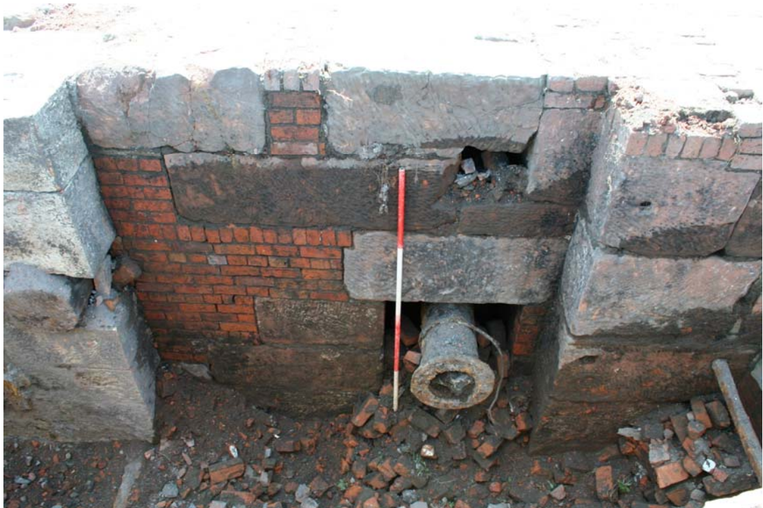
Plate 39: south-facing view of steam pipe in pump house 2404-2406
