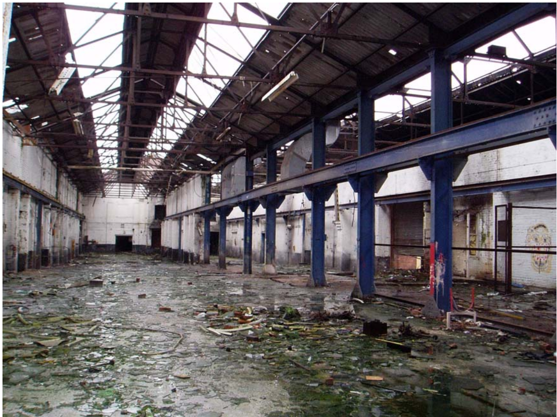
Plate 20: Interior of Buildings 9 and 12 , showing steel stanchions and brick partition
