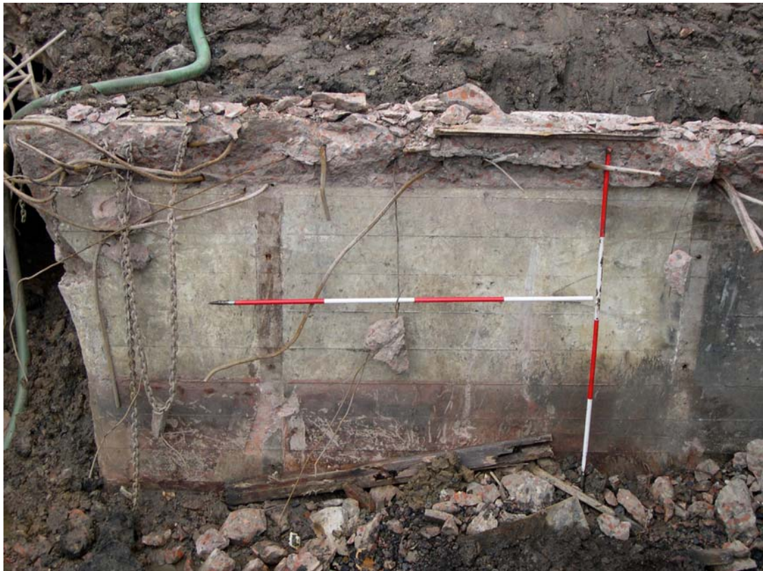
Plate 49: Exposed wall of the air raid shelter showing lines from shuttering
