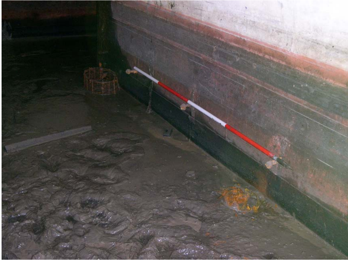
Plate 50: Bolt fastenings for a bench and internal paint finish within the air raid shelter.
