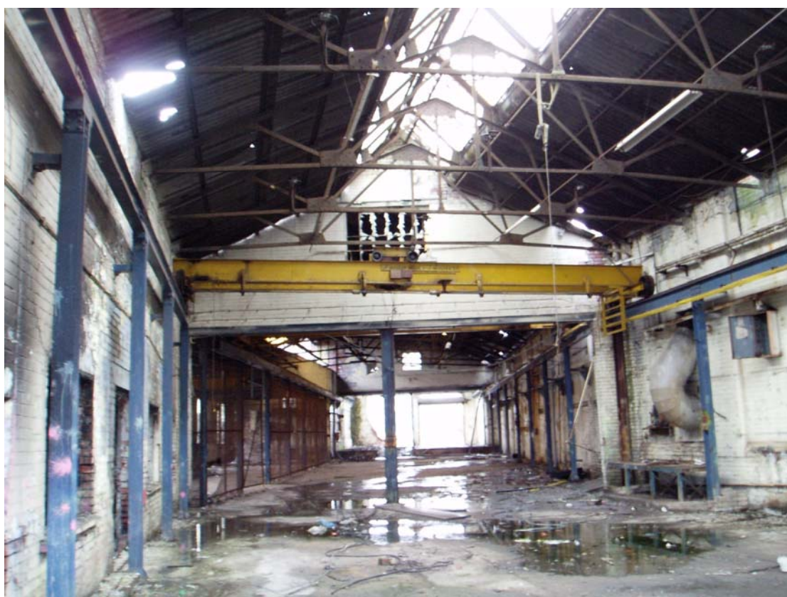
Plate 10: Lattice trusses, Building 5
