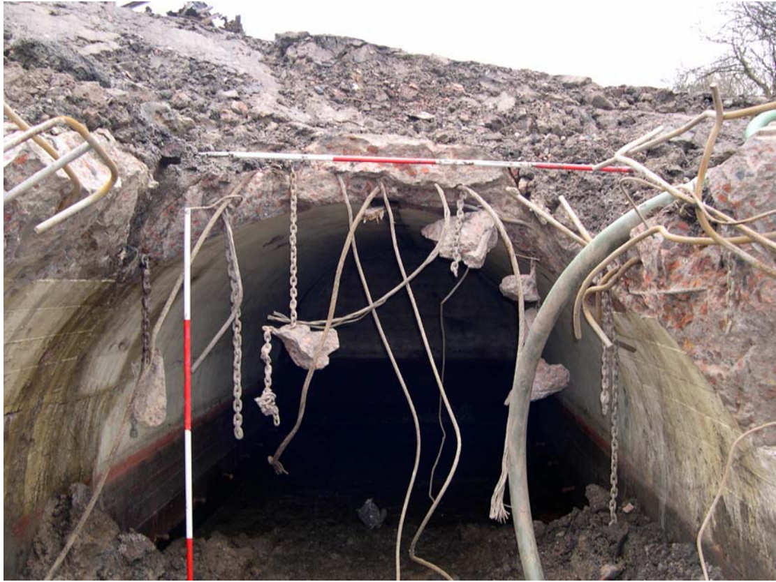
Plate 46: Section through exposed chamber of the air raid shelter showing reuse of steel ropes for strengthening
