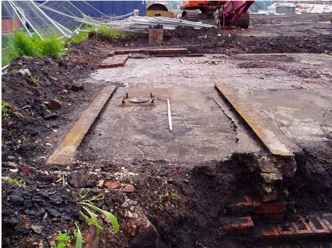
Plate 55: Metal plates and stanchion set into concrete. Coal waste was utilised as a levelling layer for the stone dust plant
