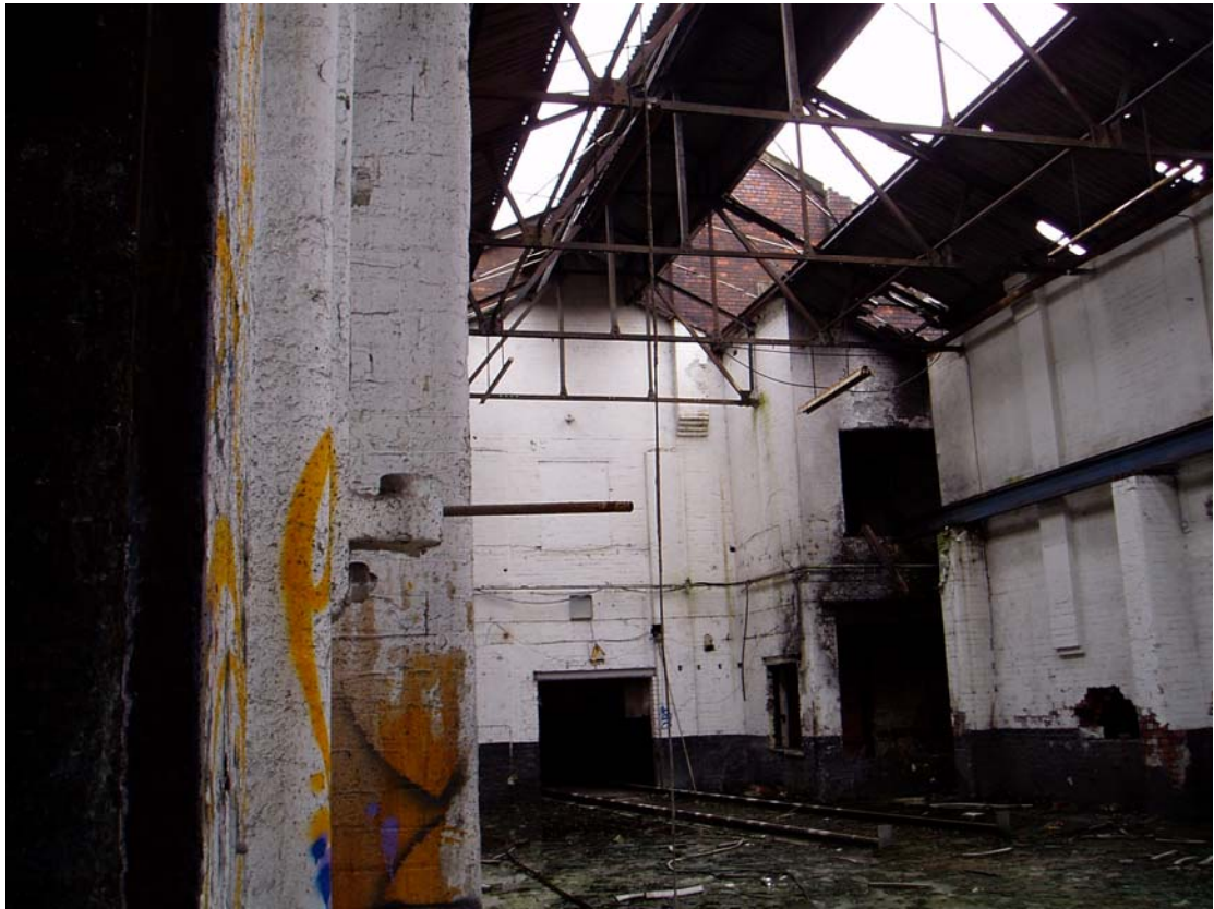
Plate 15: Interior, Building 9 , showing lattice trusses and tiered flues
