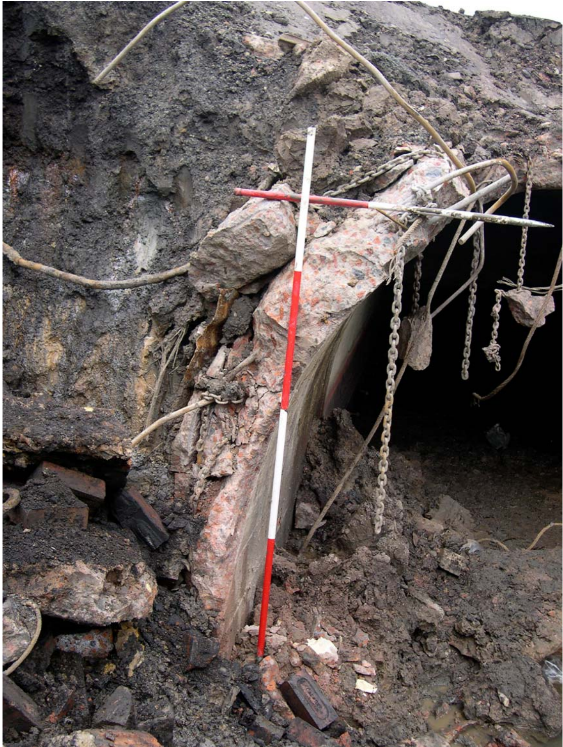
Plate 47: Construction detail of the exposed air raid shelter showing make-up of concrete
