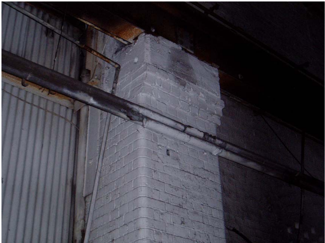
Plate 6: Corbelled buttress within Building 2
