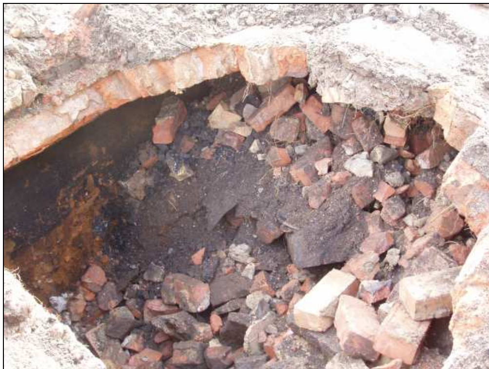
Plate 38: Vaulted cellar of Trench 5, looking south-east
