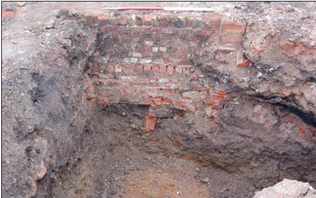
Plate 51: Excavations for Pile Cap 7, looking south-west
