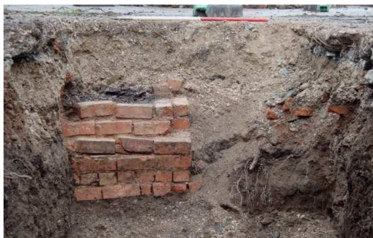
Plate 28: Wall 625 , looking north-east
