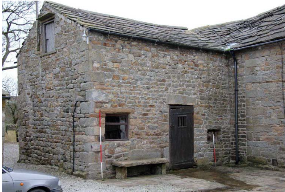
Plate 4: General view of the shippon showing north and east elevations
