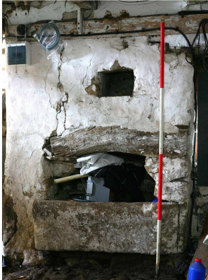
Plate 13: Drinking trough or manger in the north wall of the byre
