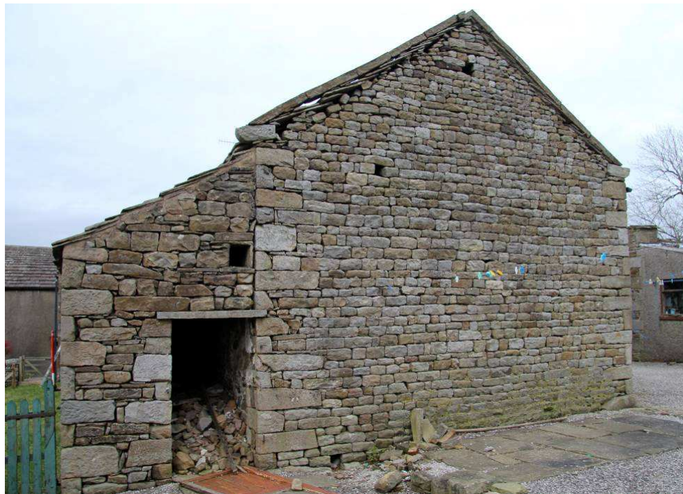
Plate 2: Oblique view of the south elevation of the barn
