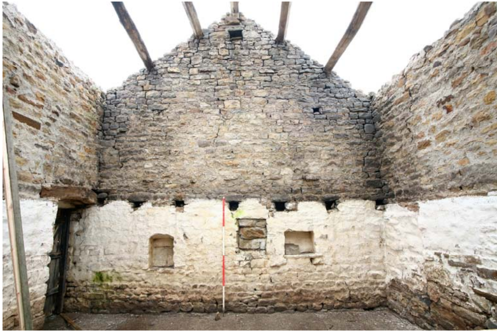
Plate 7: View of the interior of the barn facing south
