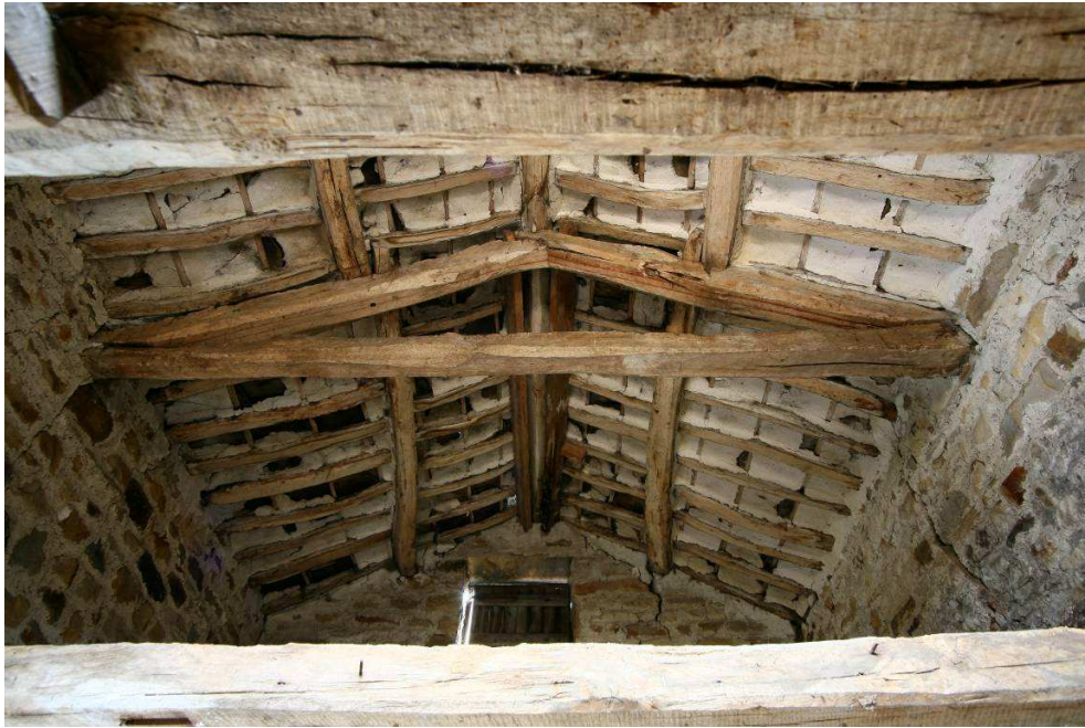
Plate 14: The roof structure in the shippon, facing east
