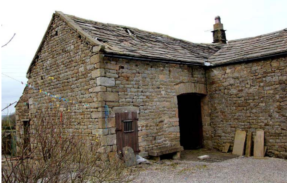
Plate 1: General view of the south side of the barn
