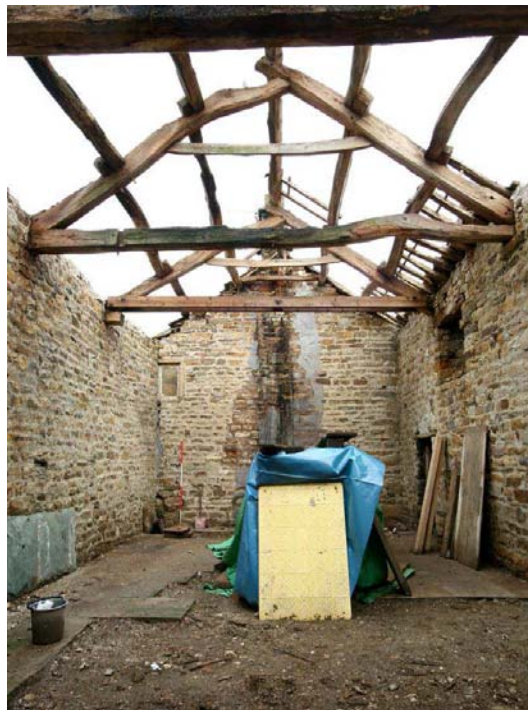
Plate 6: View of the interior of the barn facing north
