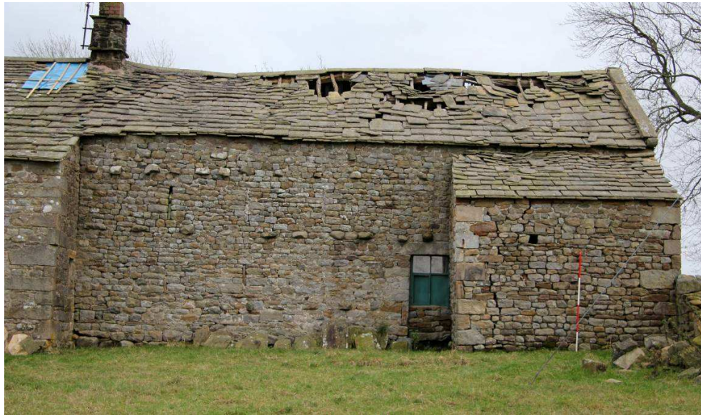
Plate 3: West elevation of the barn and lean-to
