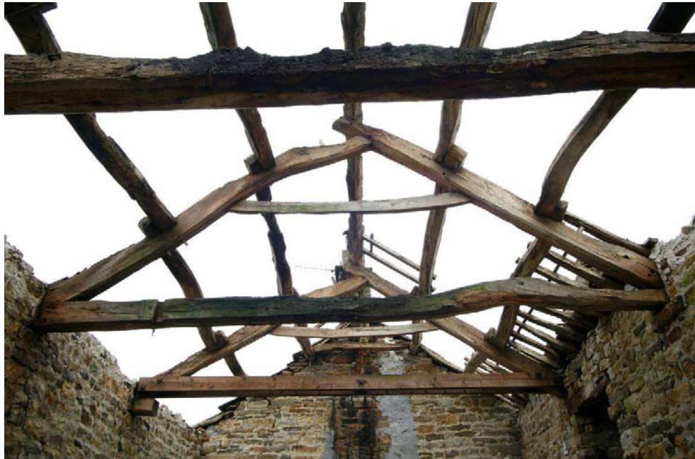
Plate 11: Truss two in the barn
