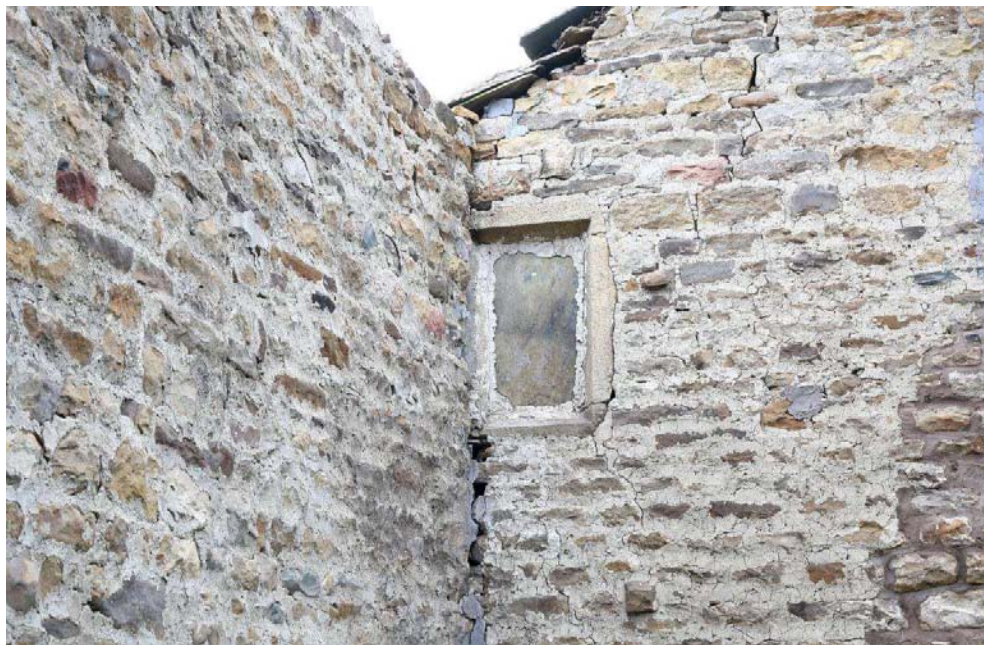
Plate 10: Bisected mullion window in the south elevation of the house
