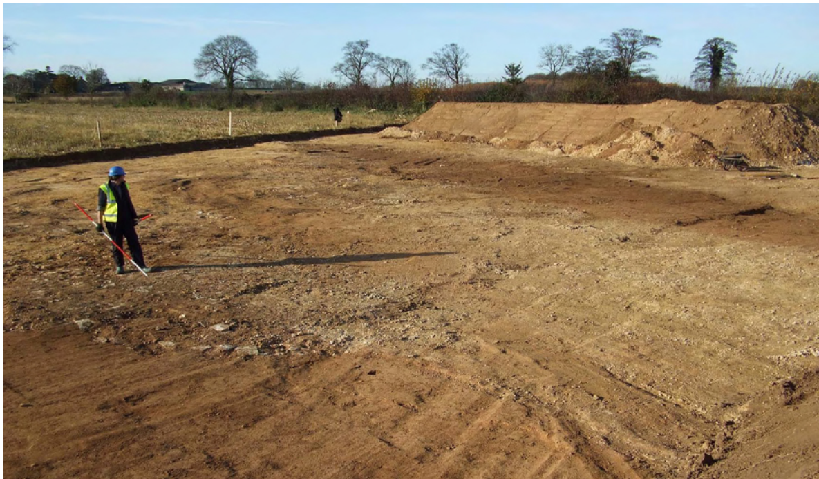
Plate 2: Site 3, showing trackway and quarry
