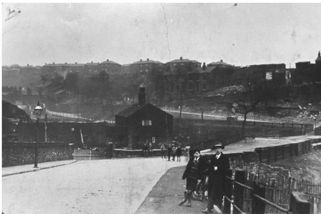
Plate 6: Demolition of houses in Bottling Wood c 1927 (270/34)
