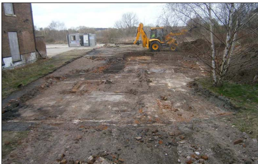
Plate 3: View looking north-west during initial mechanical stripping of the site
