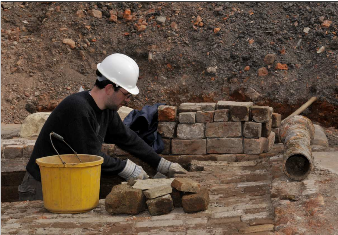
Plate 19: Volunteer excavating the remains of the Wash House
