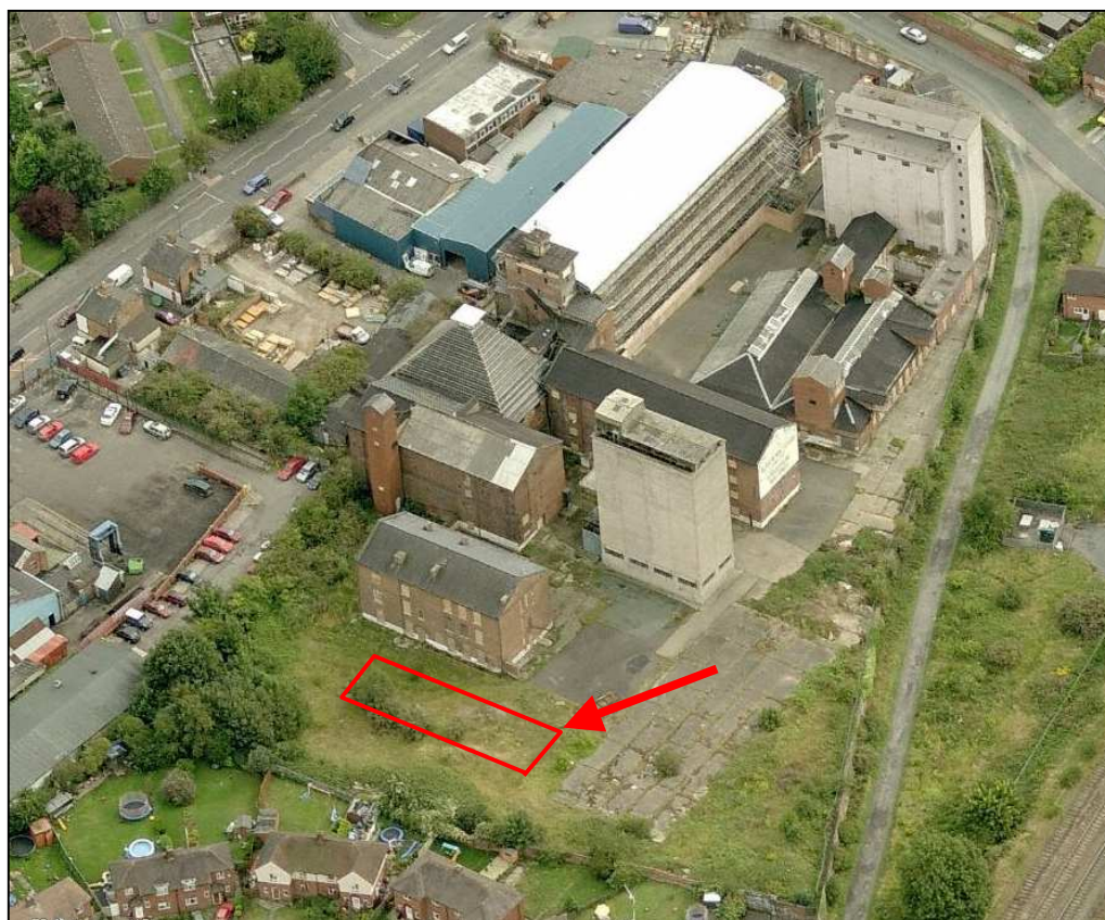
Plate 2: Arrow marking the proposed location of the excavation area, superimposed on a recent aerial view of the Ditherington Flax Mill Malting site
