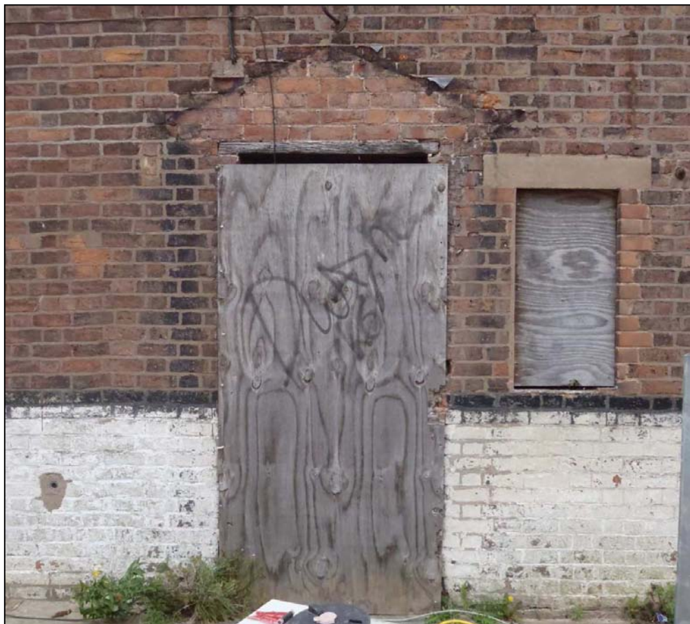
Plate 4: Wall scar 2077 visible on the north wall of the Apprentice House
