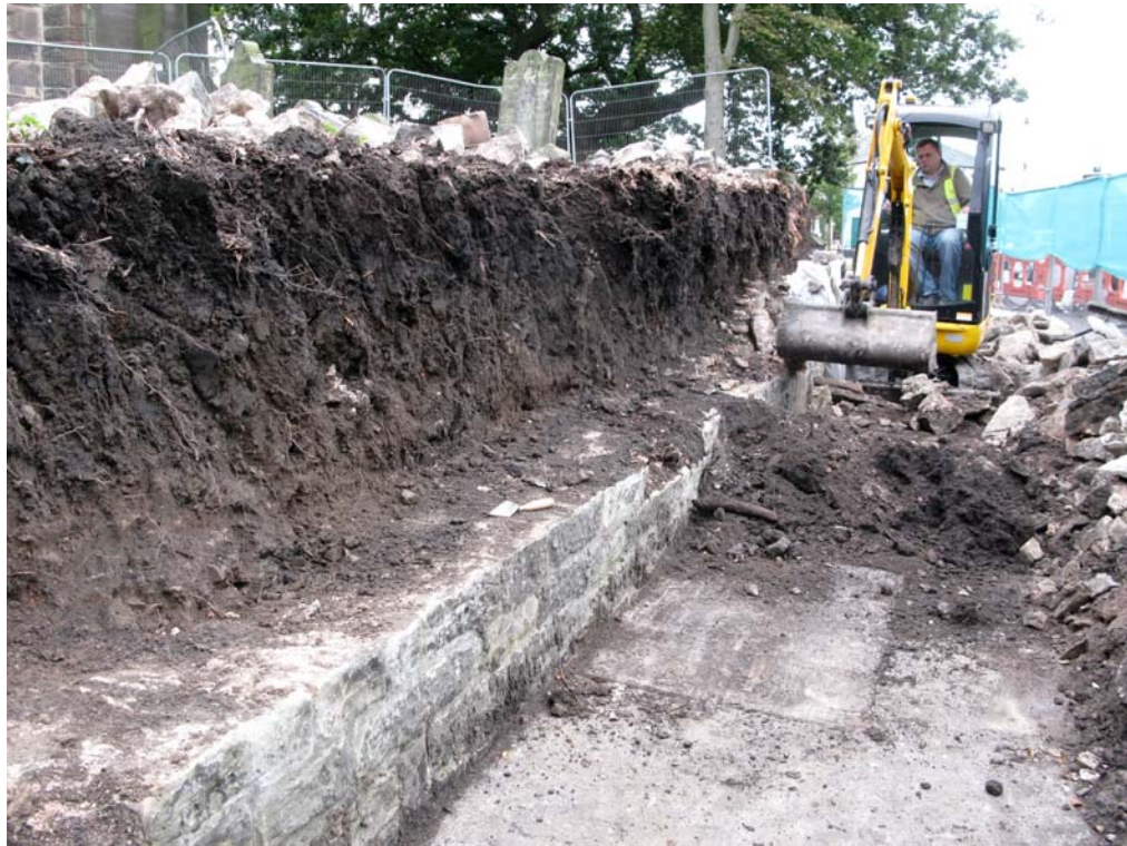
Plate 3: Excavation using a mechanical excavator
