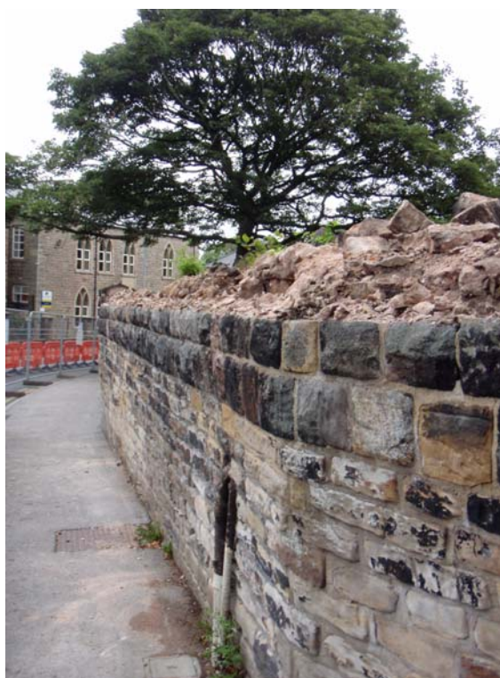
Plate 1: North-west-facing view of wall before removal for reconstruction
