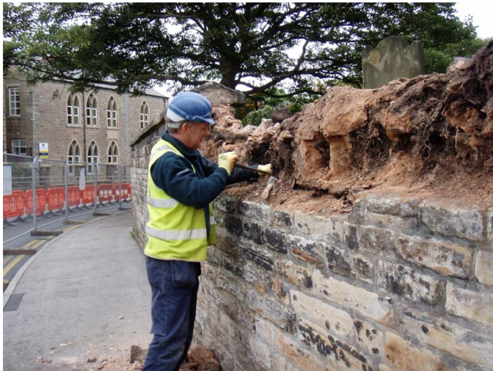
Plate 2: Careful removal of the wall manually
