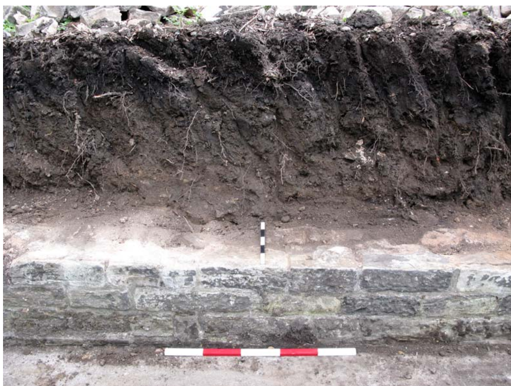
Plate 4: South-facing view of wall I and section through deposit 3
