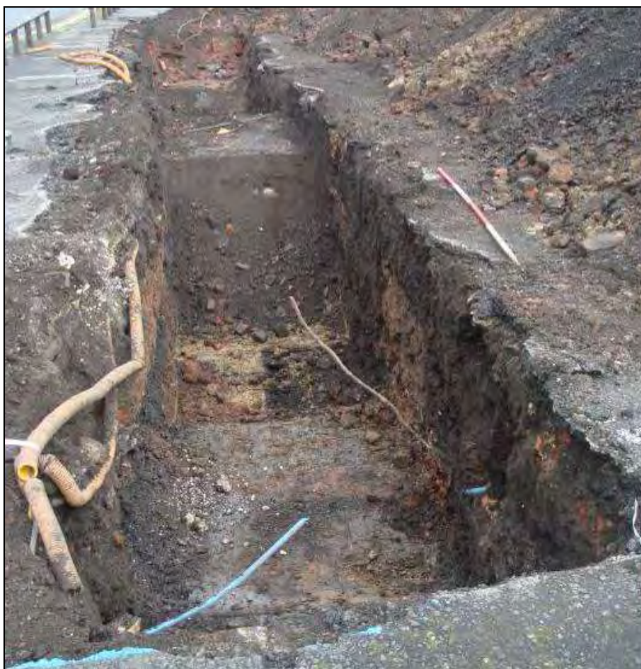
Plate 25: General view along Trench 13, looking north-east
