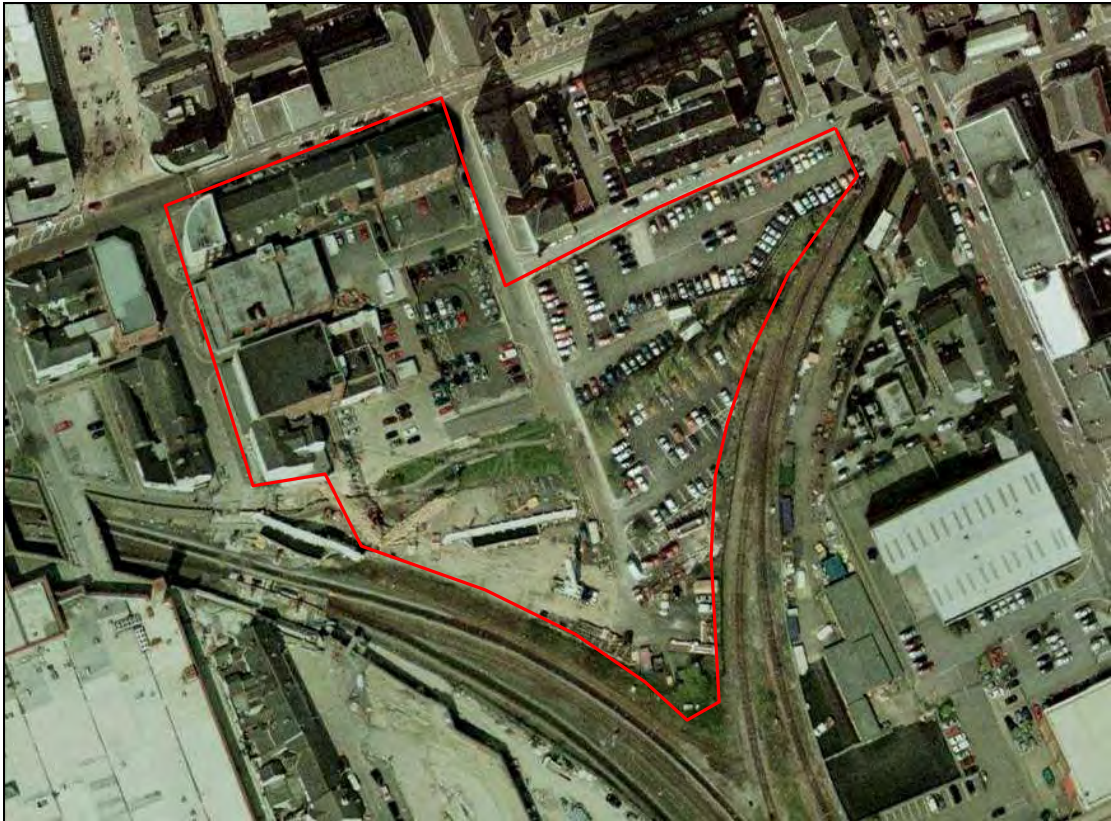
Plate 1: Recent aerial view of the study area
