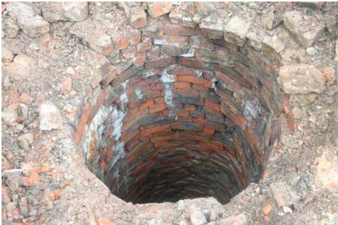
Plate 8: Brick-lined well shaft, 016 , following the removal of well cap 015
