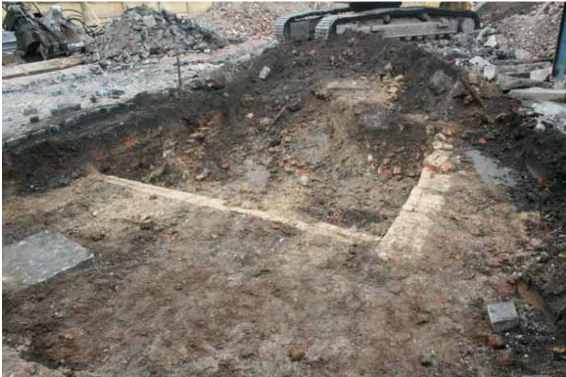
Plate 4: Area 1, south-facing shot of building foundations 006 and 008
